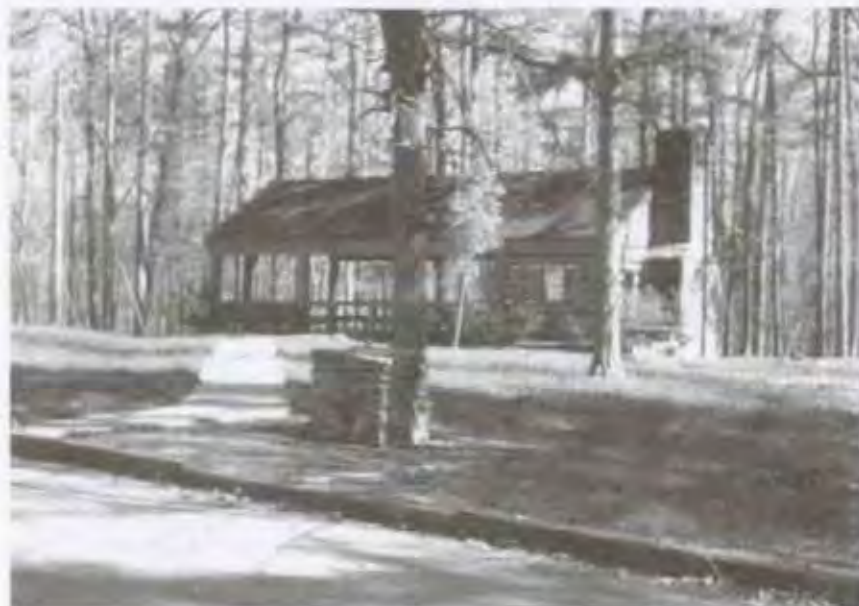
FIGURE 15. CCC Shelter in Kings Mountain State Park.
