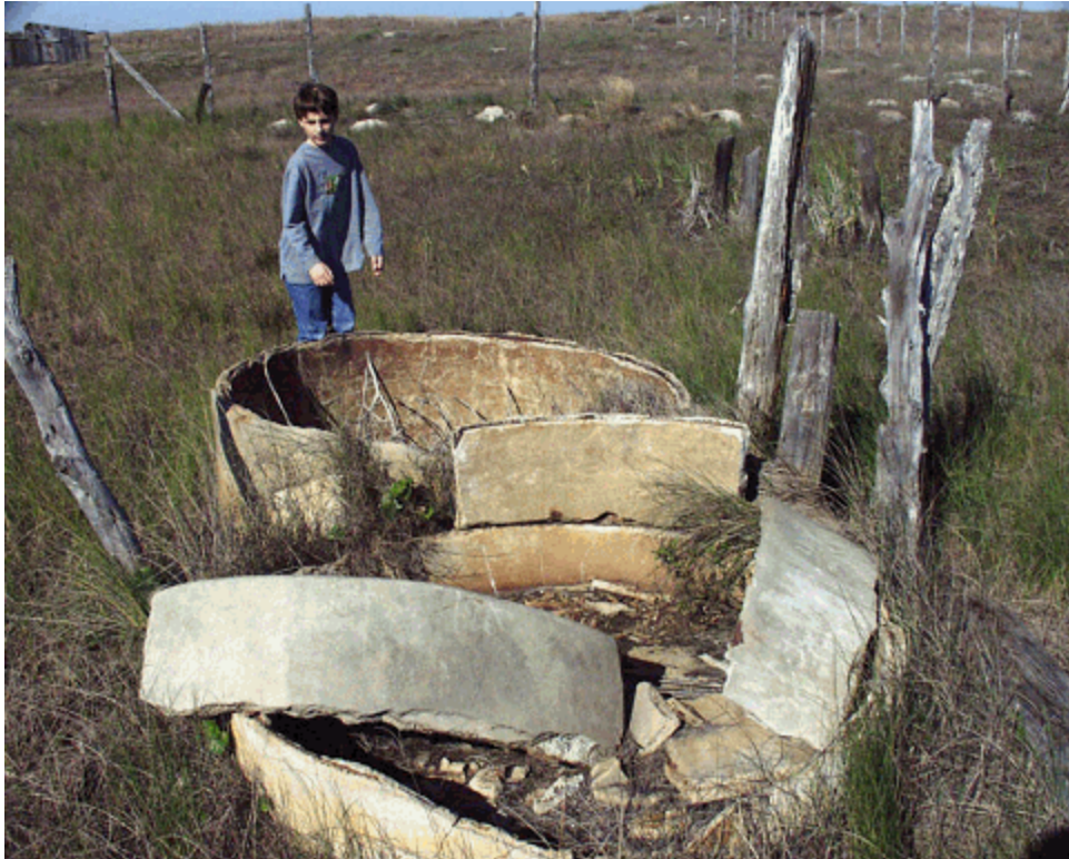
View of two concrete water tanks that held water pumped from the windmill. Photo taken February 2002.
