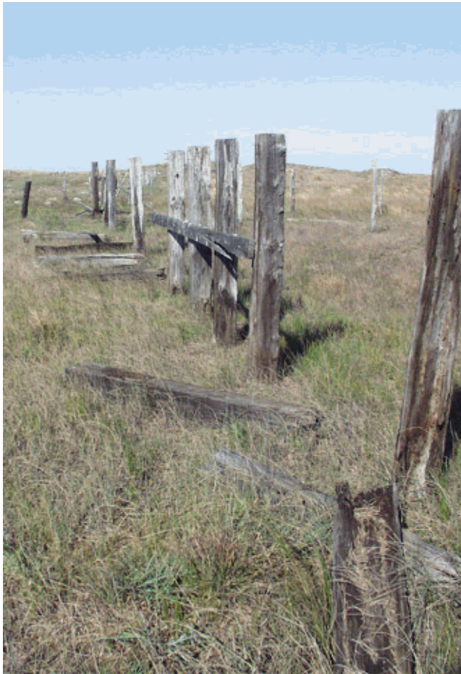
Remnants of corrals at Novillo Line Camp, looking north. Photo taken February 2002.
