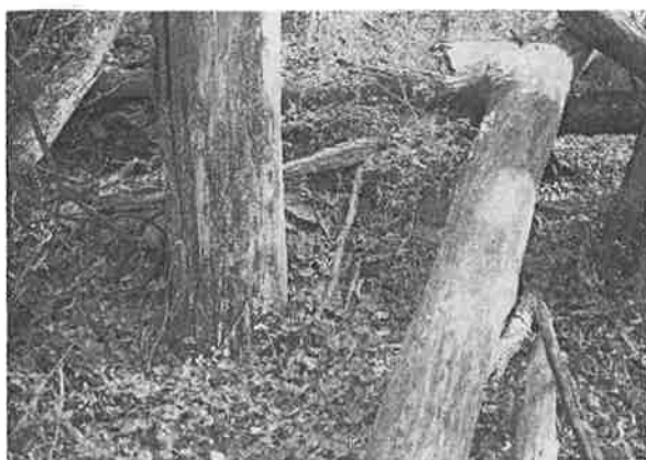
Photograph 12. Foundation of Gambrill distillery and warehouse, (JMA, 1993).
