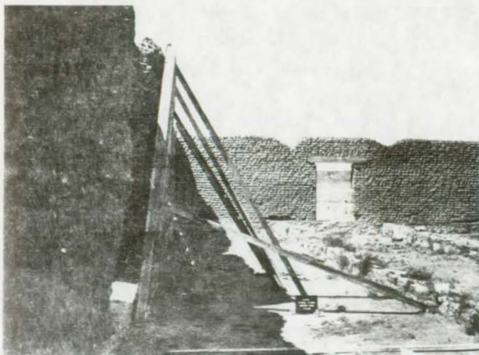
FIGURE 82. Building 3-450, Room 451, north side of south wall, before stabilization. Fort Union National Monument.
