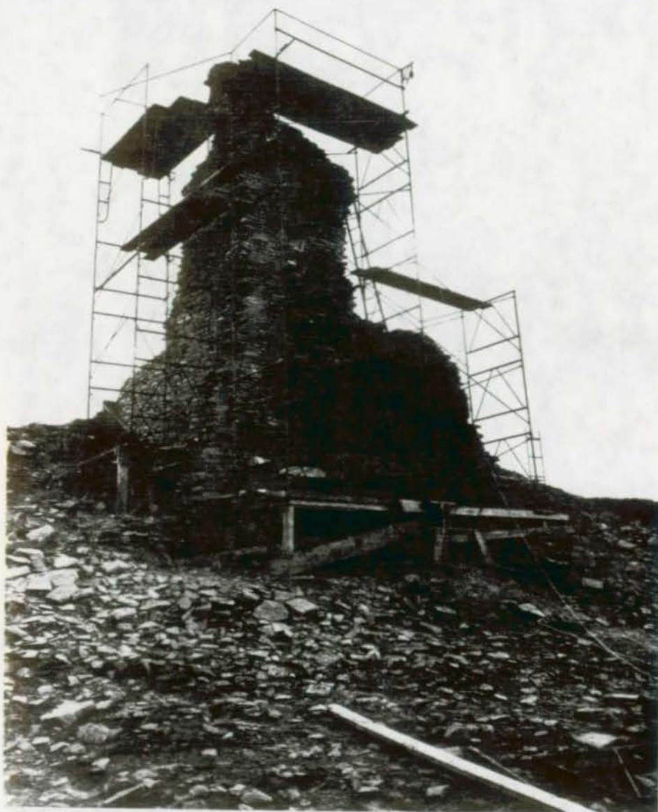
FIGURE 119. Tower Kiva. Scaffolding was anchored on firm and level bases built of heavy timbers.
