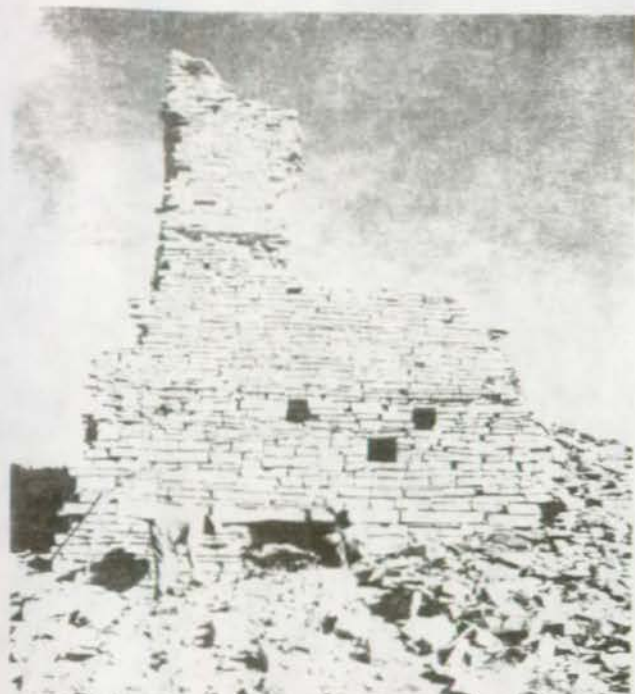
FIGURE 100. Close-up of north wall, Tower Kiva.
