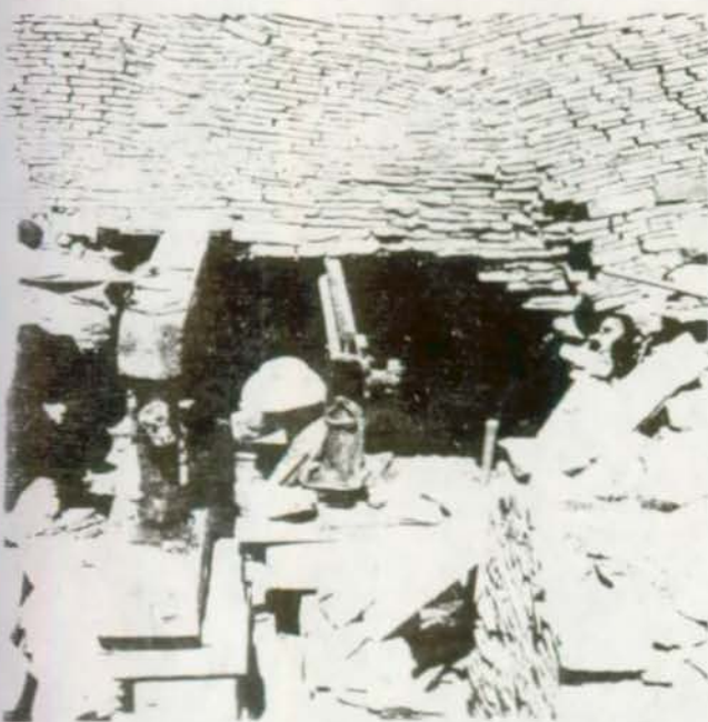
FIGURE 30. Jacks and beams provide support of wall depicted in figures 28 and 29 while arch section is removed. The break is filled with repair masonry.
