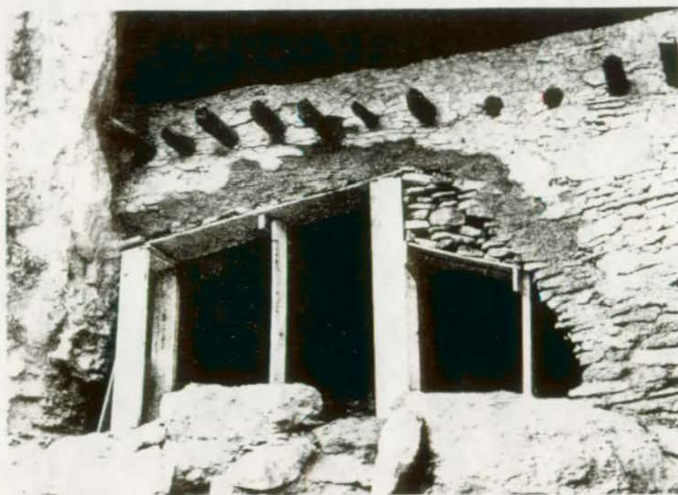
FIGURE 40. Integral member; a large reinforced arch section. The size of the break through the wall precluded filling the center with dry masonry as support, and the timber framework was substituted. The heavily reinforced band is socketed in the cliff wall at the left side, and based on bedrock at the right. The integral member has just been finished and the mortar has not yet dried. After the mortar has set the timber framework, the dry masonry at the right and that on top of the horizontal plank were removed. The large hole with its original outline remained. (Gila Cliff Dwellings National Monument, N. M.)
