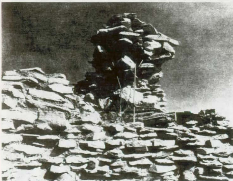
FIGURE 110. Integral members in the form of a T were installed in this top fragment of core masonry after the lower wall section had been strengthened to that point.
