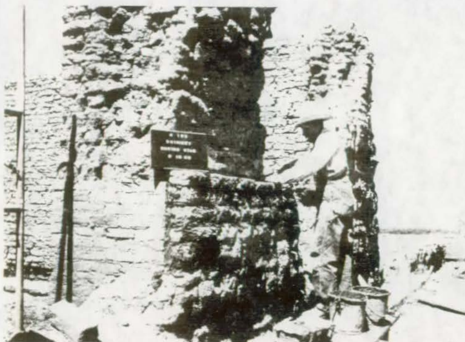
FIGURE 97. Building 6-160, Room 163, flue and chimney in east wall, during stabilization. Soil adobes are being laid to replace those that had fallen away. Fort Union National Monument.
