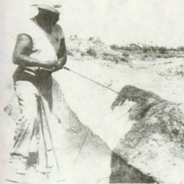
FIGURE 54. The application of a silicone water repellent. It is applied in a coarse stream, sufficient to produce a rundown of from 6 to 8 inches. (Casa Grande Ruins National Monument, Ariz.)
