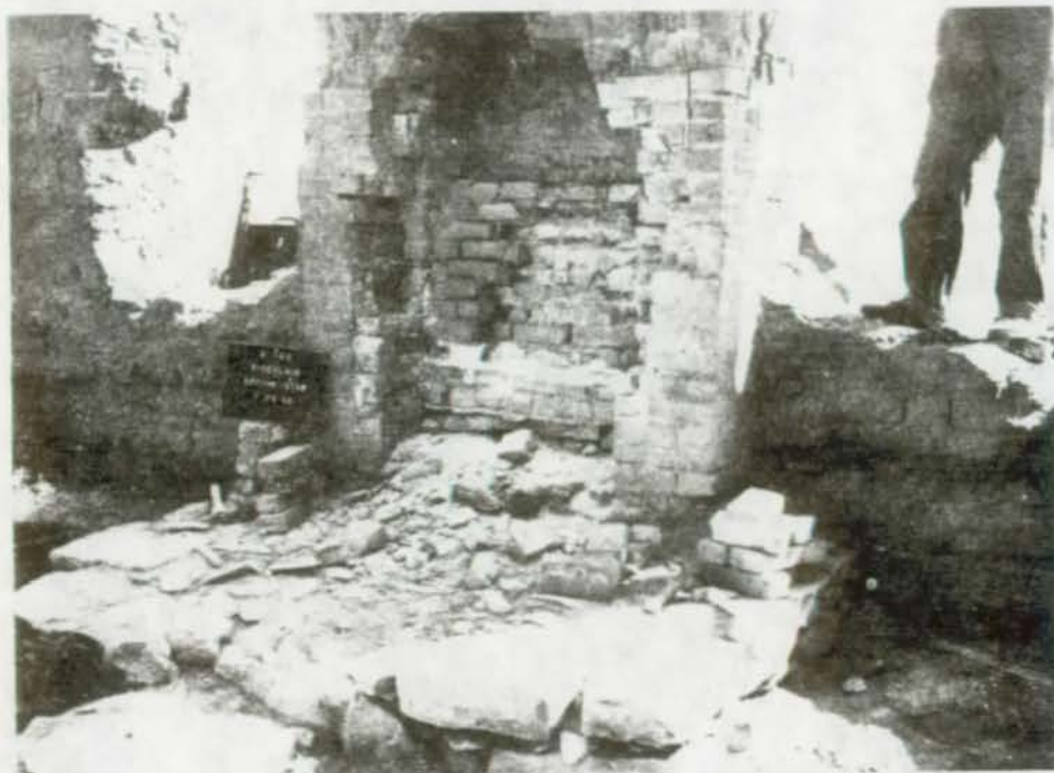
FIGURE 93. Building 6-160, Room 163, fireplace in east wall, before stabilization. Fort Union National Monument.
