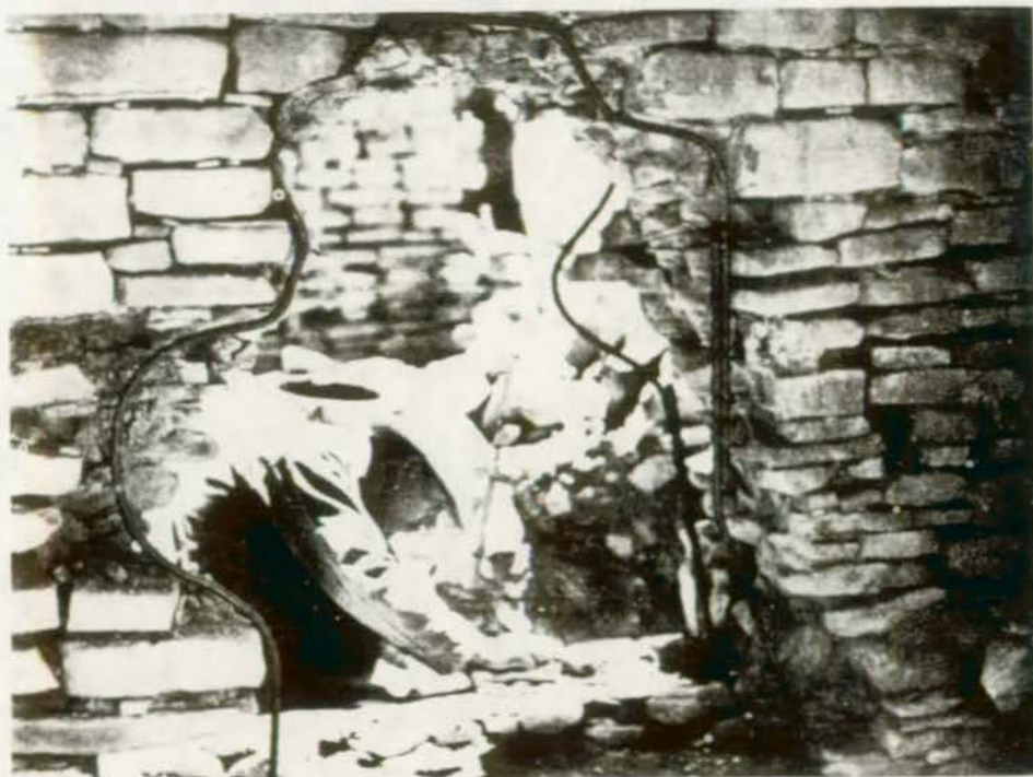
FIGURE 39. Integral members. Starting a reinforced arch section, rods have been bent to fit the contours of the break and are wired in place. The workman is laying the courses across the bottom of the break in concrete mortar to provide a solid base for the reinforced section. Above this level, masonry on the perimeter of the hole will be laid in concrete mortar which will also surround the steel rods. Masonry in the center of the hole will be laid dry or with a minimum of soil mortar; its only function will be to support masonry laid in cement until the latter has set. This dry masonry will then be removed. (Pueblo Alto, Chaco Canyon National Monument, N. M.)
