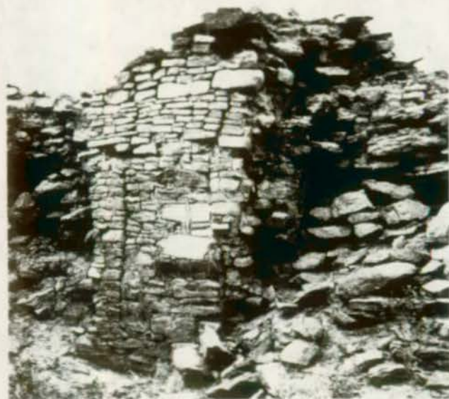
FIGURE 46. A good deal of repair masonry must be laid to fill breaks and support undercut areas in this wall at Pueblo del Arroyo. Some support must also be provided for the embedded timbers. Soil or masonry cement mortars may be used for the major part of this work. The upper courses however must be laid in concrete mortar as capping to halt further washing from the top. In this example, damage was started by surface water from adjacent, unexcavated fill and every effort should be made to prevent erosion.
