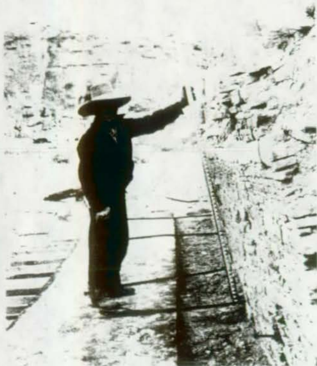
FIGURE 33. Beginning realignment. Cables have been placed through the base of the wall to be tied to the jacks. Note bolt, lower right, for holding frame against wall. (Pueblo Bonito, Chaco Canyon National Monument, N. M.)
