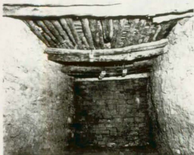
FIGURE 48. The ceiling shown in figure 47 after removal of the overburden and construction of a slab roof which protected the ceiling and permitted support of broken beams. The bolts are fastened in the slab above, and were taken up enough to transfer most of the weight from the old ceiling beams to the new roof.
