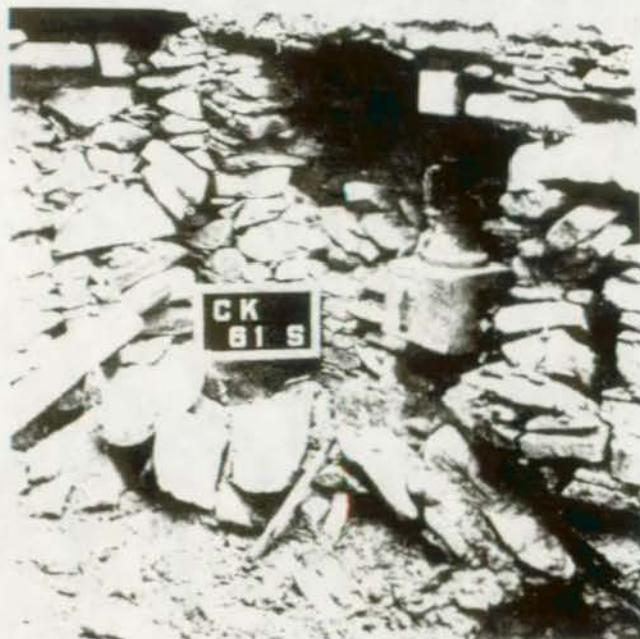
FIGURE 31. Placement of jack in line with shattered facing near the bottom of a 14-foot wall. The jack provided support while the broken area at the right was being replaced. (Chetro Kettle Ruin, Chaco Canyon National Monument, N. M.)
