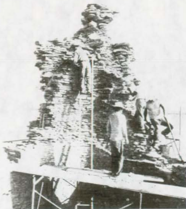
FIGURE 107. Tower Kiva, interior northeast corner, during installation of integral members to strengthen the highest wall section.
