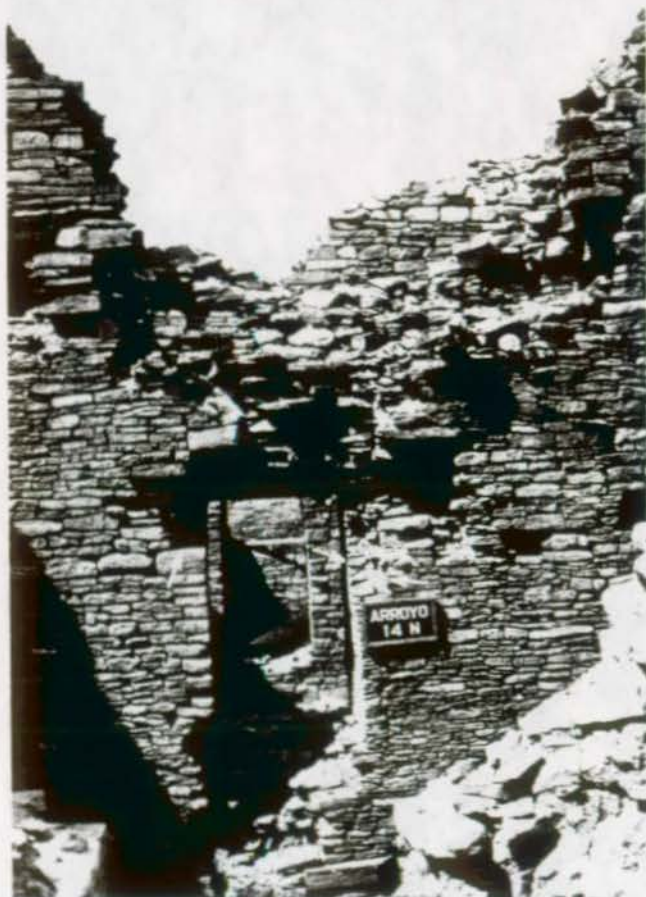
FIGURE 25. Repair at the position of the arrows will be based on a very small area in comparison with the total size of break. Every effort should be made to tie such patches securely to the existing wall. (Pueblo del Arroyo Ruin, Room 14, north wall, Chaco Canyon National Monument, N. M.)
