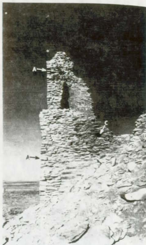
FIGURE 116. North wall stub capped (arrows A), lower portion of west wall facing reset (B), and exposed portion of thick core grouted (C).
