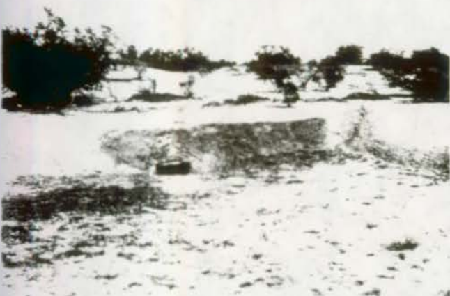
FIGURE 13. West wall of Compound A immediately after a rain. The light areas treated with silicone repelled water. The darker areas were untreated and absorbed moisture rapidly. (Casa Grande Ruins National Monument, Ariz.)
