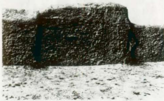
FIGURE 14. West wall of Compound A one year after the application of silicone waterproofing. Two hairline cracks were filled. The untreated smears of plaster have absorbed moisture, while the treated wall remains dry. (Casa Grande Ruins National Monument, Ariz.)
