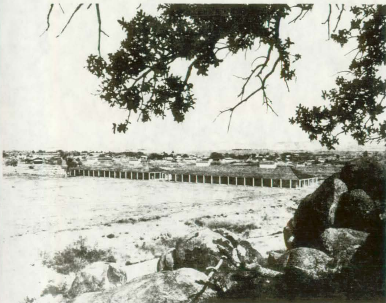
FIGURE 61. A view of the Fort Davis barracks after restoration. The ruinous shell seen in figure 60 was veneered with hand molded soil cement bricks, 4" x 4" x 12". They were made with one part portland cement (untinted), three parts unwashed sand, and three parts native soil. The bricks laid in masonry mortar with rough joints, set with spalls, were wire-brushed. Original walls were pared down where required to accommodate the veneer brick and to retain original wall dimensions and thickness. Bond beams were installed at roof line to support the restored, hipped, shingled roof. The soil cement brick walls were painted with white cement paint, although originally they were whitewashed. The building is used functionally today as the Visitor Center. Cost of the restoration: $129,000 or $12.90 per square foot.
