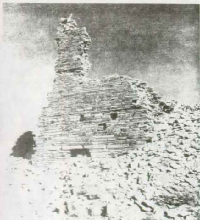
FIGURE 101. Tower Kiva, north wall exterior. Note large hole at base, and eroded insets (arrows) where second, third and fourth stories were slightly stepped back.
