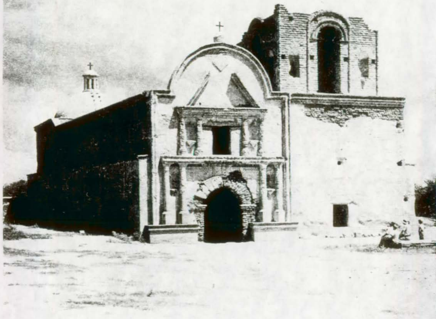
The Mission Church, Tumacacori National Monument, Tumacacori, Arizona. Comprehensive stabilization, repair, and partial restoration of the Mission Church was performed in 1921 by Frank Pinkley. Lower portions of the columns and bases of the facade were restored in 1945. Since that time, all efforts by the National Park Service have been directed to preserving existing original construction. Replacement plaster, where required to cover eroded original lime plaster and adobe brick surfaces, consists of a tinted cement-lime-sand mortar employed with a bonding agent.
