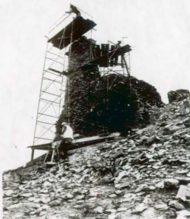
FIGURE 42. Reinforced integral members are important in the stabilization of spirelike structures such as this at the Tower Kiva, Kin Ya-a Ruin, Chaco Canyon National Monument, N. M. Considerable strength must be added without serious or objectionable alterations of the original profile.
