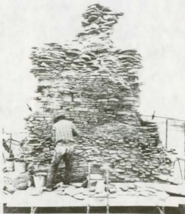
FIGURE 109. Beginning the vertical, reinforcement capping (arrows).
