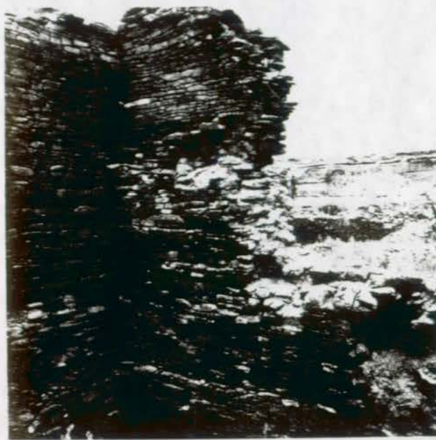
FIGURE 45. Patching of this hole at Pueblo del Arroyo will be combined with a short section of horizontal capping plus vertical capping for the exposed and weathered vertical rise of wall.
