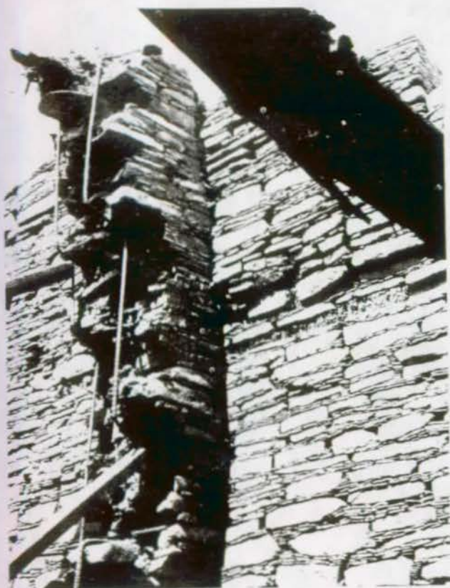
FIGURE 41. Integral members; steel in place for a narrow vertical section. The steel must be tied in securely to the cross wall at the top to provide support for the overhanging area. Some support will be required for the vertical strip of masonry as it is being laid, and until the concrete mortar has set. (Chetro Kettle Ruin, Chaco Canyon National Monument.)
