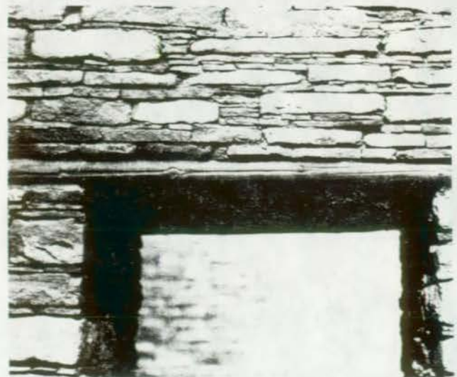
FIGURE 37. The cast concrete lintels have the same appearance as the originals from which they were cast. (Chetro Kettle Ruin, Chaco Canyon National Monument, N. M.)
