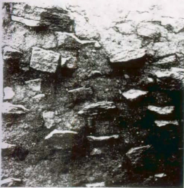
FIGURE 8. The use of heavy grouting to replace native soil between random stone; after 10 years exposure to the elements. (West Ruin, Aztec Ruins National Monument, N. M.)
