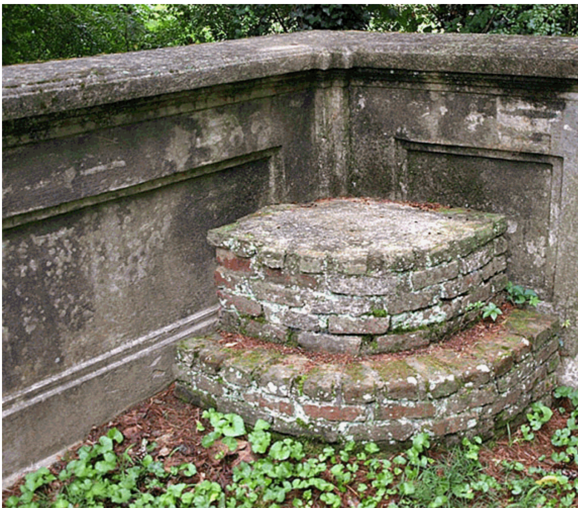
Figure 41. Unidentified brick feature at the southeast corner of the cemetery in 2010. Source: NPS SERO
