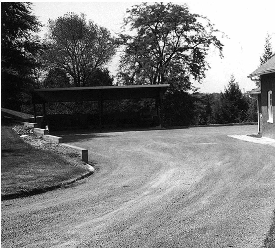
Figure 14. The utility area undergoing expansion (c.1958-1961). Source: ANJO Photo Collections
