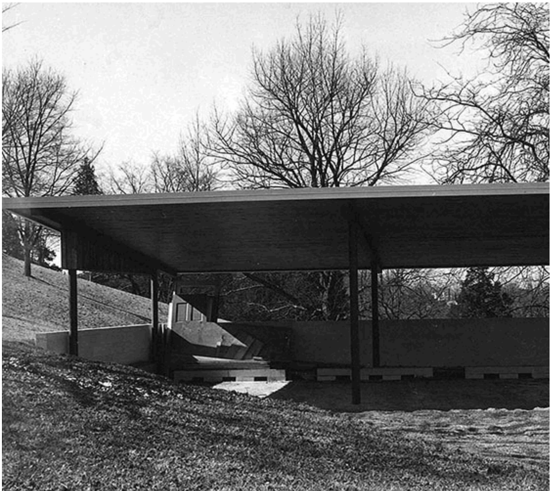
Figure 13. Maintenance shed near completion in 1957. Source: ANJO Archives
