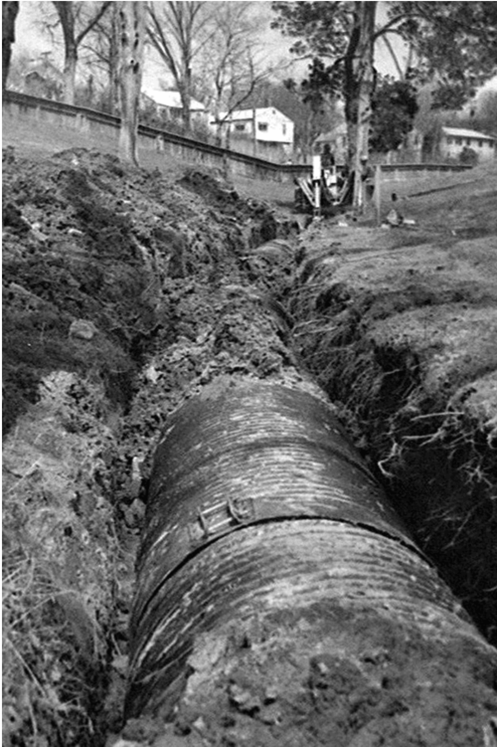
Figure 19. A drainage culvert during installation in 1975, replacing an open-drainage flume near the western edge of the property. Source: ANJO Photo Collections
