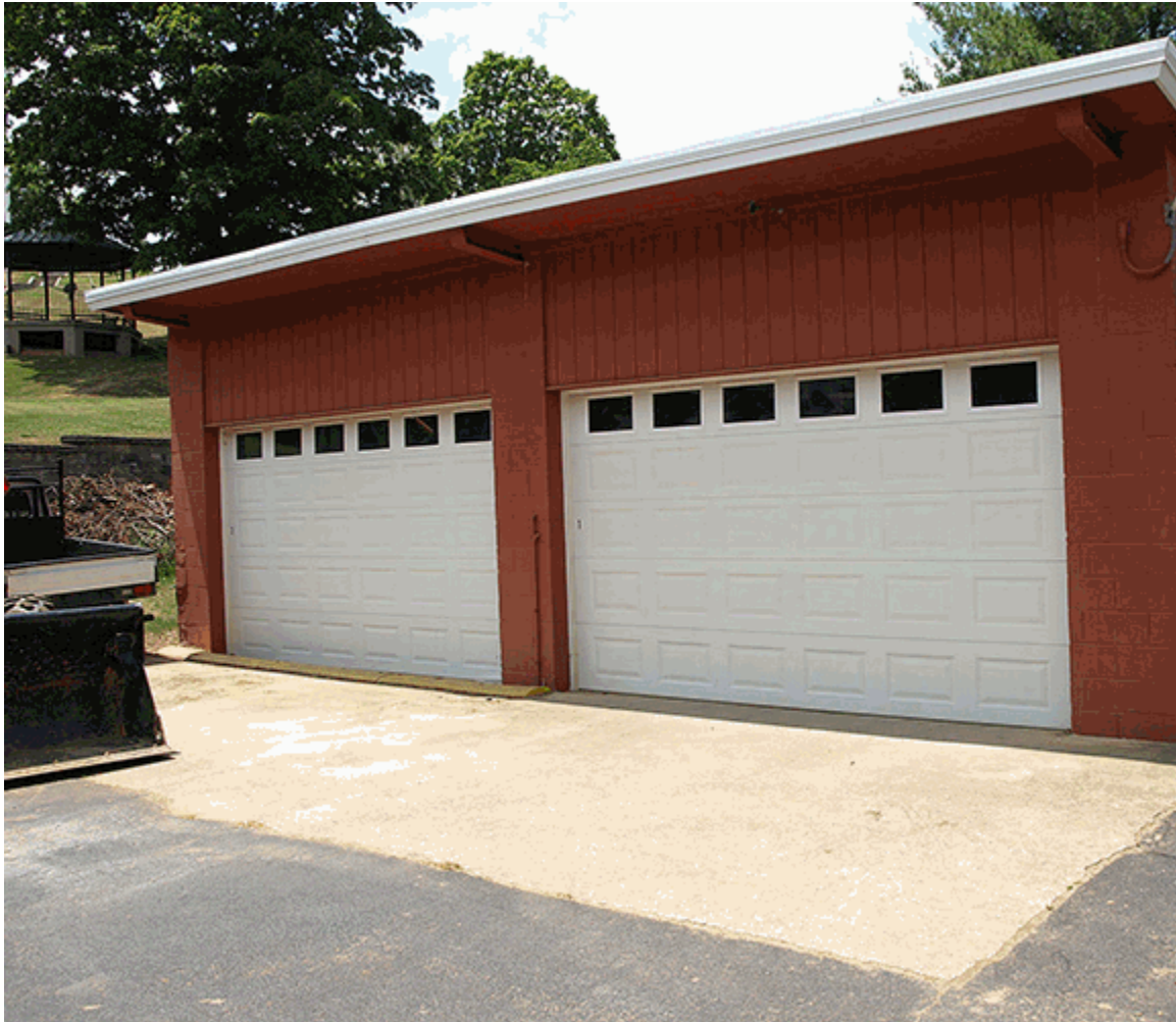
Figure 34. The maintenance shed in 2010. Source: NPS SERO
