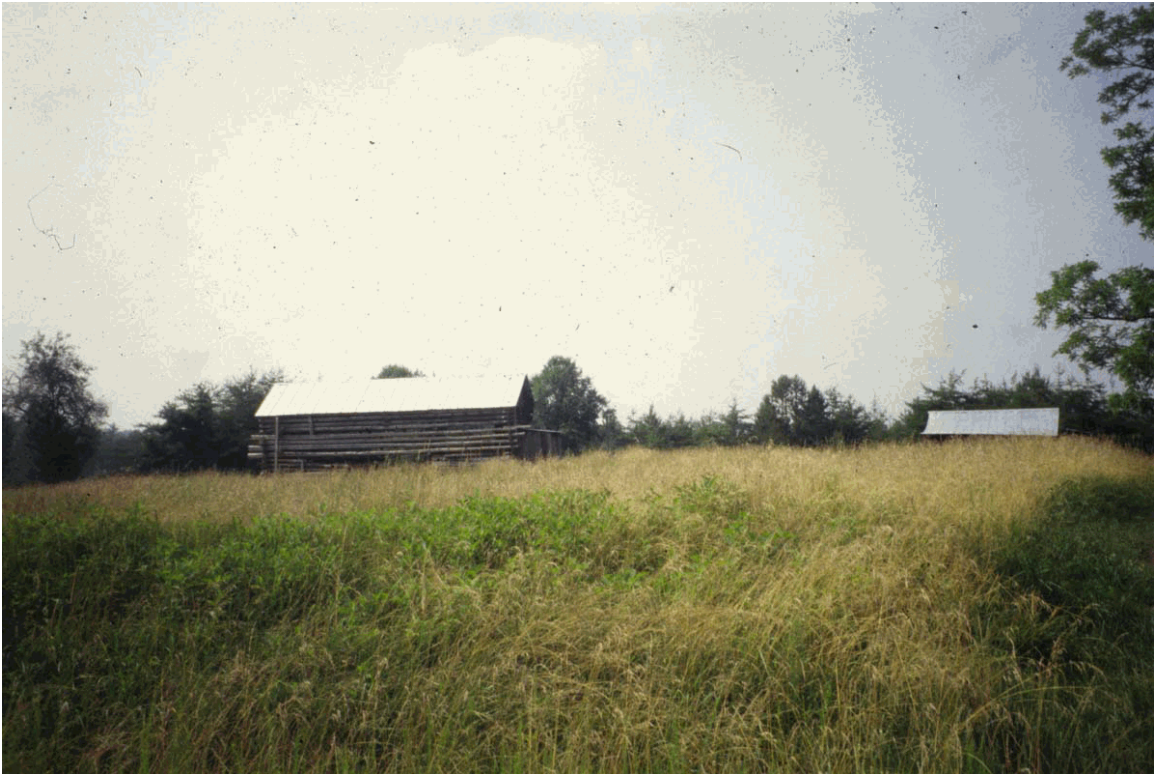
Lora Blevins log barn, with log corncrib to right and open field in foreground
