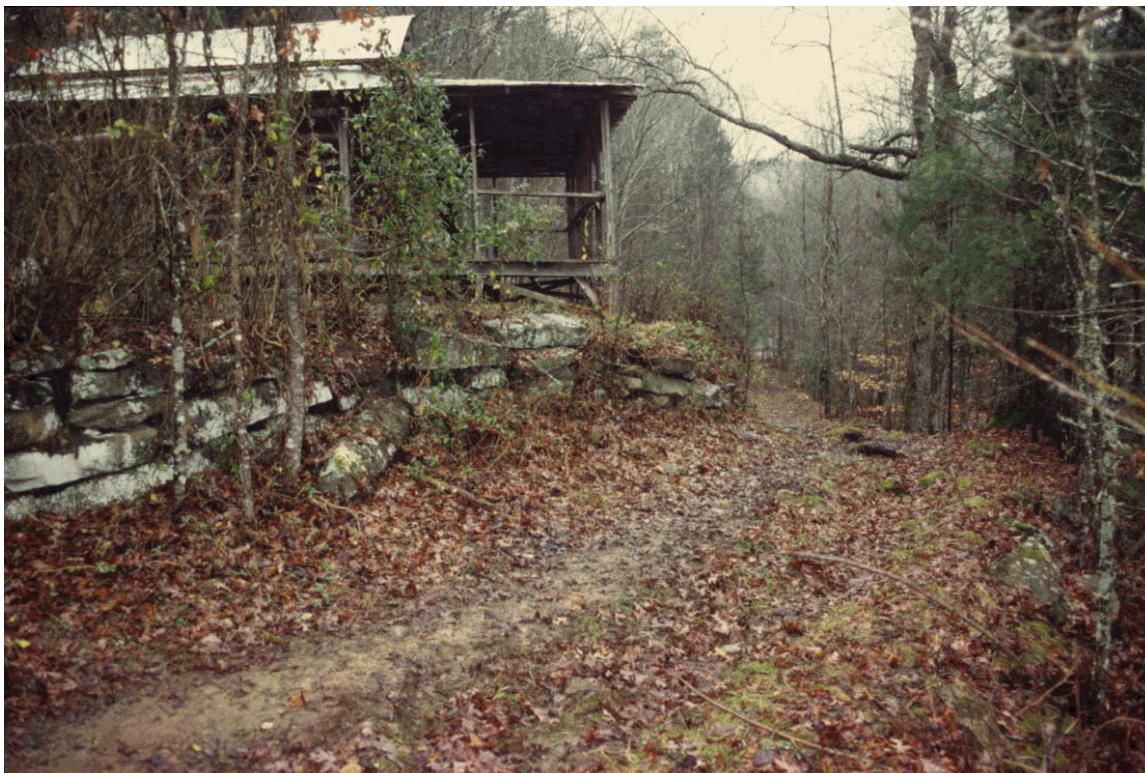
Stone retaining wall along trail in front of cabin (non-extant)
