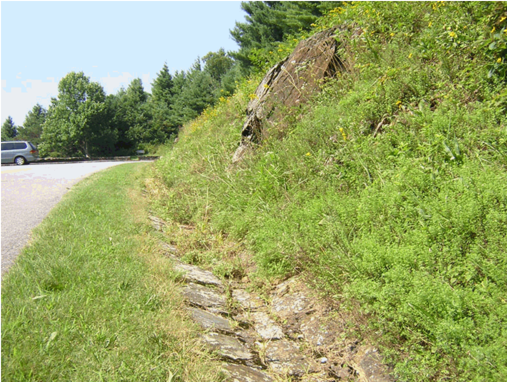
Stone gutter on west edge of parking lot (2005).
