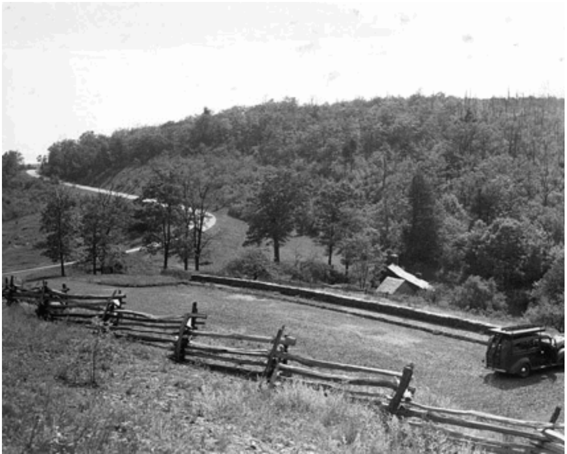
Brinegar Cabin Parking Area (1946)
