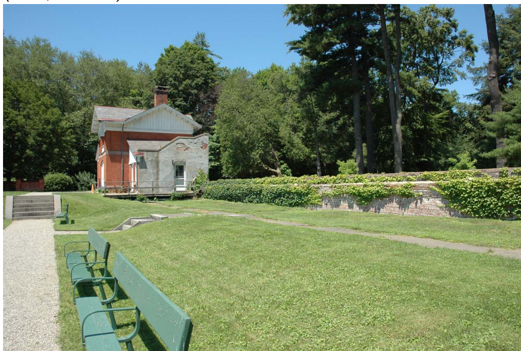
Figure 25. View northeast of the Tool House and site of the former Carnation House. Three steps that formerly led into the center of the Carnation House are visible on the left (OCLP, June 2008).
