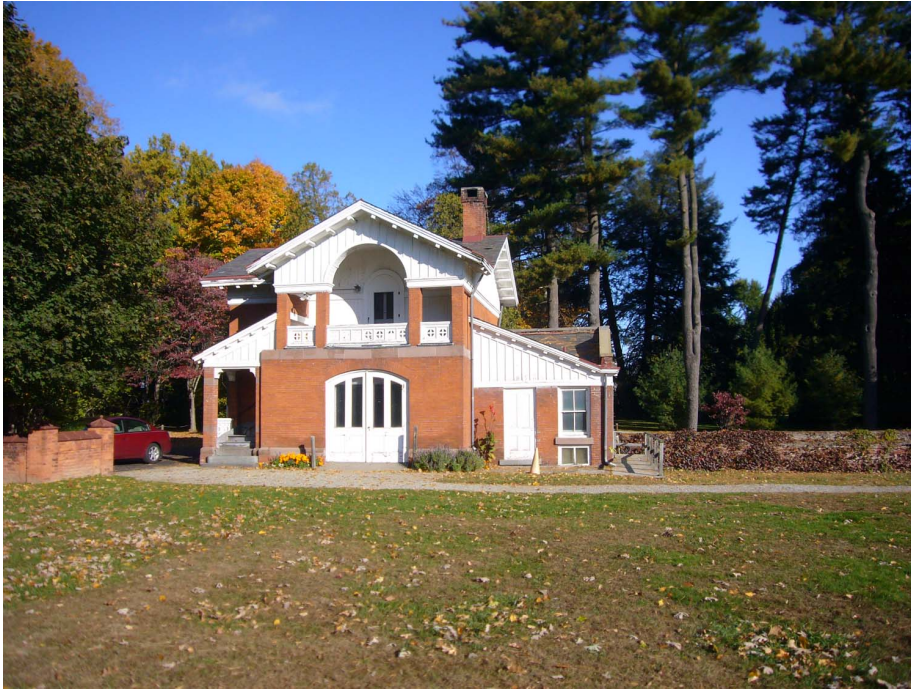
Figure 16. View north of the Tool House, constructed in circa 1875, which is now used by the Frederick W. Vanderbilt Garden Association as its meeting and office space (OCLP, October 2008).
