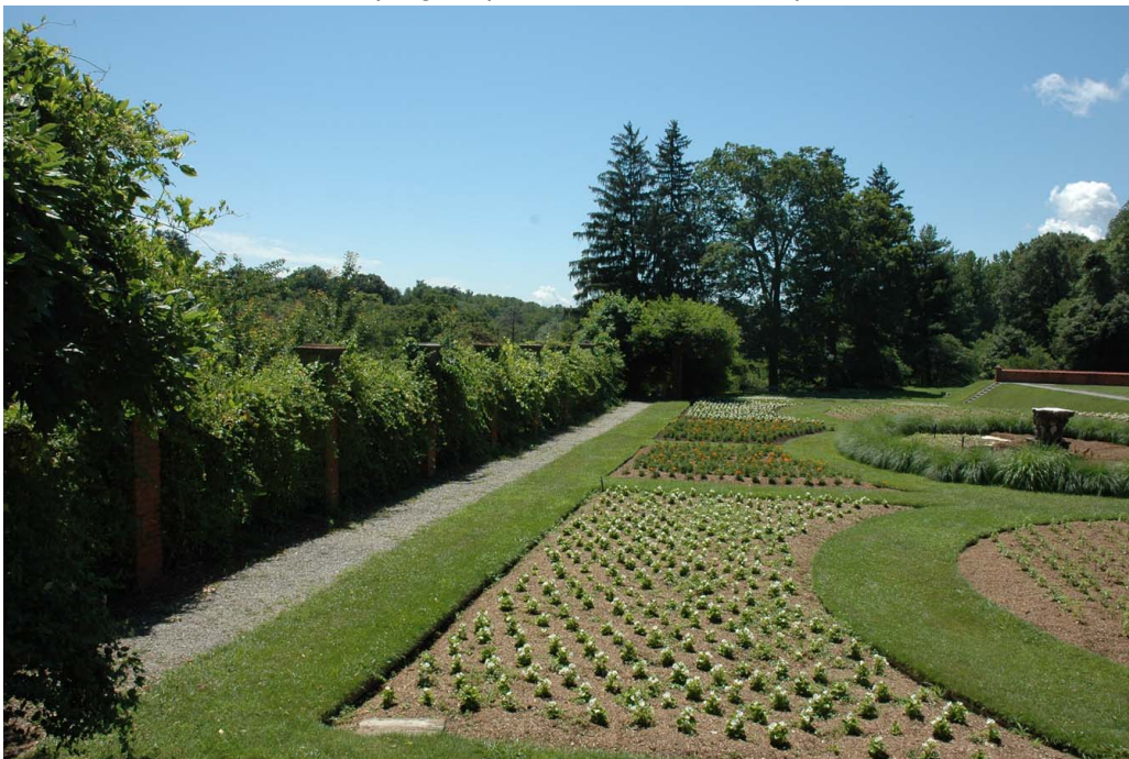
Figure 27. View south of the upper annual terrace edged by a pea stone walkway and trellis structure. The trellis consists of brick piers with limestone capitals that support a wire lattice and vines (OCLP, June 2008).
