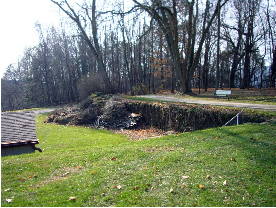
Figure 22. View looking northwest showing the mortared stone retaining wall along the former cutting garden (OCLP, October 2009).
