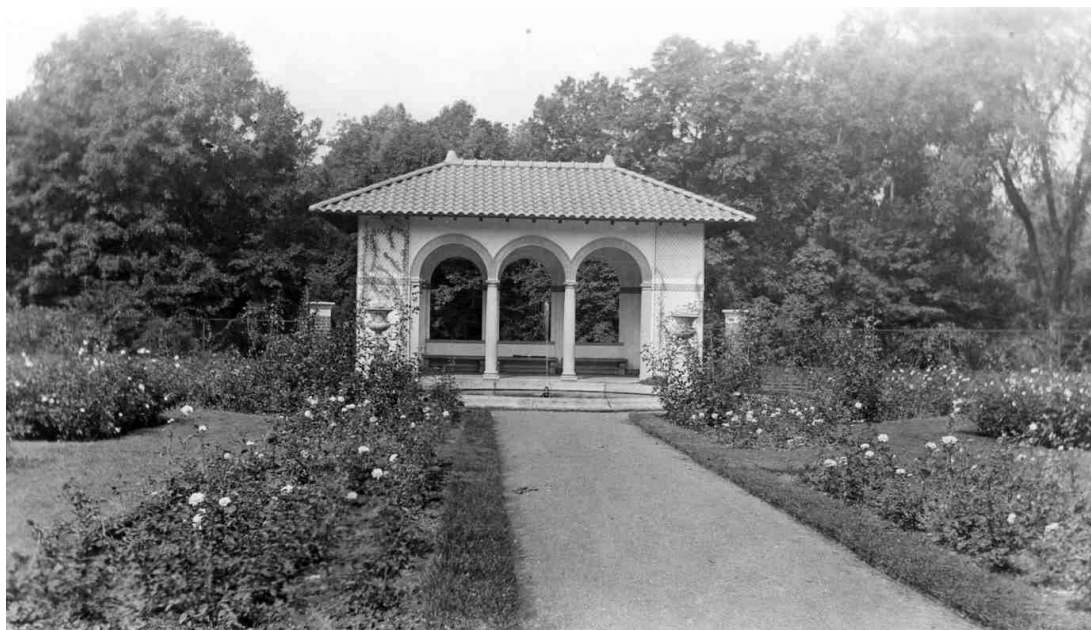
Figure 13. View looking east showing the rose garden loggia flanked by ornamental vases with the frog fountain at center, circa 1922. Shrubs planted outside the perimeter fence are barely visible (VAMA, no. V-41, Alex Knauss Collection).
