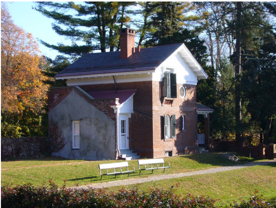
Figure 17. View northeast of the Gardener's cottage, constructed in circa 1875, which now serves as a park staff residence (OCLP, October 2008).
