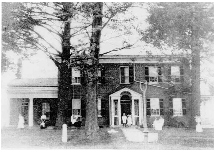
Figure 5. A 1903 photograph of the south side of the Hunt House. (Seneca Falls Historical Society)
