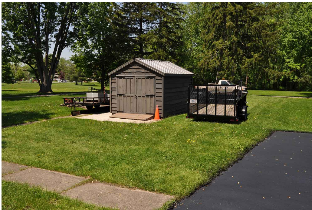
Figure 24. View of the remnant pool deck of the filled swimming pool, and the storage shed. (View northwest, OCLP 2018, DSC-065)
