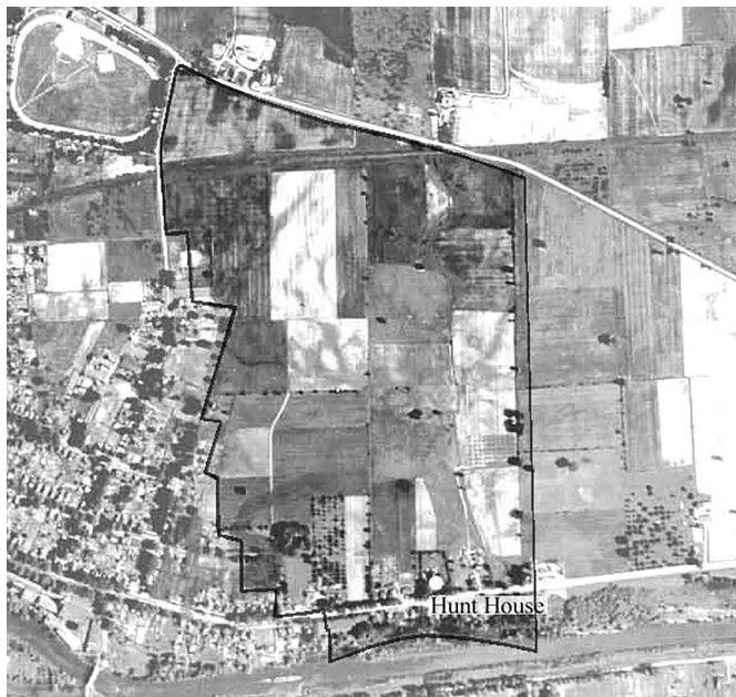
Figure 6. An 1938 aerial photograph showing the Hunt Farm and several structures north of the Hunt House. The approximate location of original Hunt property is outlined. (Bird Library Map Collection)
