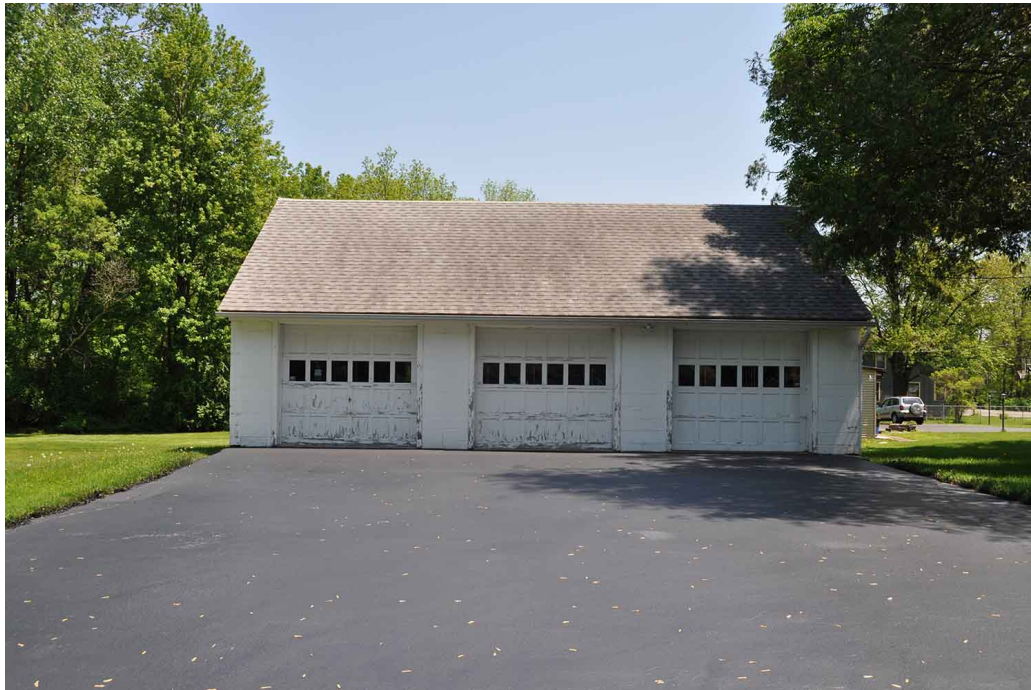
Figure 23. West side of the garage, constructed in 1954. (View east, OCLP 2018, DSC-064)
