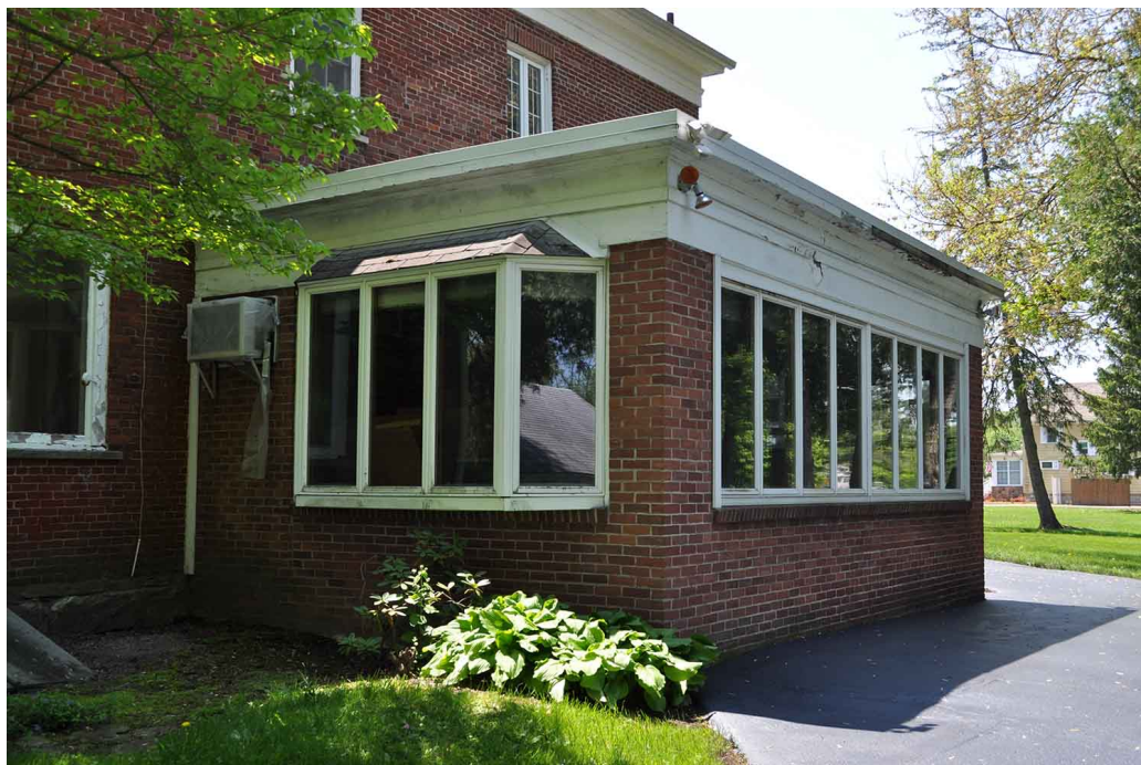
Figure 21. View of the 1960 addition to the north (rear) of the house. (View southwest, OCLP 2018, DSC-061)
