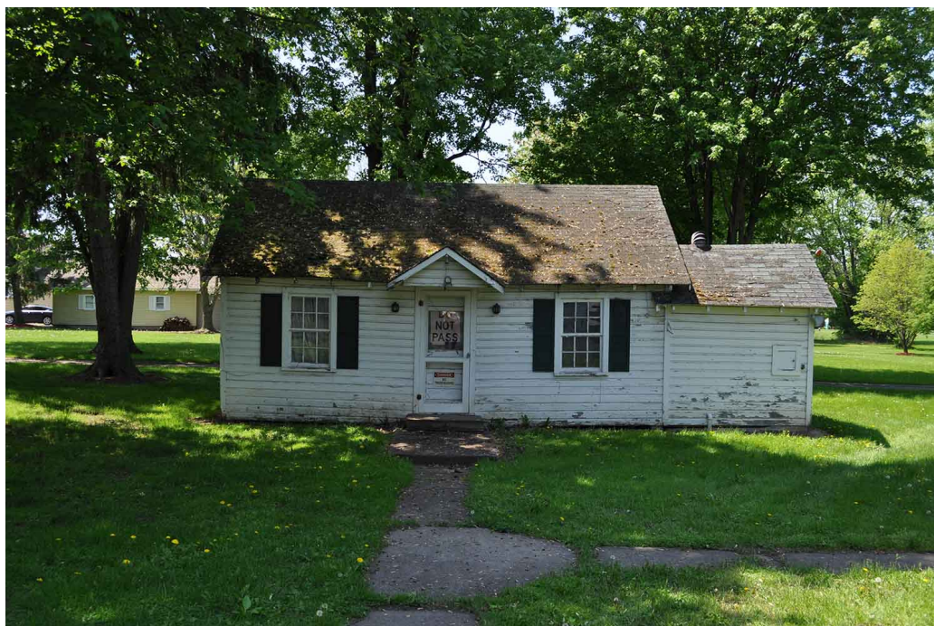
Figure 22. East side of the cottage/pool house. (View west, OCLP 2018, DSC-063)
