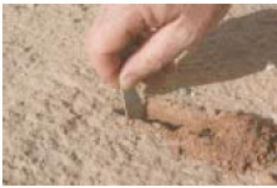
Figure 8-3. Excavate small trench
