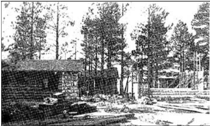
Illustration 16. Construction of Deluxe Cabins, North Rim, 1927. ( Nebraska State Historical Society )
