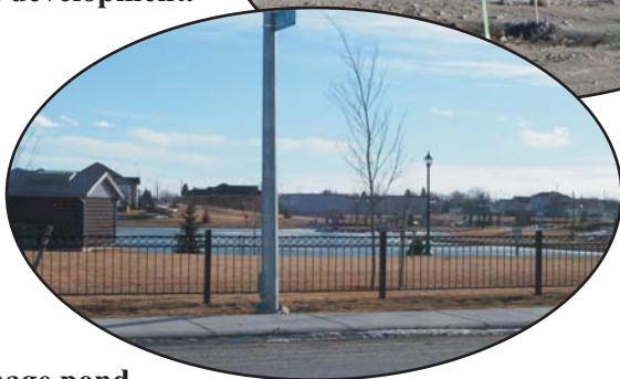
Gravity drainage pond.
