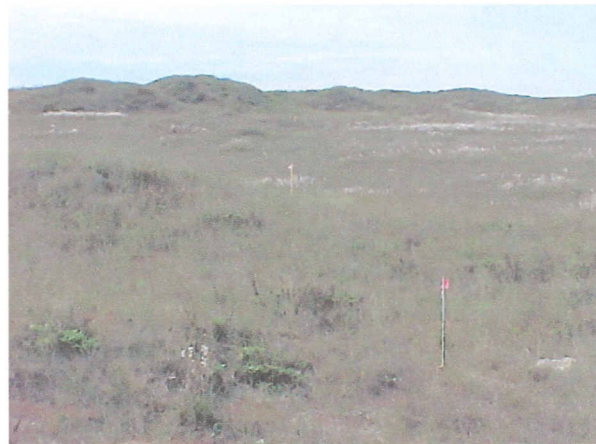
L/LS stakes marking pipeline route
