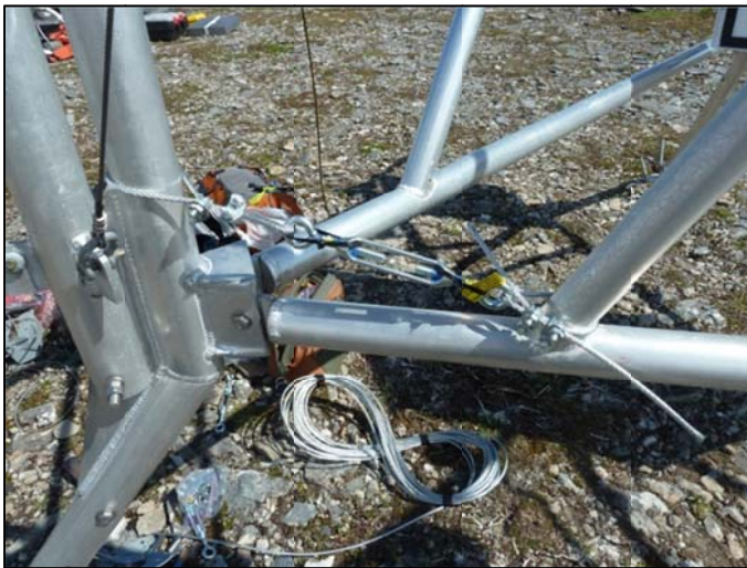
Figure 15. Fourpeaked RAWS – Field repair of broken weld in tri-leg tower frame.
