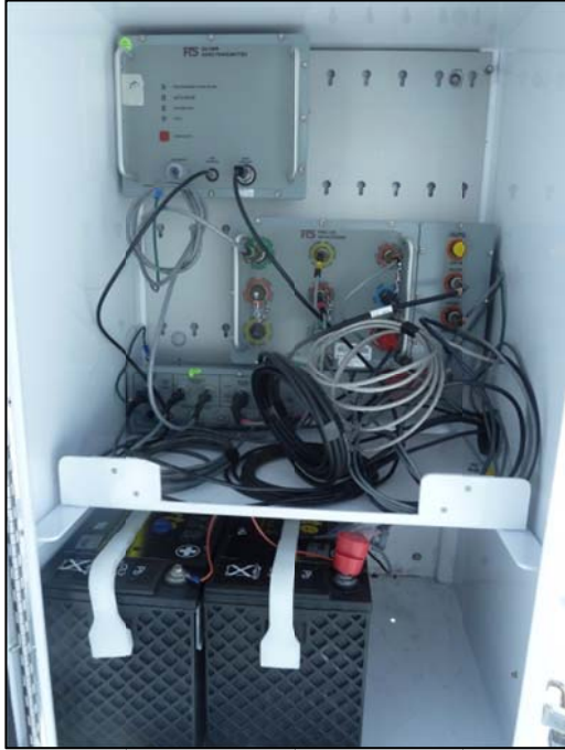
Figure 4. Chigmit Mountain RAWS - The inside of the instrument enclosure photographed just before departure.
