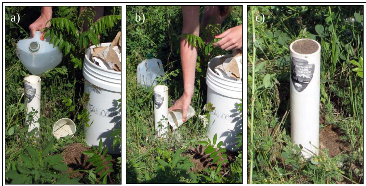
Figure S2.6. Installation of the PVC pipe benchmark, a) and b) Inserting the cement, water and sand into and around the pipe, and c) NPS logo on PVC pipe.
