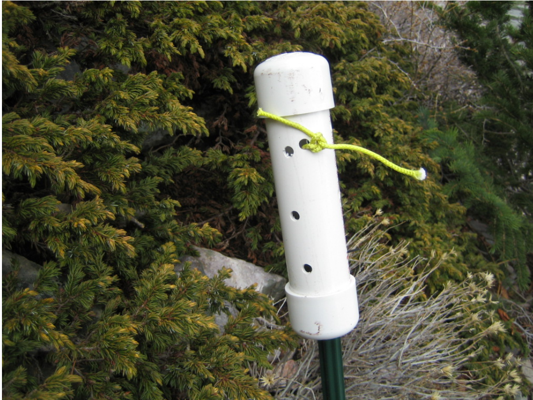
Figure SOP 10.4. PVC stilling well used to house logger.
