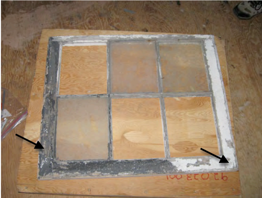
Figure 9. Cape Lookout Lighthouse, October 2008. A salvaged window sash currently located at the North Carolina Maritime Museum. Two samples were removed from the exterior face of the sash (arrows). Photograph by author.
