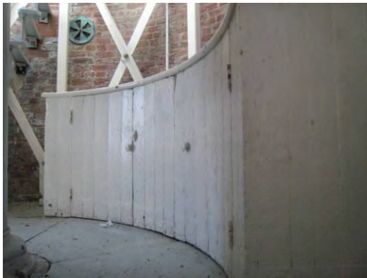
Figure C-91 Two-door cabinet in Eighth Floor Watch Room.
