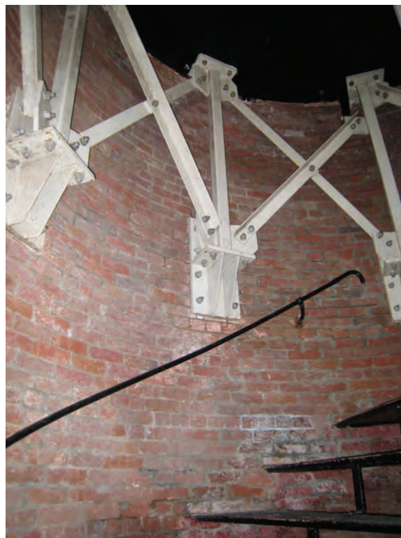
Figure C-16 1989 steel framing at Seventh Floor.
