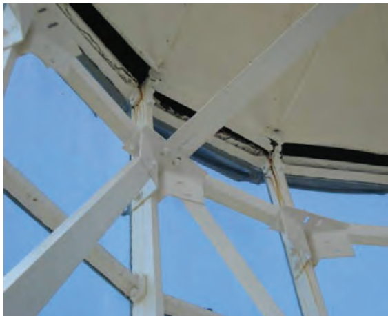
Figure C-100 Metal ceiling panels.
