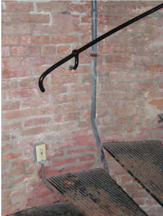
Figure C-46 Original iron handrail of 1-inch diameter.
