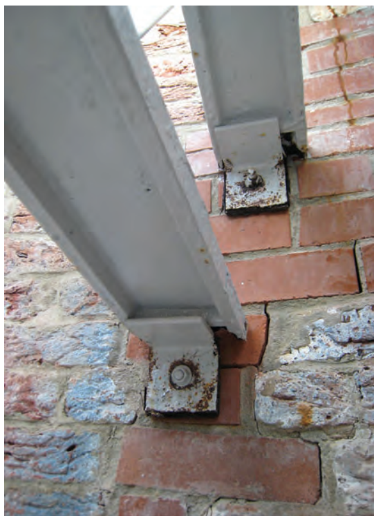
Figure C-8 Modern masonry repairs in Watch Room.
