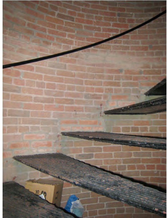
Figure C-62 Typical cast-iron treads of Spiral Staircase.
