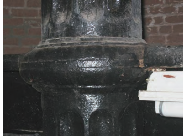
Figure C-14 Bolted connection between column sections.
