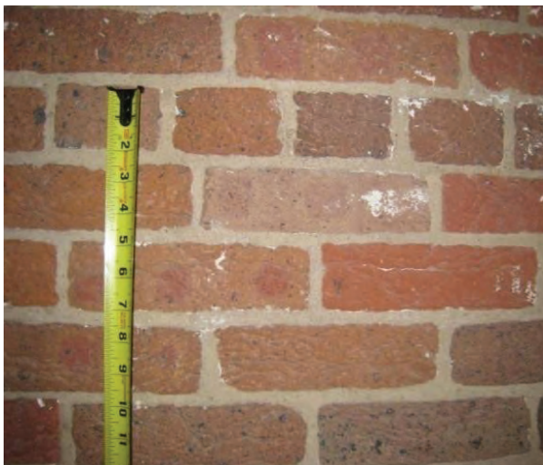
Figure C-9 Brickwork of interior face of core wall.
