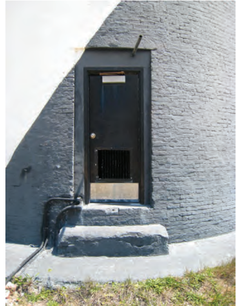
Figure C-28 Original masonry opening for First Floor doorway with modern infill and steel door.
