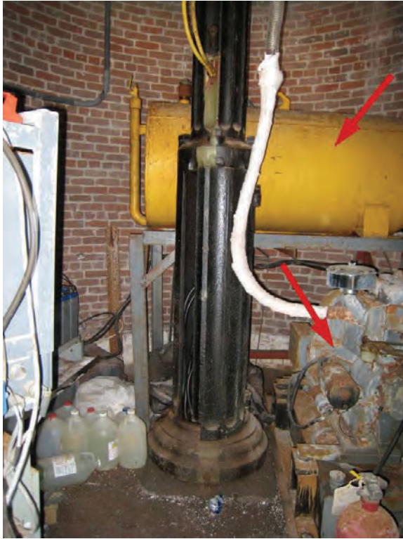
Figure C-13 Center column on sandstone pedestal, abandoned emergency generator and fuel tank nearby.
