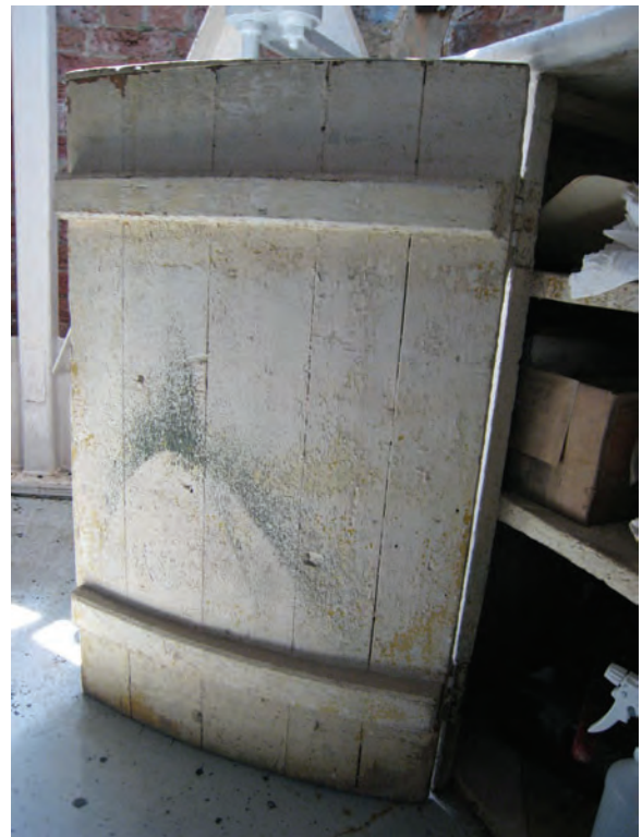
Figure C-92 Curved interior face of board-and-batten cabinet door.
