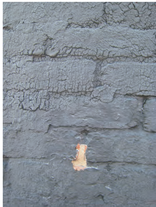
Figure C-108 Non-breathable coating on exterior masonry.
