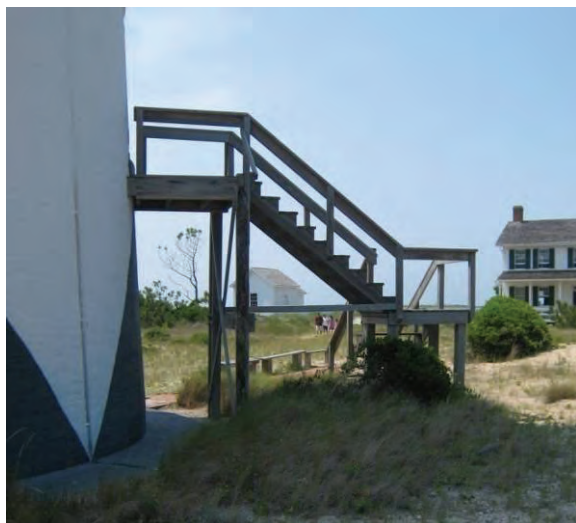
Figure C-35 Stairs for Main Entrance.
