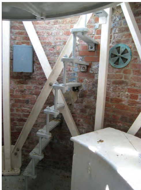
Figure C-89 Original cast-iron ship's ladder to Lantern.
