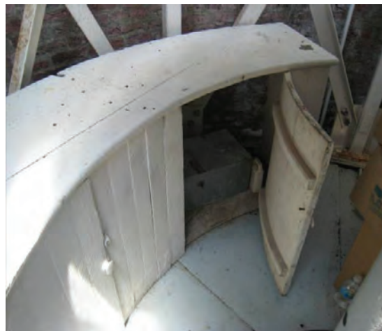
Figure C-51 Watch Room cabinet.
