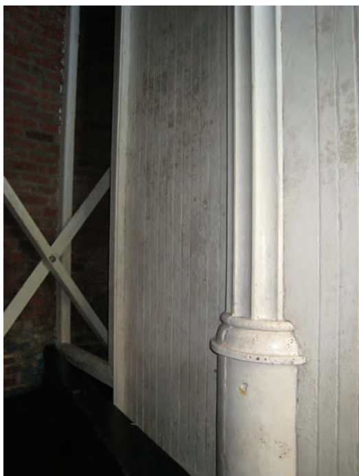
Figure C-77 1914 board wall and doorway at Seventh Floor landing. Note 1989 steel reinforcement added at masonry perimeter.
