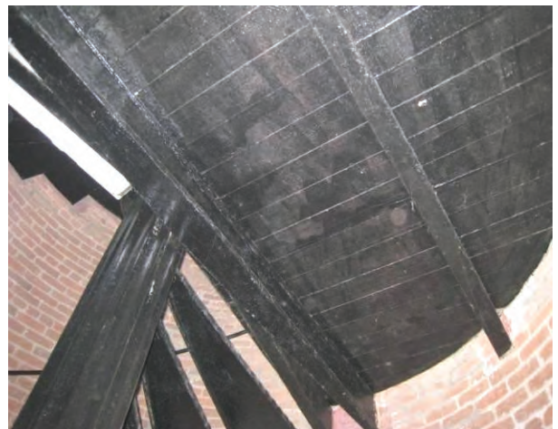
Figure C-66 Third Floor wood Landing.
