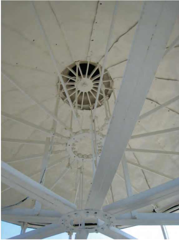
Figure C-17 Structural supports and central ventilator of dome.
