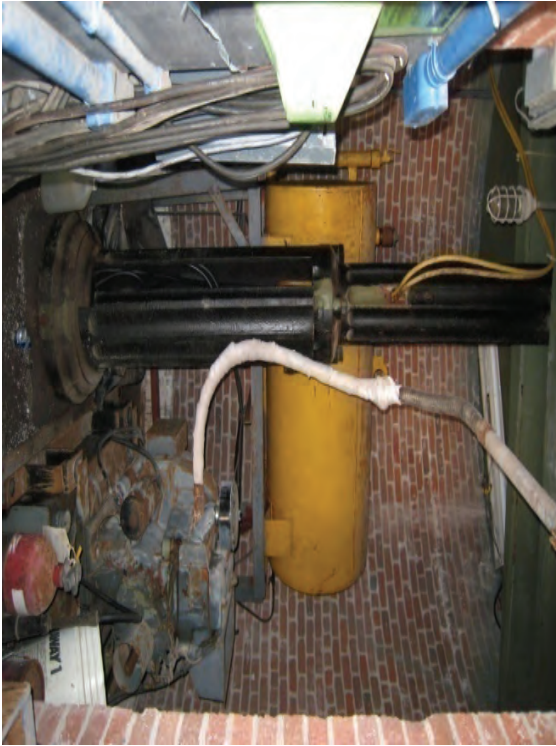
Figure C-56 View of First Floor Room from Passageway.
