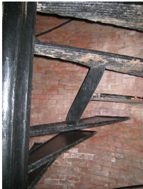
Figure C-73 1914 tread modification to accommodate the weight for occulting mechanism.
