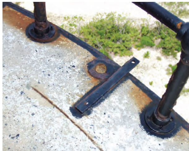
Figure B-14 Attachment location for radio antenna.
