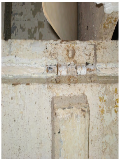
Figure C-94 Cabinet's five-knuckle hinge and batten.
