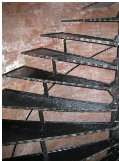
Figure C-74 Metal strap reinforcement of unknown installation date.
