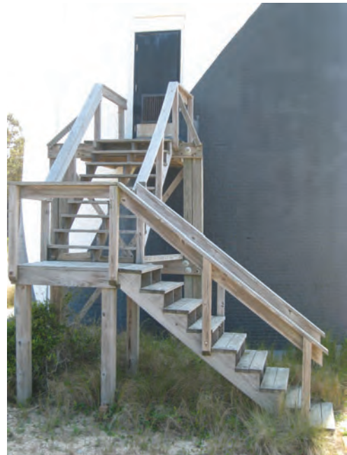
Figure C-29 Modern entrance stair to Second Floor.
