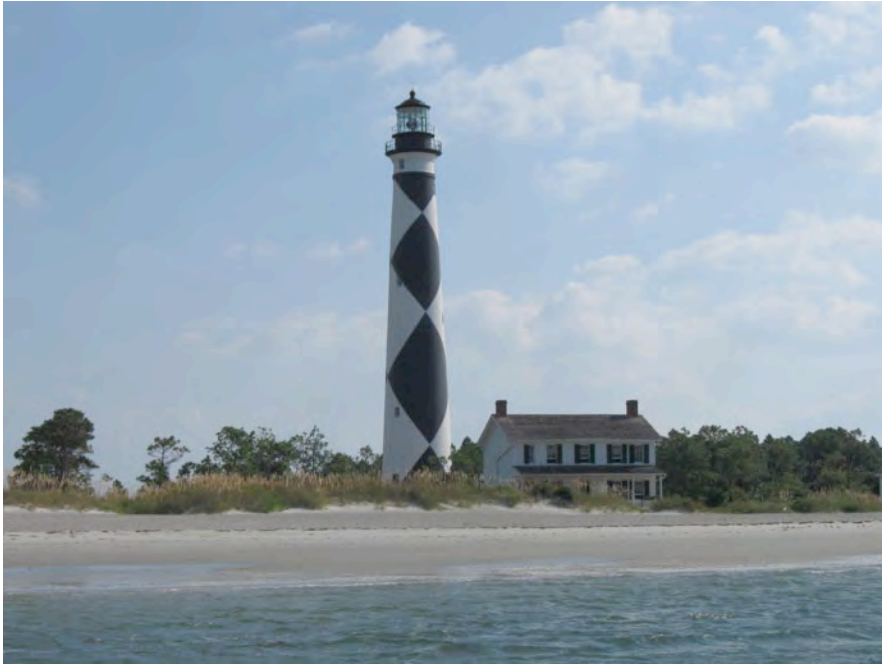
Figure 1. Cape Lookout Lighthouse, September 2008. Photograph by author.
