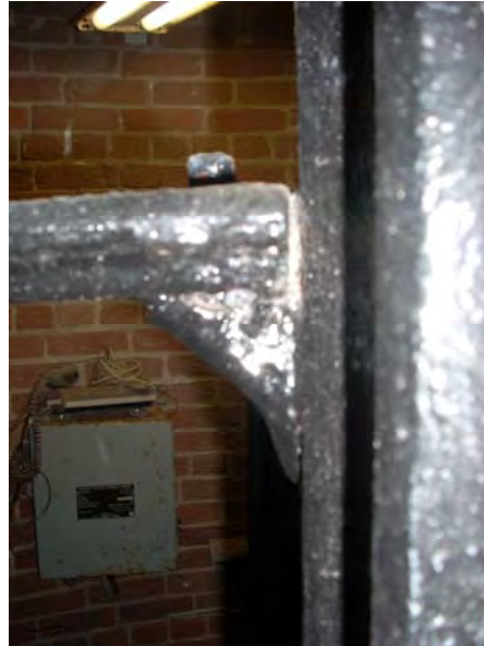
Figure 3 – Pin Connection at Interior Support Column
