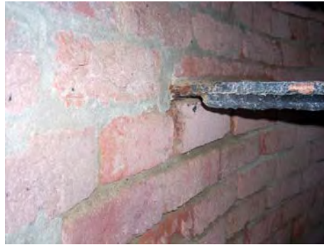
Figure 2 – Stair Connection at Exterior Masonry Wall
