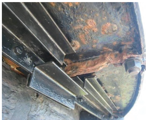
Figure C-106 Underside of Lantern Gallery reinforced in 1989.
