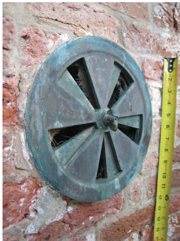
Figure C-95 Brass manual control for adjusting air flow.
