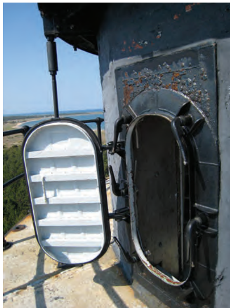
Figure C-30 Ship's Hatch at Observation Deck
