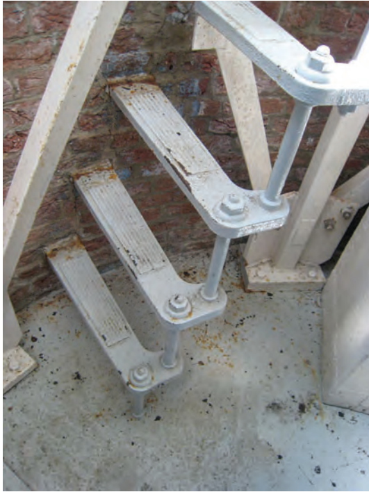
Figure C-90 Close-up view of ship's ladder to Lantern.
