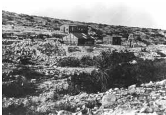
Miners worked several small-scale guano operations in the minor caves of the Guadalupe beginning in the 1890s. Soon after the turn of the century, the largest of these operations was the Bat Cave, today's Carlsbad Caverns. This photograph shows the above-ground facilities at the Bat Cave that existed in 1924. The A-frame hoist and bucket are at right. (Courtesy Southeastern New Mexico Historical Society of Carlsbad)
