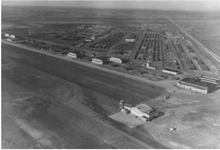
During World War II Carlsbad Army Air Field sprang into existence southwest of town as a training facility for navigators and bombardiers. When the war ended, the base disappeared almost as quickly as it had appeared. This aerial photograph was taken shortly after the base closed in 1945. (Courtesy Southwestern New Mexico Historical Society of Carlsbad)
