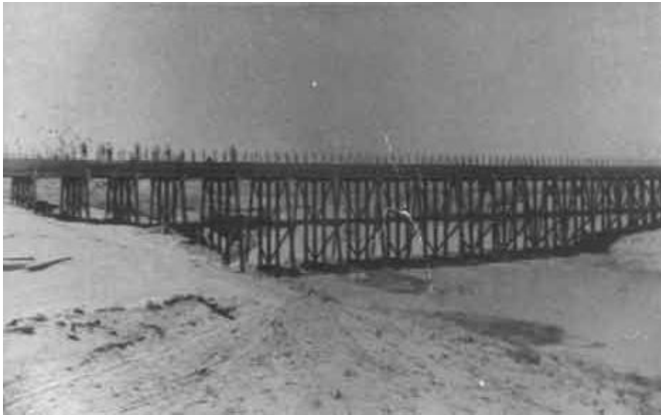
One of the pivotal structures in the original irrigation system near today's Carlsbad was this large wooden flume which carried the main canal across the Pecos River. Floods would periodically destroy the structure – and shut down the irrigation system – several times, before a concrete flume replaced the wood one. (Courtesy Southeastern New Mexico Historical Society of Carlsbad)
