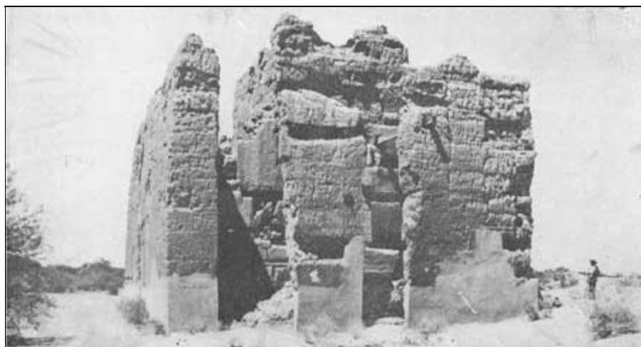
Casa Grande about 1892, from southwest.
