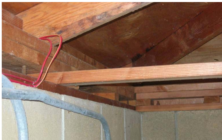
Figure 42: Joists, Top Plates, and Anchor On CMU Wall
