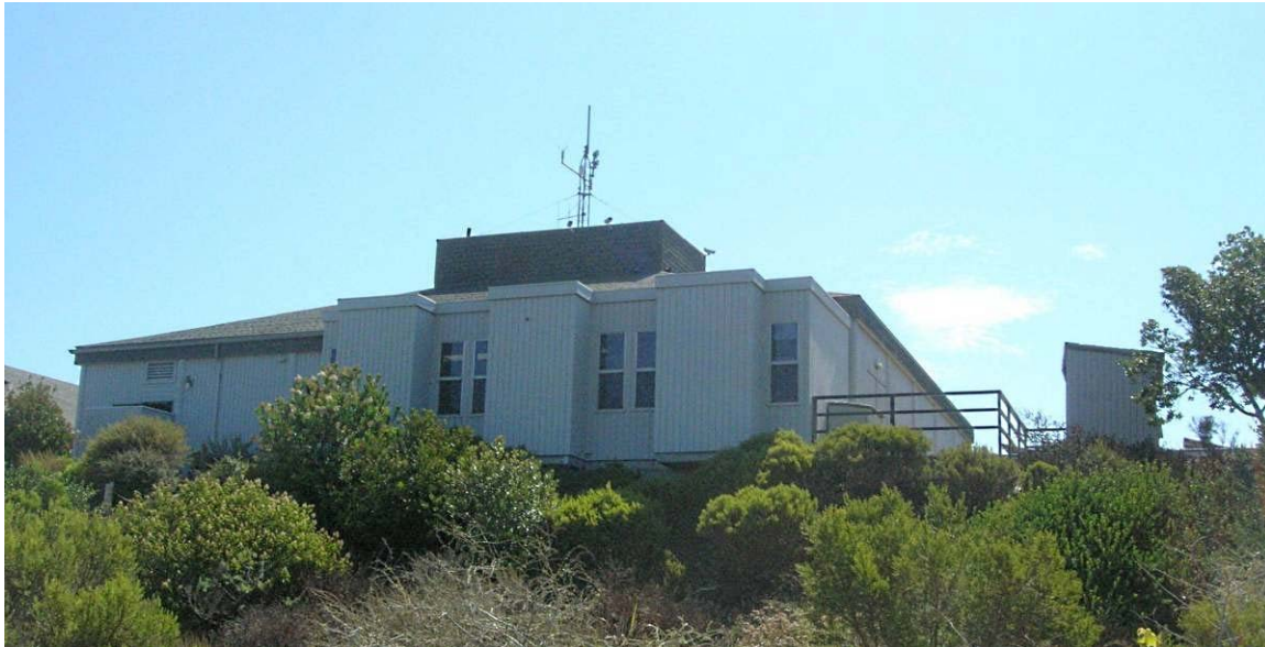
Figure 18: Auditorium/Museum West Facade and Extension
