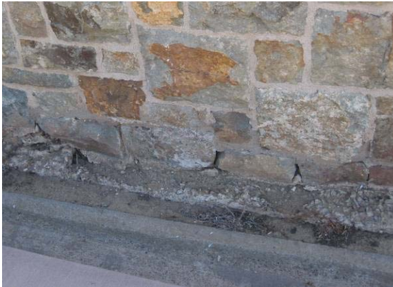
Figure 31: Mortar Deterioration
