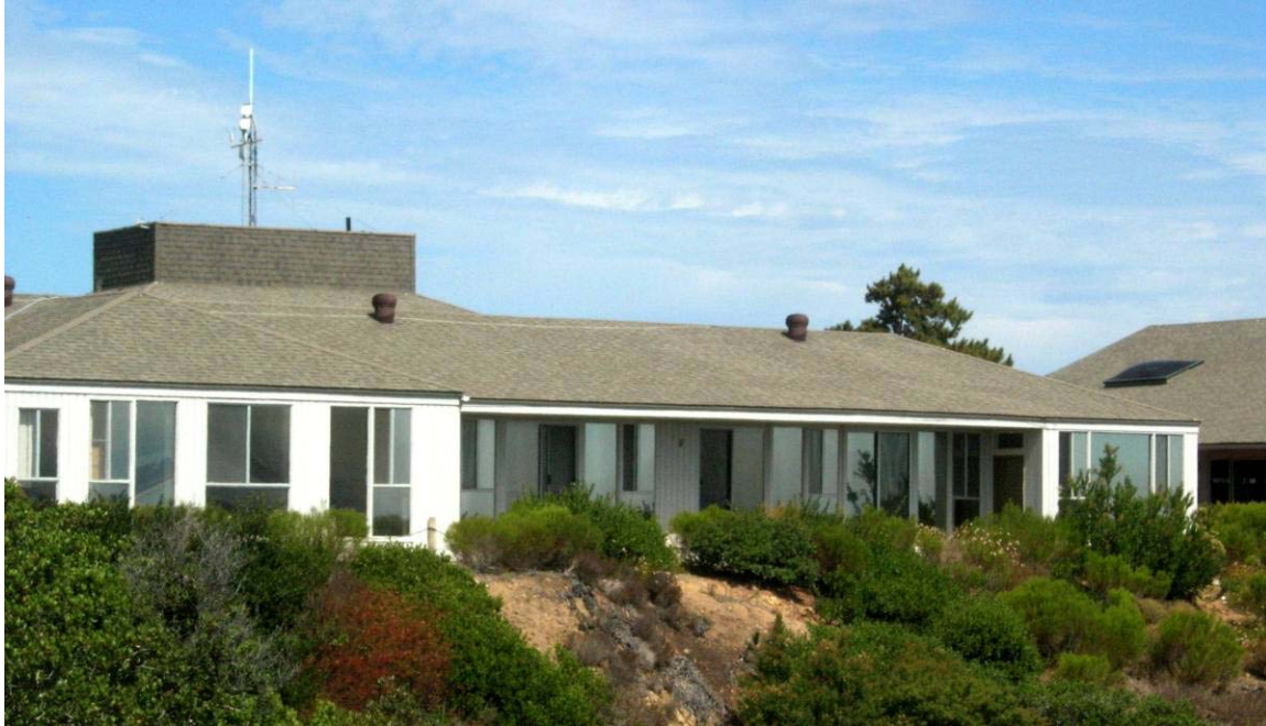
Figure 11: Administration Building East Facade
