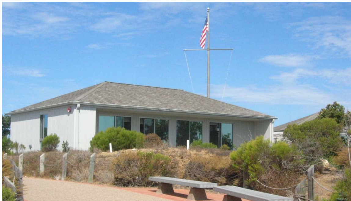
Figure 16: Visitor Contact and Law Enforcement Support Building East Facade
