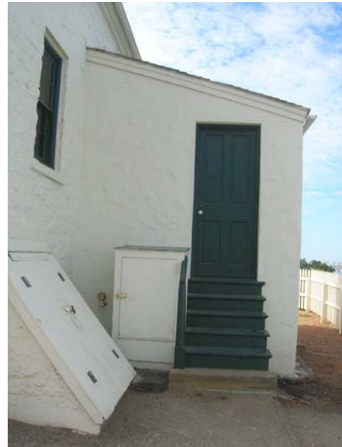
Figure 25: Lean-To Entrance on North Wall
