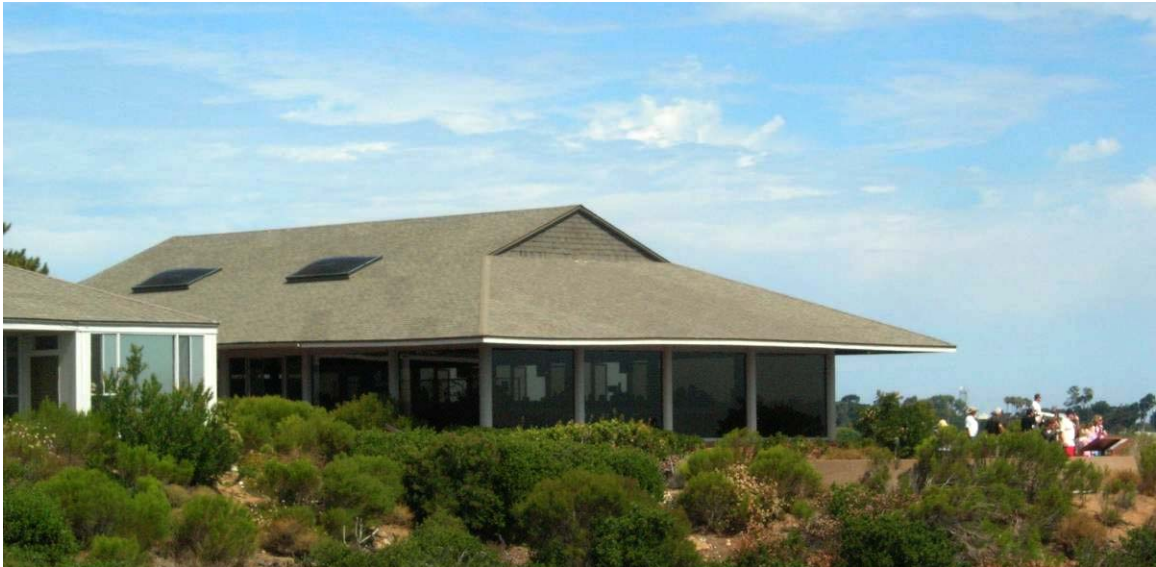
Figure 4: Visitor Center View Building East Facade
