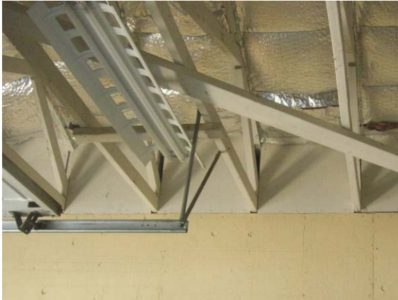
Figure 37: Plywood Between Rafters
