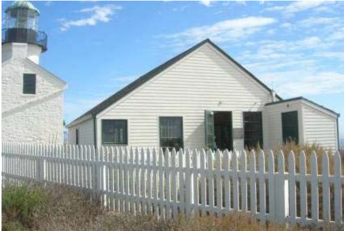
Figure 27: Assistant Lighthouse Keepers Quarters South Facade
