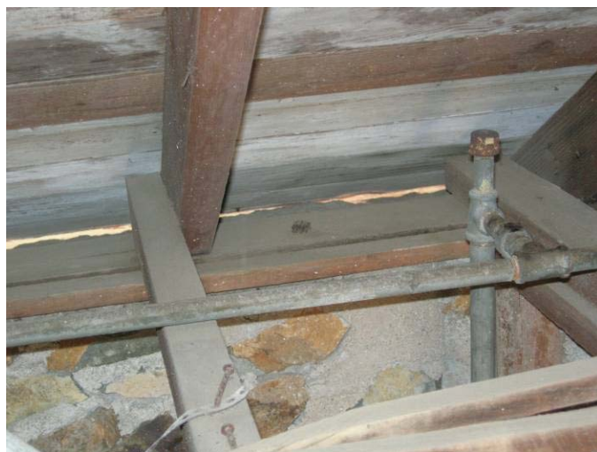
Figure 30: Roof Rafter, Top Plate, and Ceiling Framing
