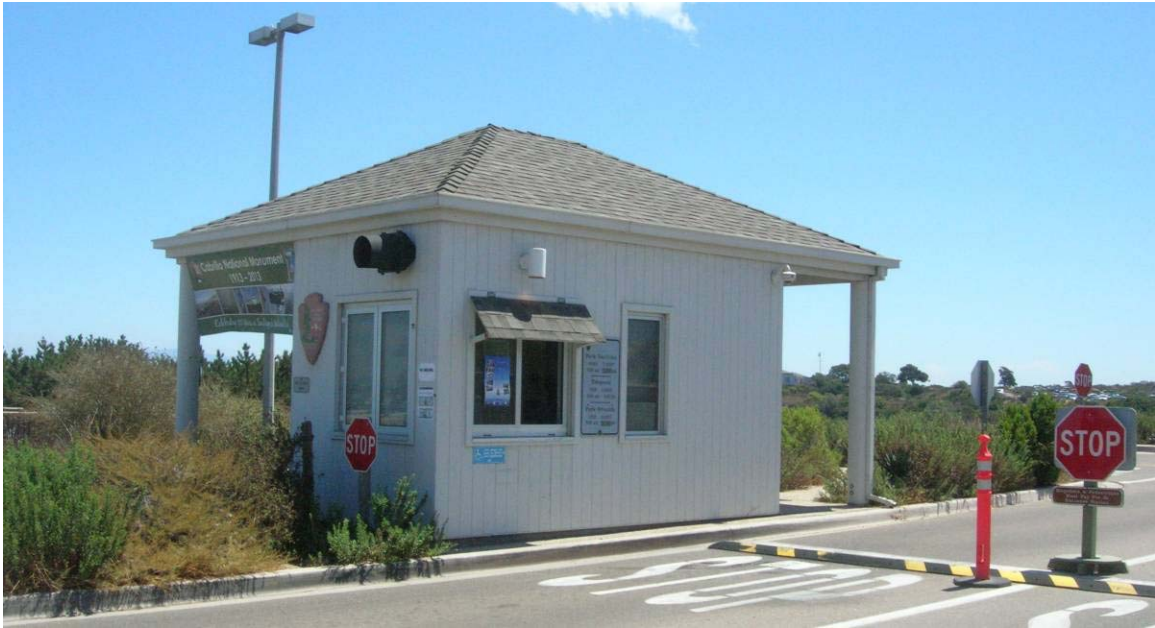
Figure 33: Entrance Station Building
