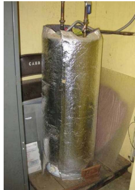
Figure 38: Unbraced Water Heater
