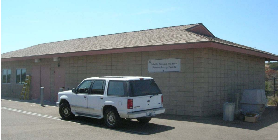
Figure 44: Curatorial Building (Museum Storage Facility)
