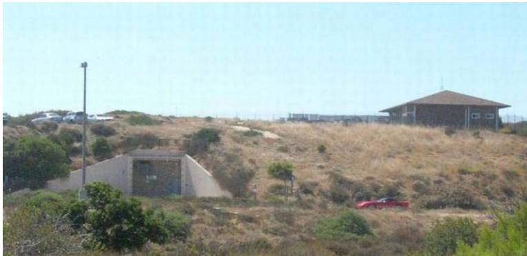
Figure 36: Bunker Entrance (Left) Upper Maintenance (Right)
