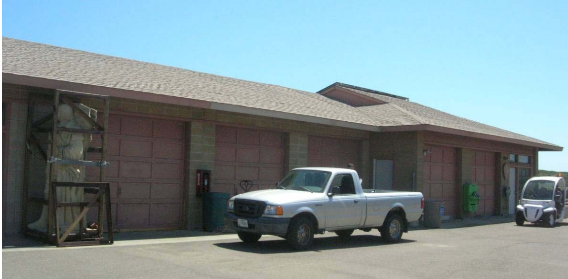
Figure 40: Lower Maintenance Facility
