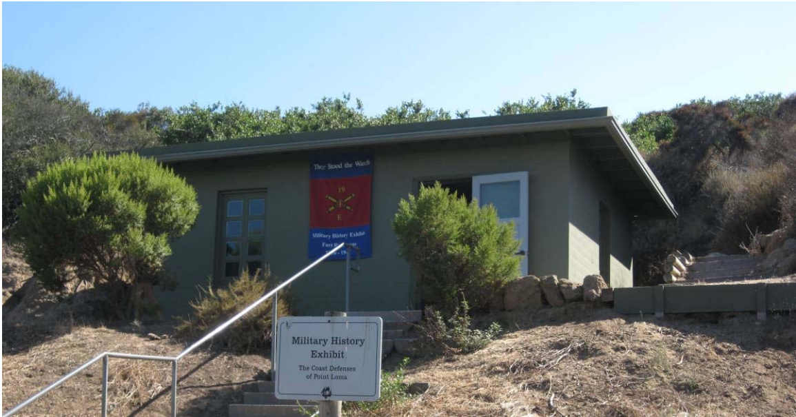
Figure 22: Military History Museum (Radio Room) North Facade
