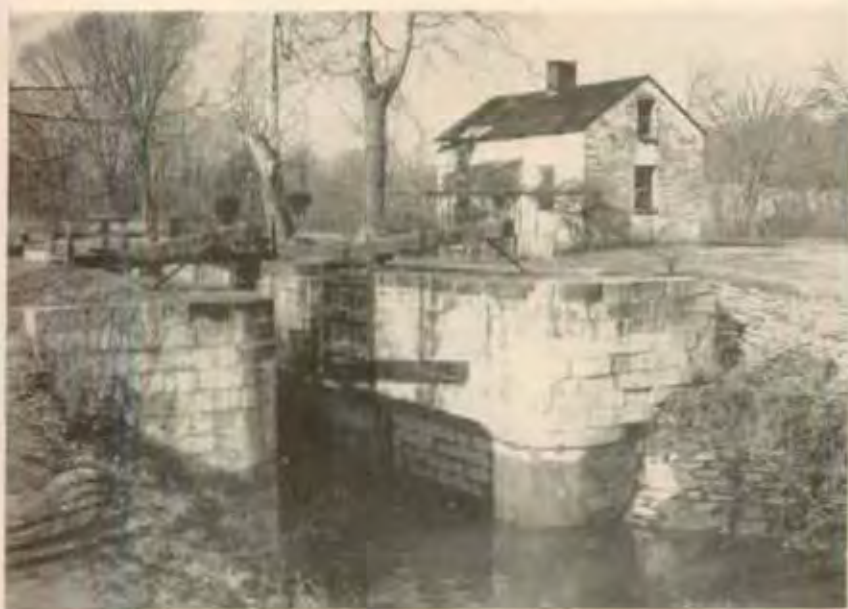
Typical lock house and lock.
