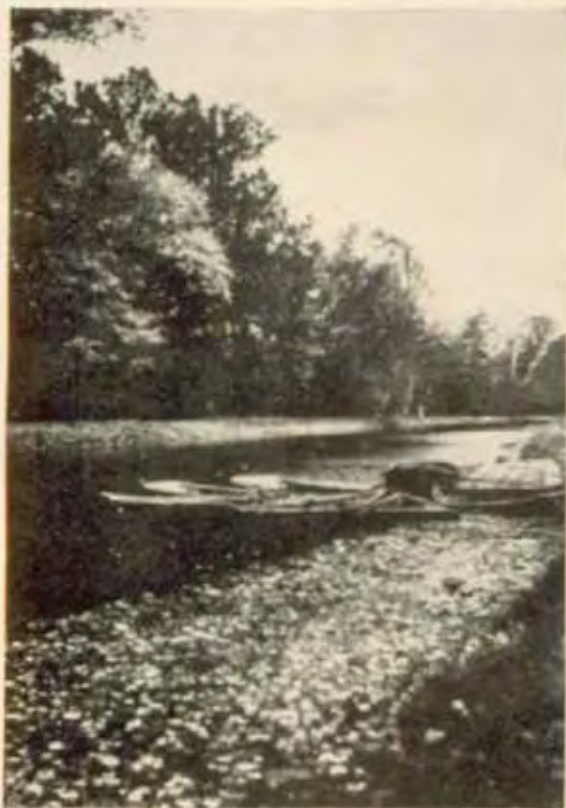
Section of restored canal near Seneca.
