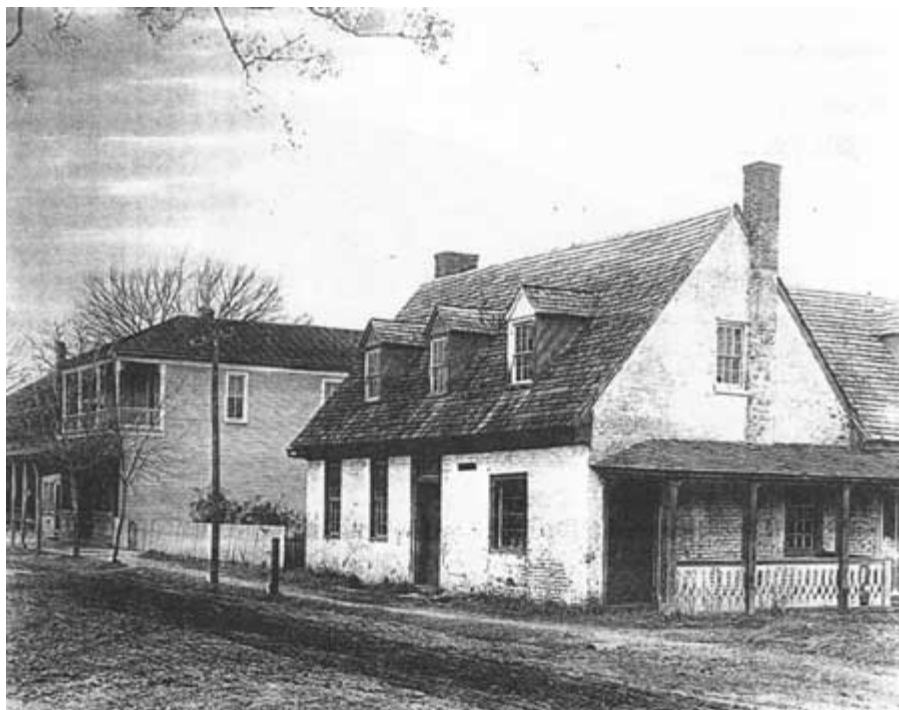
Photograph 9: View of the Digges House from the south, across a rutted dirt Main Street, with a telegraph pole to the left. The house seems to have declined somewhat. All shutters have been removed from front and visible right windows. A solid front door has replaced the glazed leaves, and an old nail-studded leaf is in the right front door. There are nine-over-nine sash with wide muntins in the right window lighting the right front room, perhaps the earliest surviving sash visible in any of the photographs. A small rectangular sign has been attached to the right of the front door transom.
