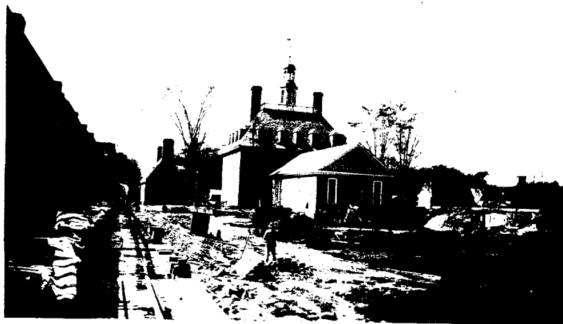
Governor's Palace - Restoration work underway (III,ii,B)
