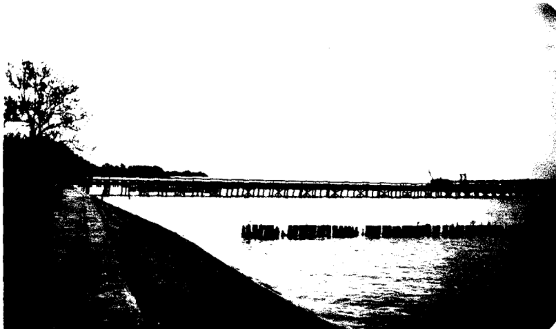
Sea Wall and Government Pier
