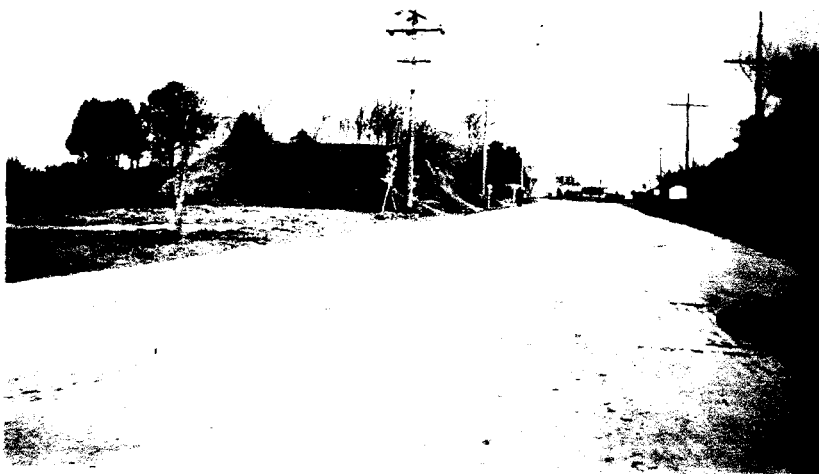
Exterior, looking in, northward
