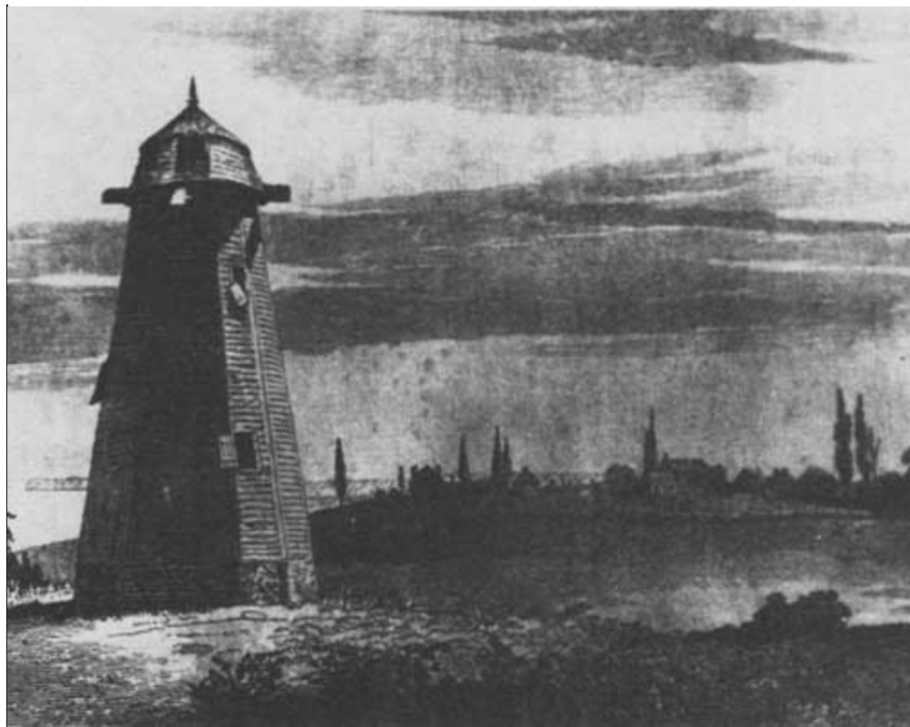
No. 6B The old windmill tower at Yorktown much in disrepair prior to 1840.
