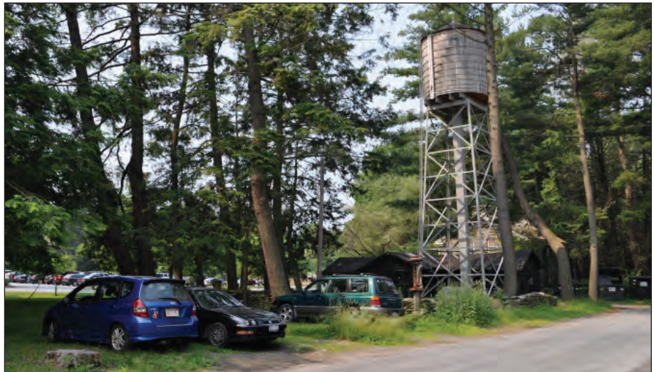
Figure 2.21. Buildings and Structures. View looking southwest toward the water tower and pump house, which stand adjacent to the water tower. The Wallace Center parking area is in the background of this photo (OCLP 2011).
