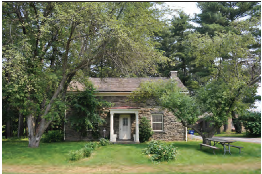
Figure 3.29. View looking north toward stone house, 2011. Two mature apple trees stand in front of the house. The old garage remains in the far right (OCLP 2011).
