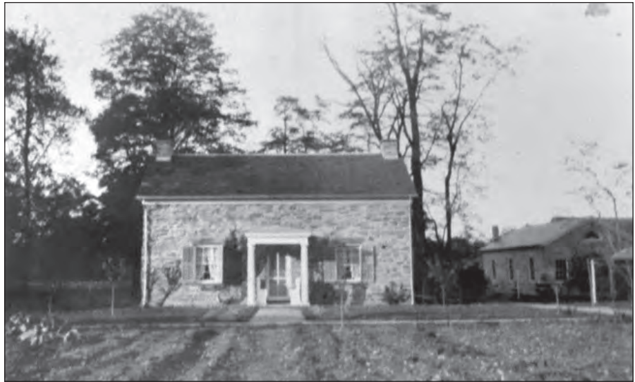
Figure 3.28. View looking north from the vegetable garden of the stone house in 1907, which was built in 1807. Young fruit trees line the gravel pathway in front of the house. The old garage stands in the far right behind the stone house (Newbold-Morgan Collection, ROVA Archives).
