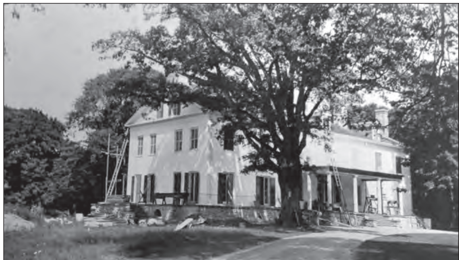
Figure 1.22. Bellefield house during renovations, 1911. View looking northwest toward the house from the main entrance drive. The tree at the corner of the porch is a white oak (Newbold-Morgan Collection, ROVA Archives).
