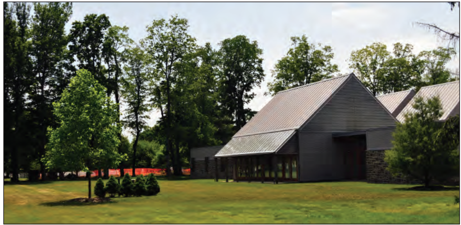
Figure 4.19. New plantings at septic system, 2012. View looking southwest toward the Wallace Center. The new tree and shrubs grow in front of the system control box (OCLP).
