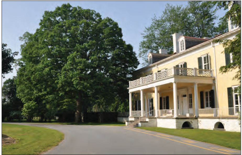
Figure 4.6. Main entrance drive, at the Bellefield house, 2012. View looking southwest toward the house and walled garden. The twenty-five foot wide drive area in front of the house does not currently reflect the historic character (OCLP).
