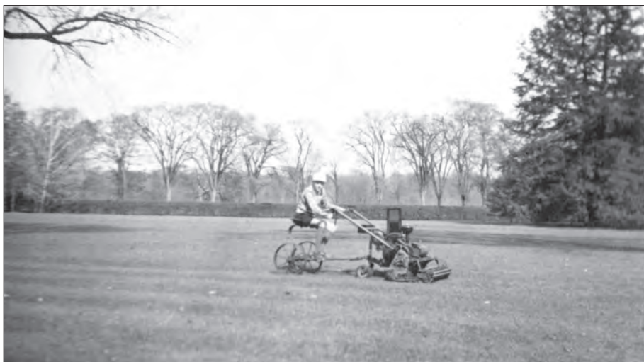
Figure 1.64. East lawn area within the main entrance drive, 1941. View looking east toward the Albany Post Road, elm trees, and hemlock hedge. One of the Morgan children operates a lawn mower. A single hemlock stands on the right side of the image (Newbold-Morgan Collection, ROVA Archives).
