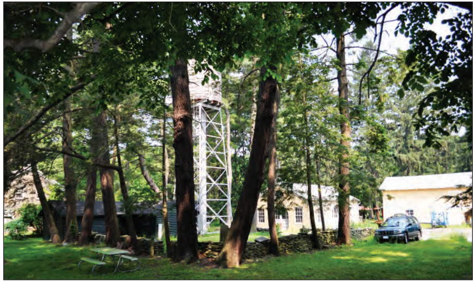
Figure 2.6. Spatial Organization. View looking northwest toward the cemetery and evergreen trees. The pump house, water tank, old garage, and old barn stand in the background (OCLP 2011).
