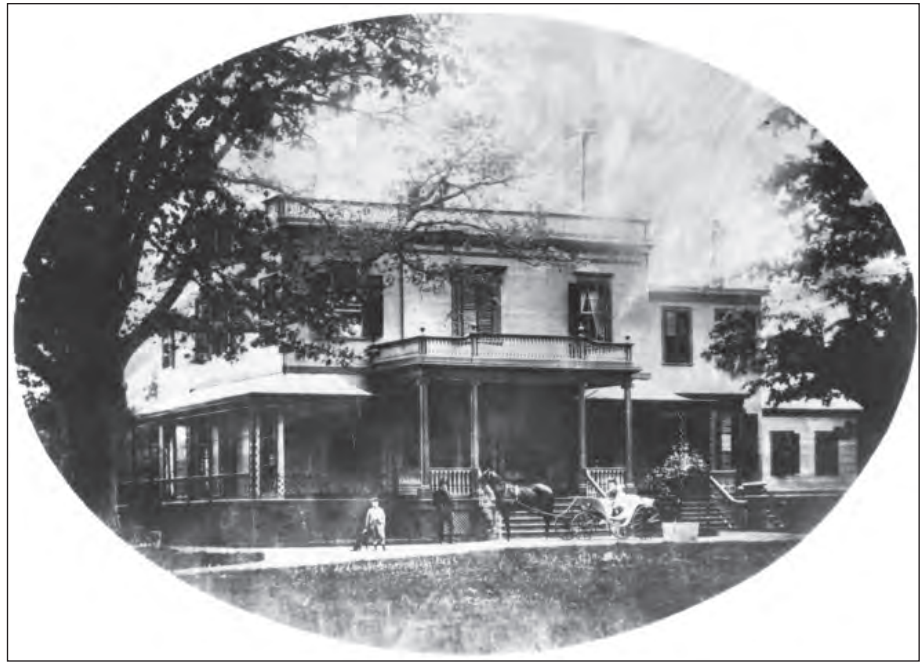
Figure 1.15. View looking northwest of the Bellefield house from the east lawn, c. 1900. The photo shows the renovation of the house from c. 1890 (Newbold-Morgan Collection, ROVA Archives).
