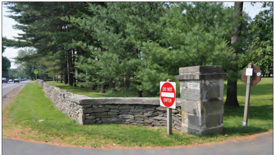
Figure 2.20. Buildings and Structures. View looking south along Albany Post Road from the south exit of the main entrance drive. The stone wall and pier are located at the entrance and exit of the main entrance drive. The wall continues onto the Roosevelt Estate (OCLP 2011).
