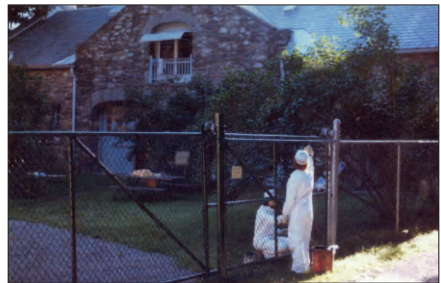
Figure 1.92. View looking northeast of the new garage, 1985. A fence encloses the service area (ROVA staff, Henry Van Brookhoven).
