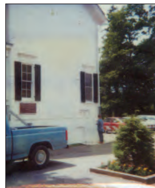
Figure 1.85. Staff parking, 1985. View looking southwest toward the north facade of the house. The planting area on the right was removed in 2004 (ROVA staff, Henry Van Brookhoven).
