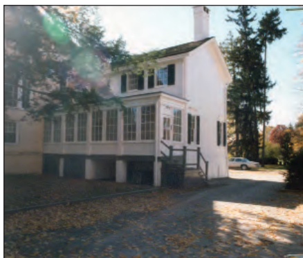
Figure 1.84. Bellefield house and Bellefield service road, 1986. View looking southwest toward the staff parking (ROVA staff, Henry Van Brookhoven).
