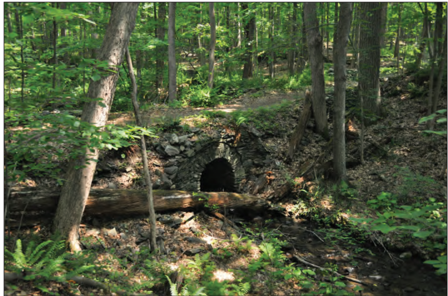
Figure 2.22. Buildings and Structures. View looking north toward one of the stone bridges on stone cottage road, within Rogers Land, west of Bellefield (OCLP 2011).
