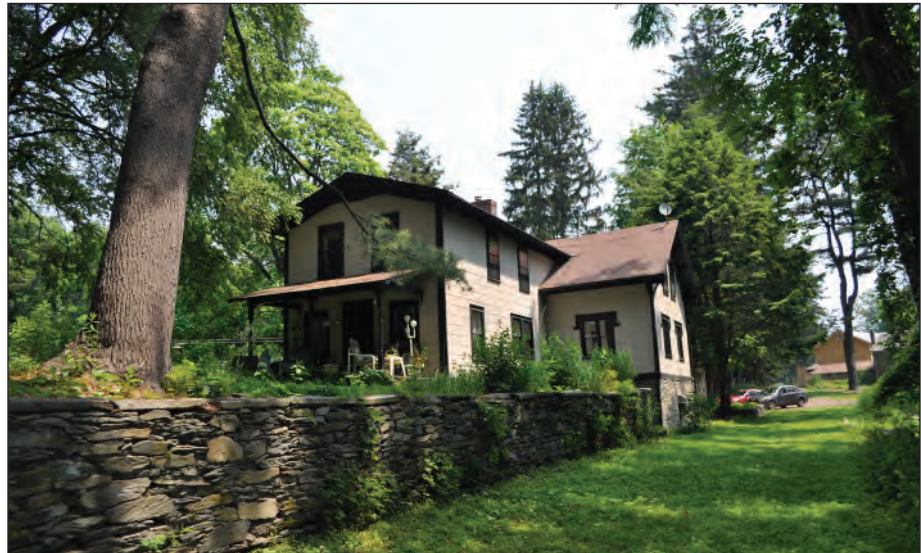
Figure 2.19. Buildings and Structures. View looking northwest toward the Bellefield cottage. This house is leased as a private residence by Scenic Hudson and stands outside of the park boundary (OCLP 2011).
