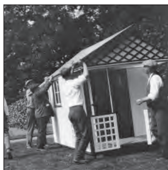
Figure 4.25. Playhouse, c. 1935. View looking northeast during the construction of the playhouse (Newbold-Morgan Collection, ROVA Archives).
