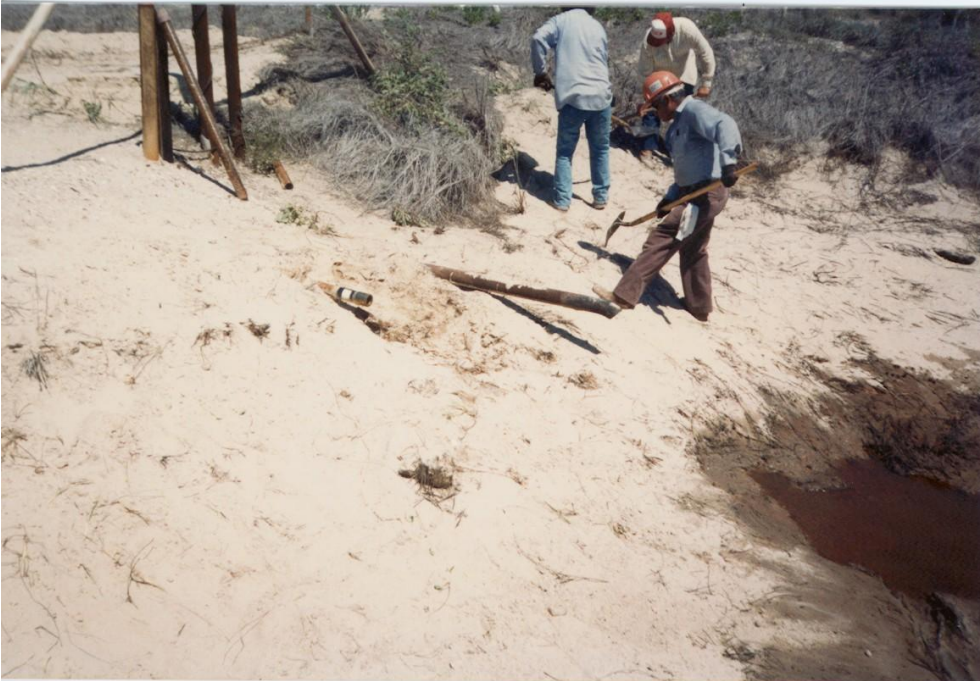
Amoco Sight 8/30/1989: Pipe is no longer draining.
