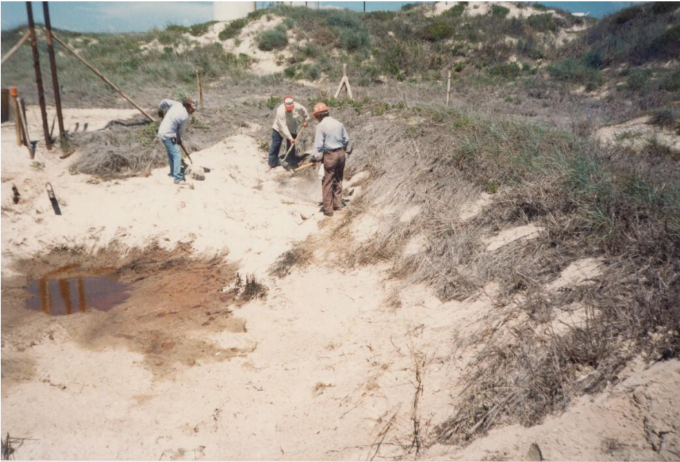
Amoco Sight 8/30/1989: Pond was pumped, scraped, and is in the process of being covered with fresh sand.
