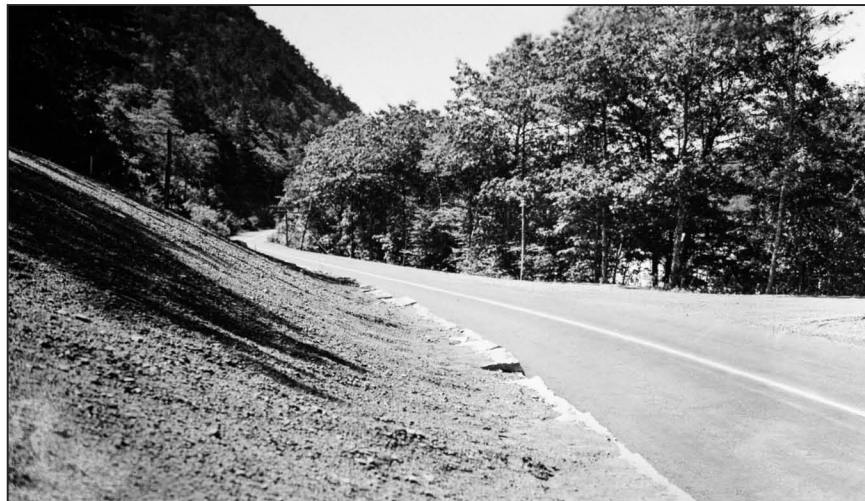
Figure 14. “Before” and “after” photographs along the Tarn, Kebo road extension, 1939-1940. (The Strout Family Collection - Ahlblad’s Frame Shop)
