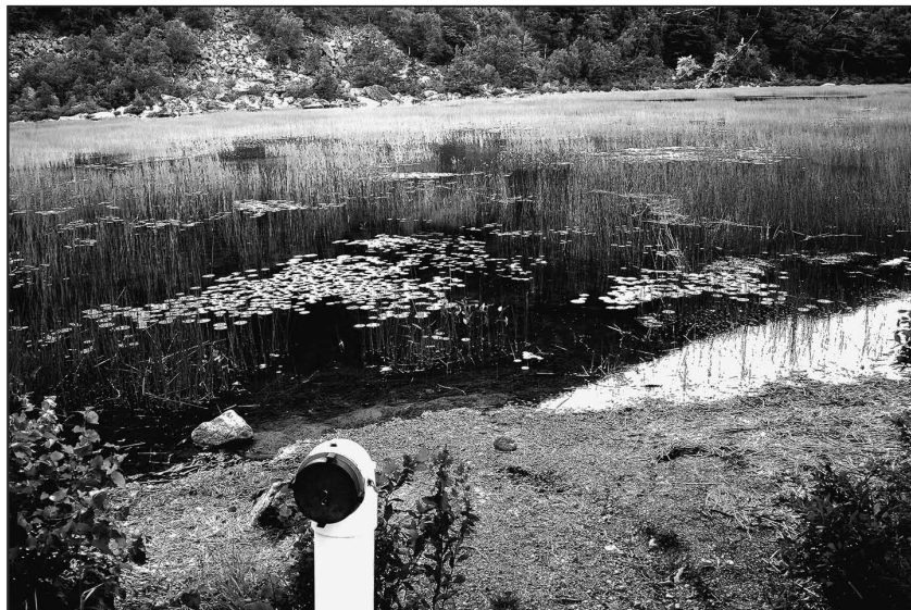
Figure 25. Dry hydrant at the Tarn, 2010.
