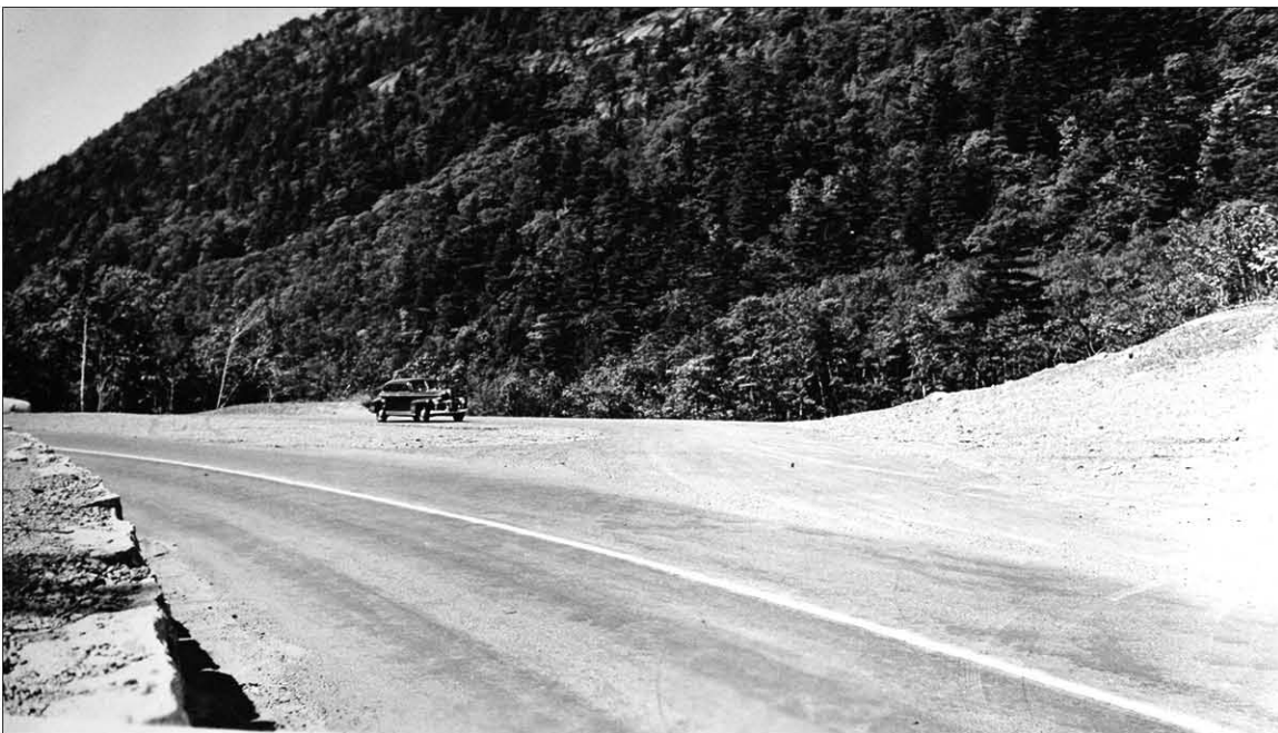
Figure 32. Parking area construction at the Tarn, "after" shot. 1940. (The Strout Family Collection – Ahlblad's Frame Shop)
