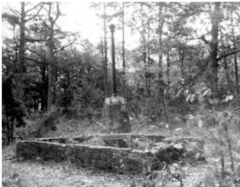
Figure 32: The Washington Light Infantry Monument in a deteriorated condition, 1975
