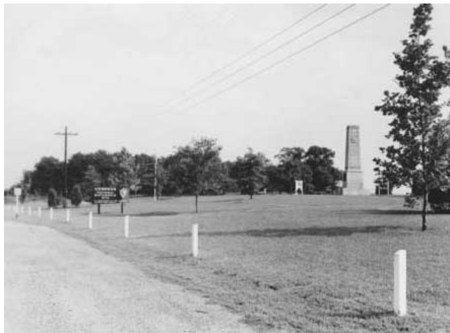
Figure 8: Cowpens NBS following Mission 66 improvements. Note the new place name sign, the two new exhibit cases on either side of the U.S. Monument, and the missing fence around the monument
