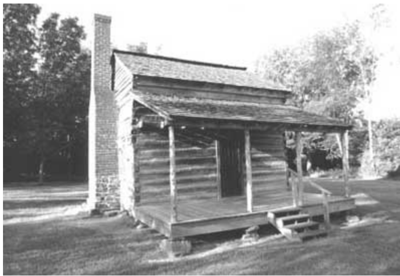
Figure 31: The Scruggs House after restoration, 1999
