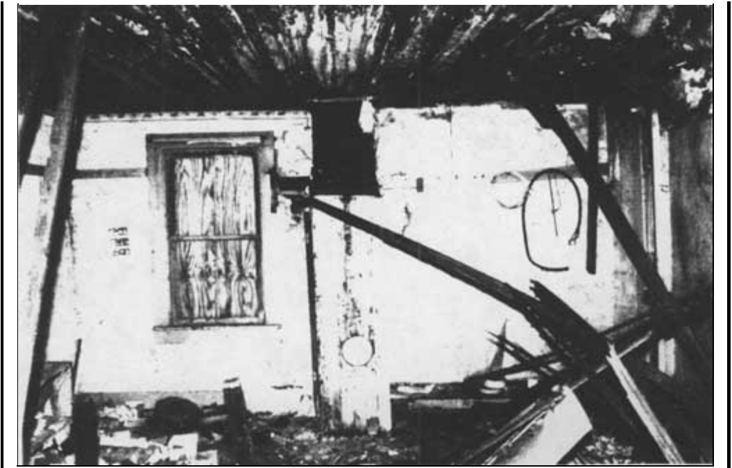
46. Room 104 South Wall
