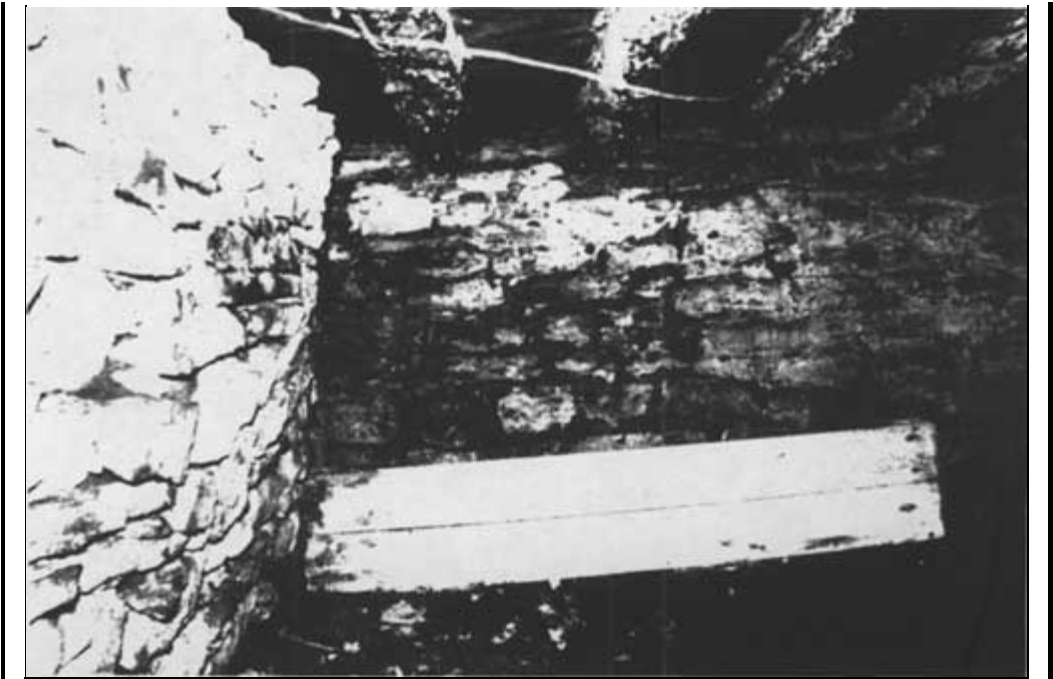
12. Room 001 Northwest Corner of Cellar
