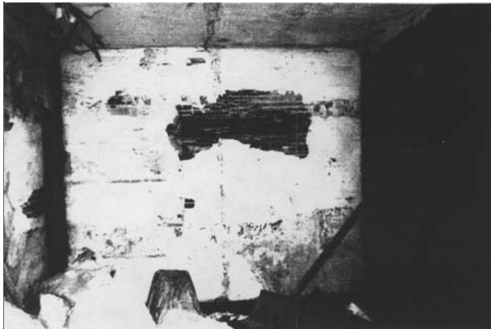
27. Room 102 East Wall
