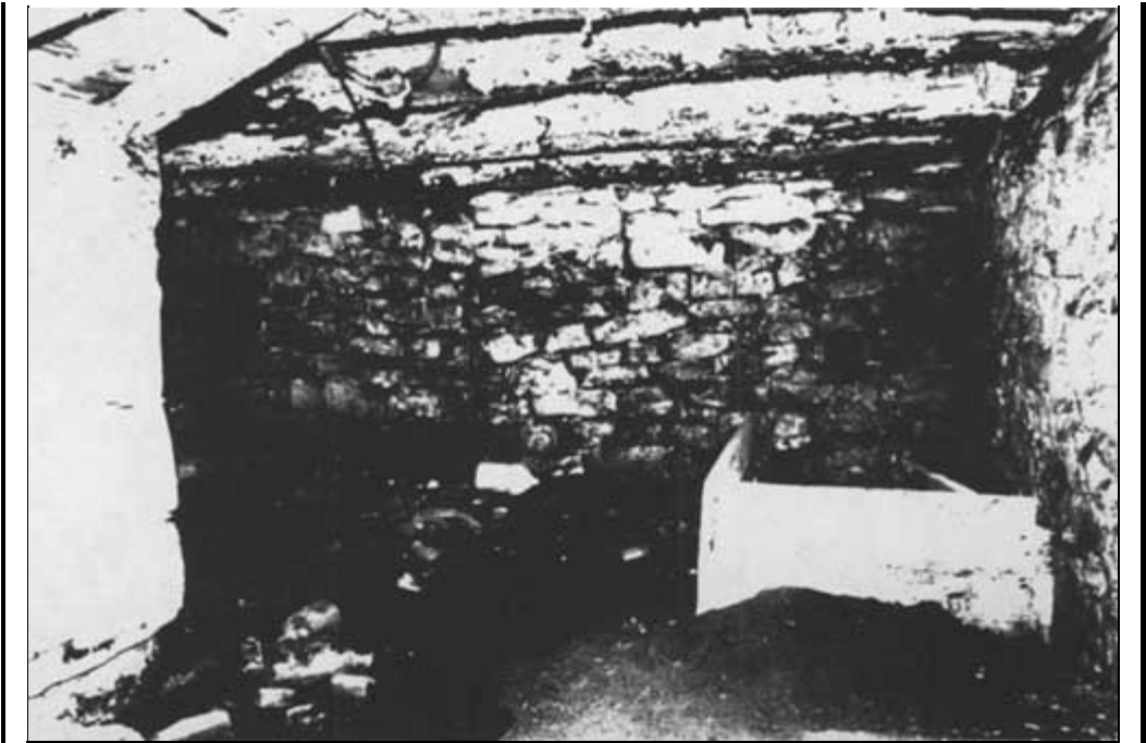
10. Room 001 North wall of Cellar
