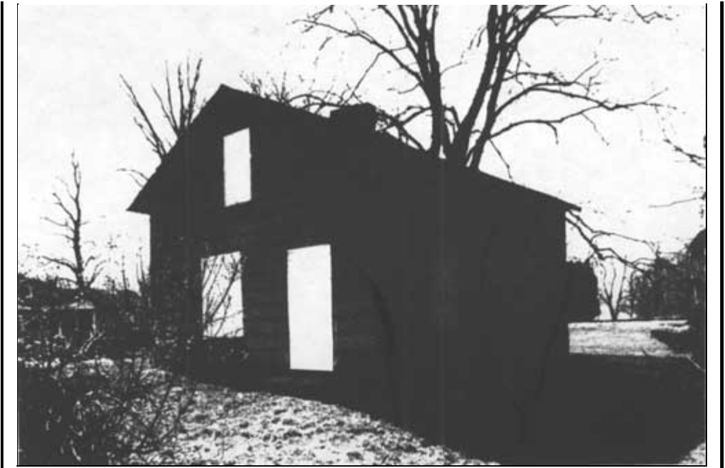
NORTH AND EAST ELEVATIONS OF MAIN WING
