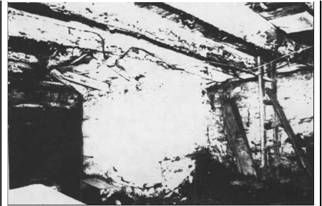
6. Room 001 West Wall of Cellar Cribbed timbered chimney footing
