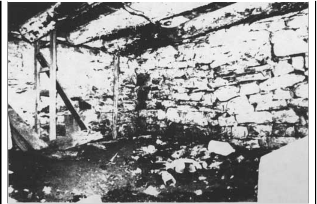
14. Room 001 Northeast Corner of Cellar
