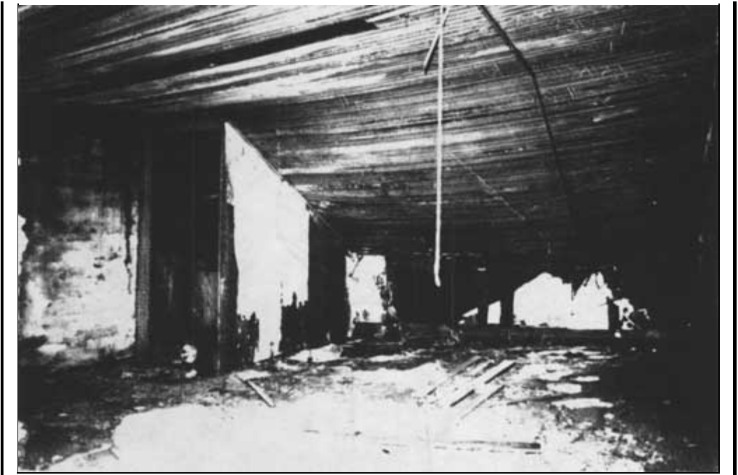
33. Room 203 Southeast Corner
