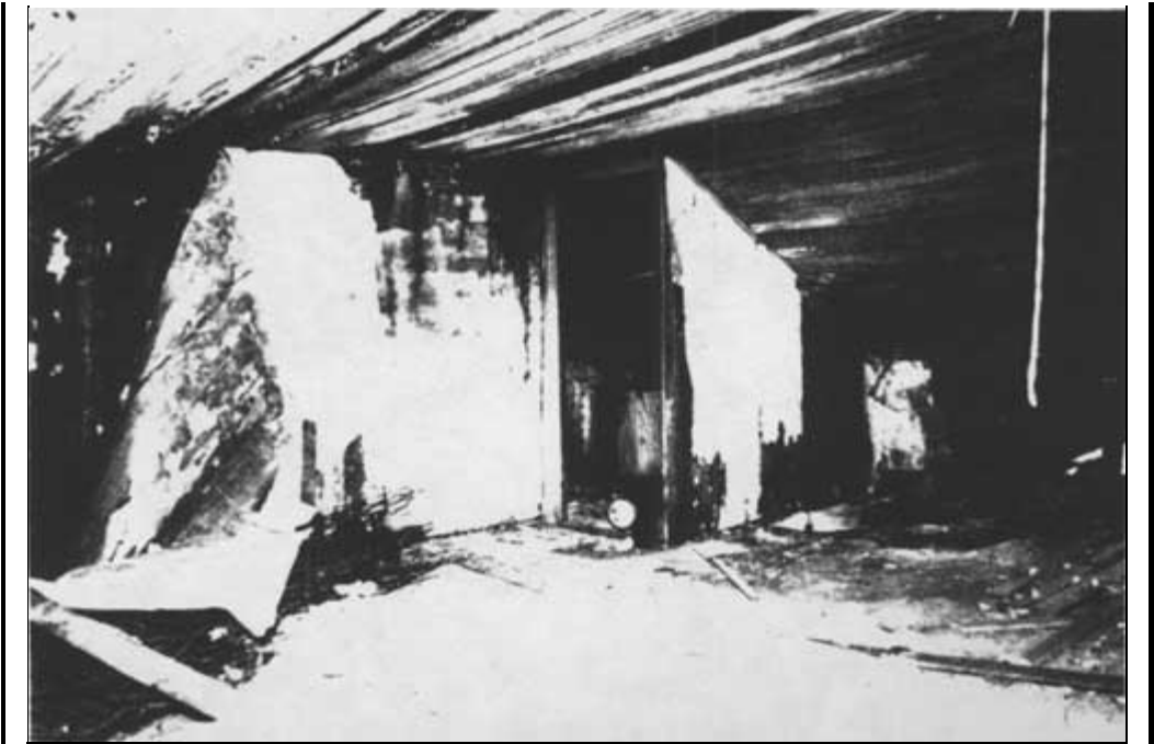
36. Room 203 Southeast Corner
