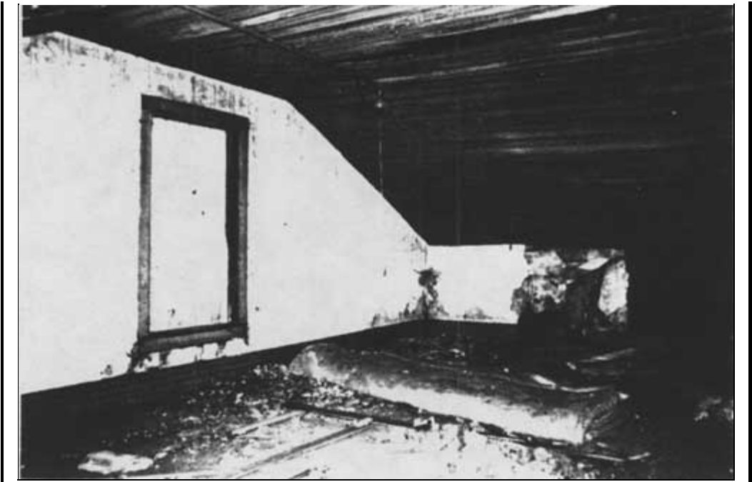
39. Room 203 Northwest Corner
