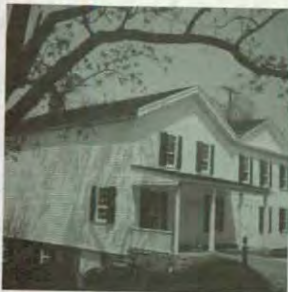
Once a tavern and store at Lock 38, this restored structure now serves as the Canal Visitor Center in CVNRA.
