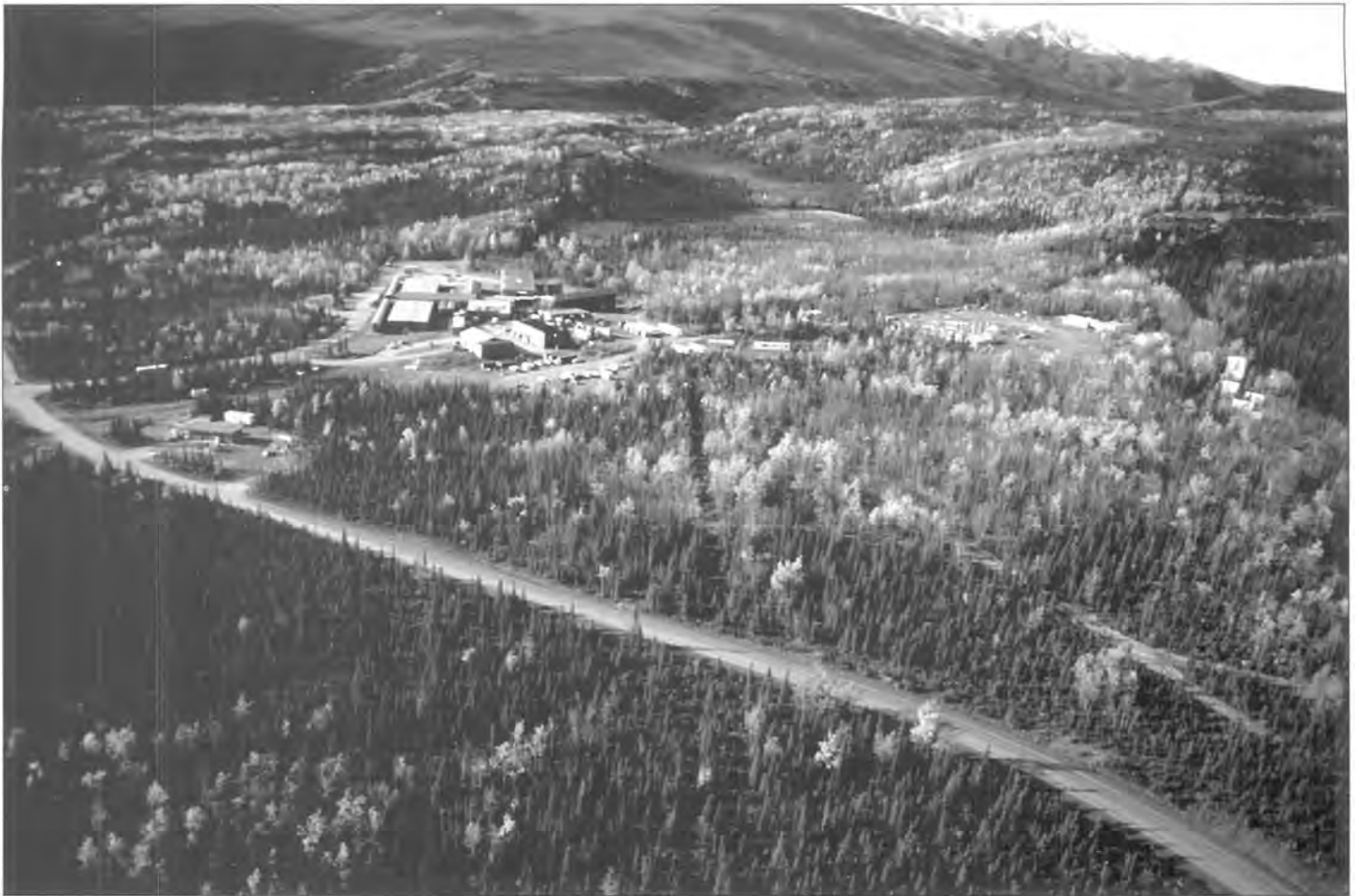
This 1980s view of the McKinley Park Hotel area shows concession employee housing in a clearing on the right, the temporary hotel in the center, and the original 1938 dormitory and powerhouse near the hotel. NPS Interp. Collection, #3502, Denali National Park and Preserve
