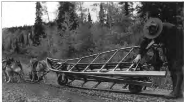
In 1939, ranger John Rumohr experimented with attaching wheels to a dog sled so it could be used for summer sled dog demonstrations. No other national park unit offered this interpretive activity, which was begun on a full-time basis in 1940. DENA 11-135, Denali National Park and Preserve Museum Collection
