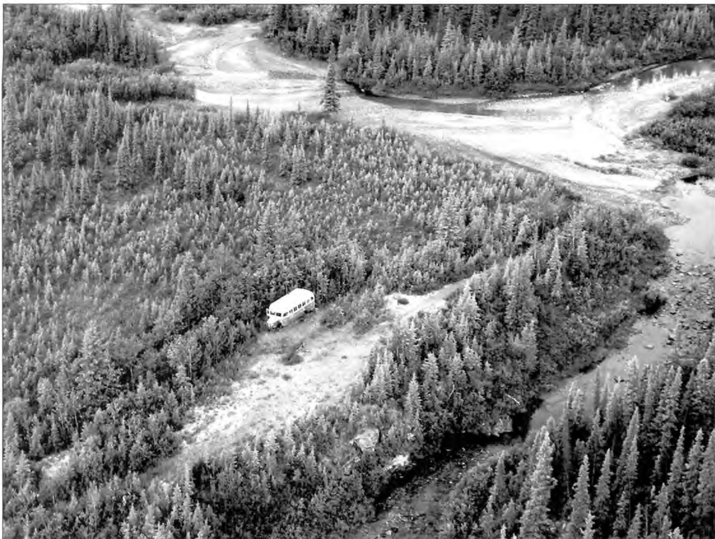
Where the Stampede Road crosses the Sushana River, a bus was left by the Stampede Road contractor. Since the 1960s it has been used as a temporary shelter by hunters, trappers and other travelers along the trail. NPS Photo
