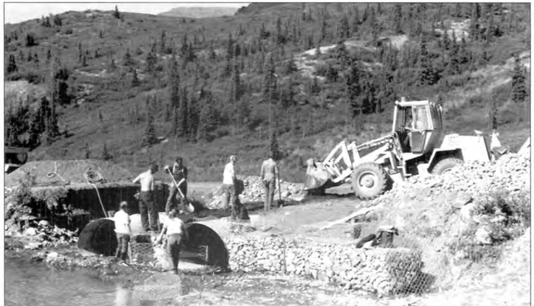
A park road maintenance crew replaced the wooden bridge at Hogan Creek with two large culverts in 1983. NPS Roads Office Collection, Denali National Park and Preserve
