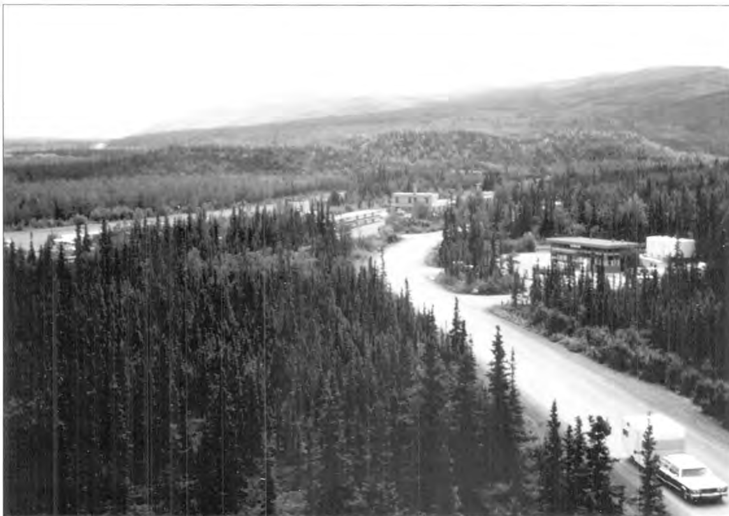
The original park entrance road passed the concession-run gas station and mercantile, on the right, and the Alaska Railroad depot, in the center. Federal Highway Administration, from "1984 Road Improvement Study"
