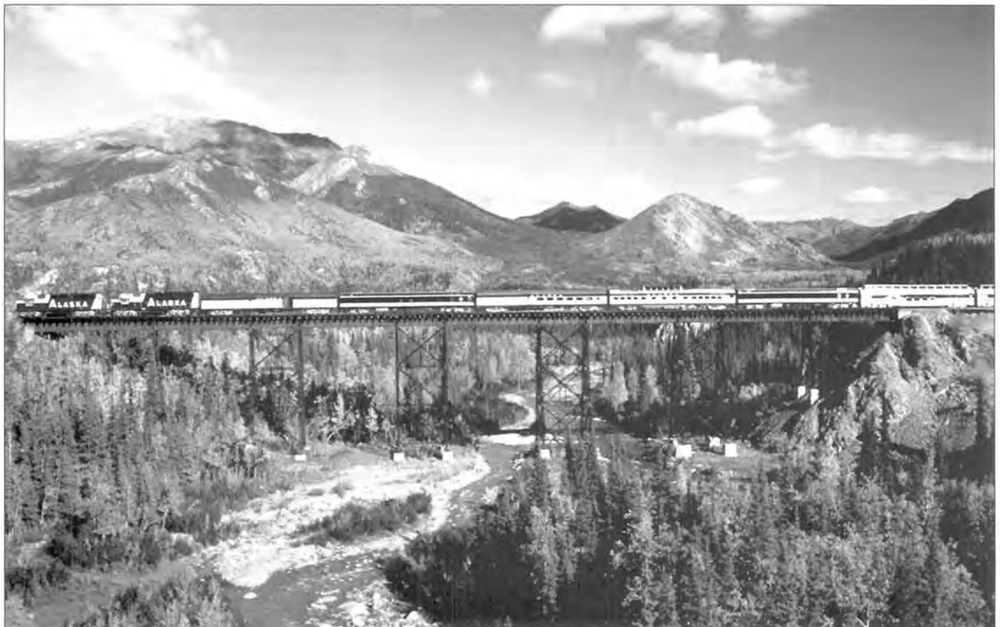
Tom Habecker Collection The Alaska Railroad crosses Riley Creek just south of the McKinley Station Depot. Tom Habecker Collection
