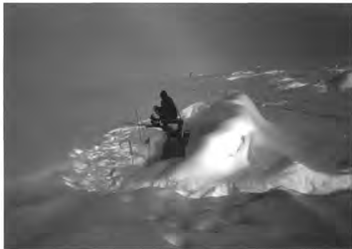
Rangers Nick Hartzell and Bob Butts created this simple outhouse design and constructed it in Talkeetna in 1977. The outhouse was placed above a 10-foot hole in the glacier. The last year for pit toilets at the Kahiltna Glacier Base Camp was 2005. Roger Robinson Photo
