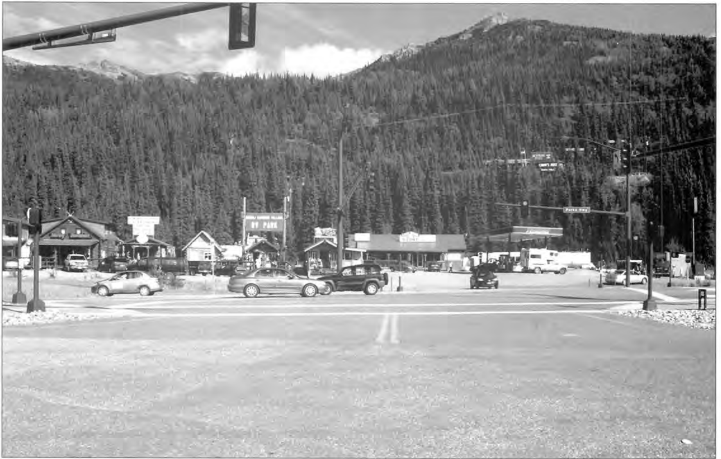
"Glitter Gulch" received the first two stop lights in the area in 2003 as part of the Alaska Department of Transportation program to improve safety along this busy section of the George Parks Highway. NPS Photo
