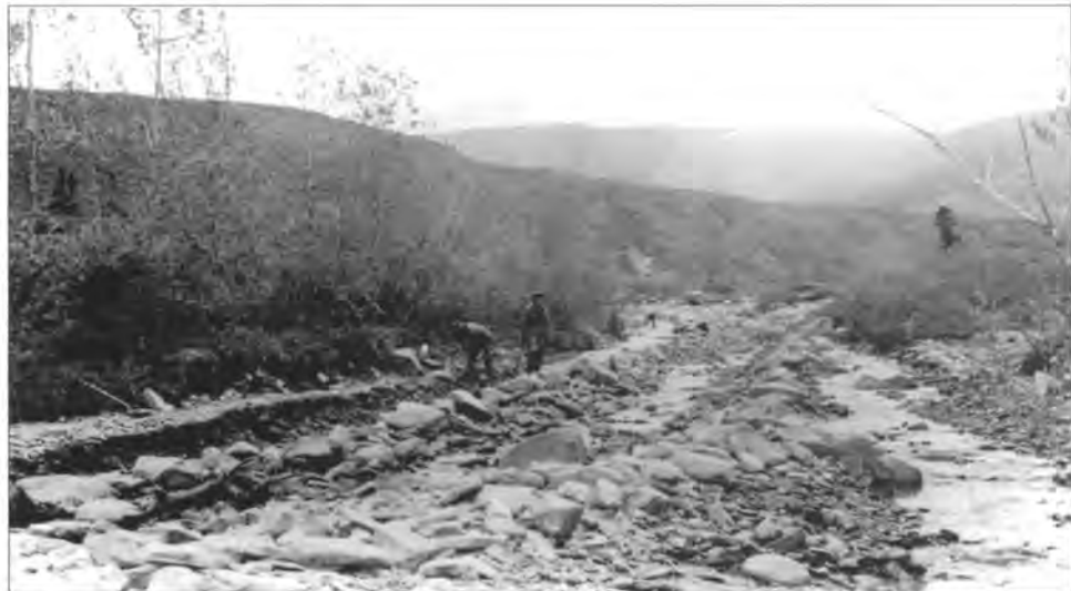
The Glen Creek drainage, first prospected during the 1905-06 gold rush, had mining activity on it until 1985. The photographer, Stephen Foster, described the scene in the above photo as "ground sluicing on Glen Creek" in 1919. Stephen Foster Collection, 69-92-596, University of Alaska Fairbanks Archive
