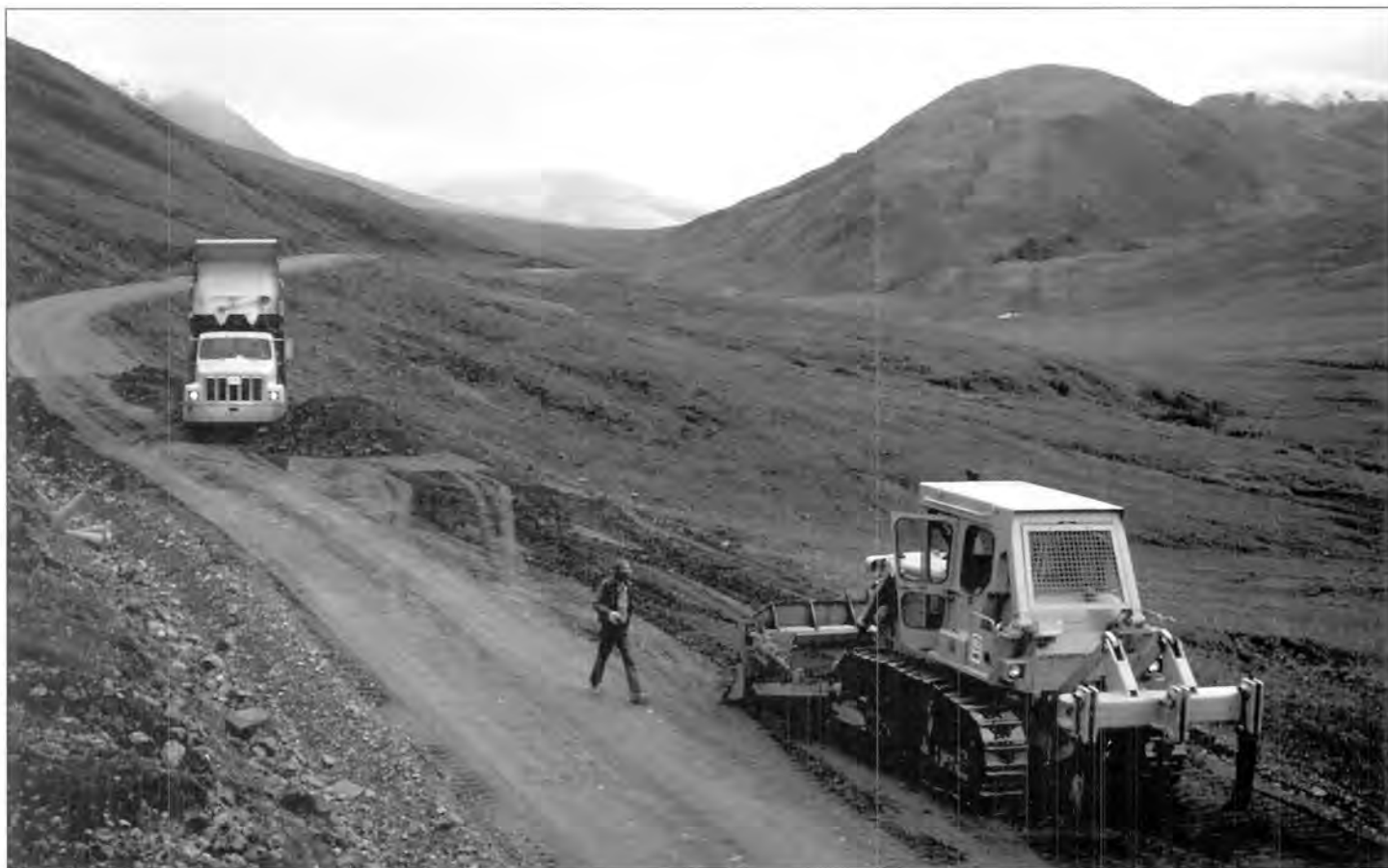
The park road maintenance crew began widening Thorofare Pass in 1984. Brad Ebel Collection
