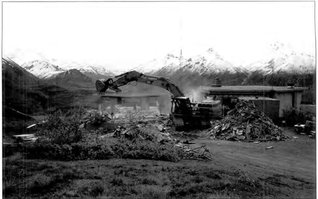
Eielson Visitor Center was demolished during the late summer of 2005. NPS Photo
