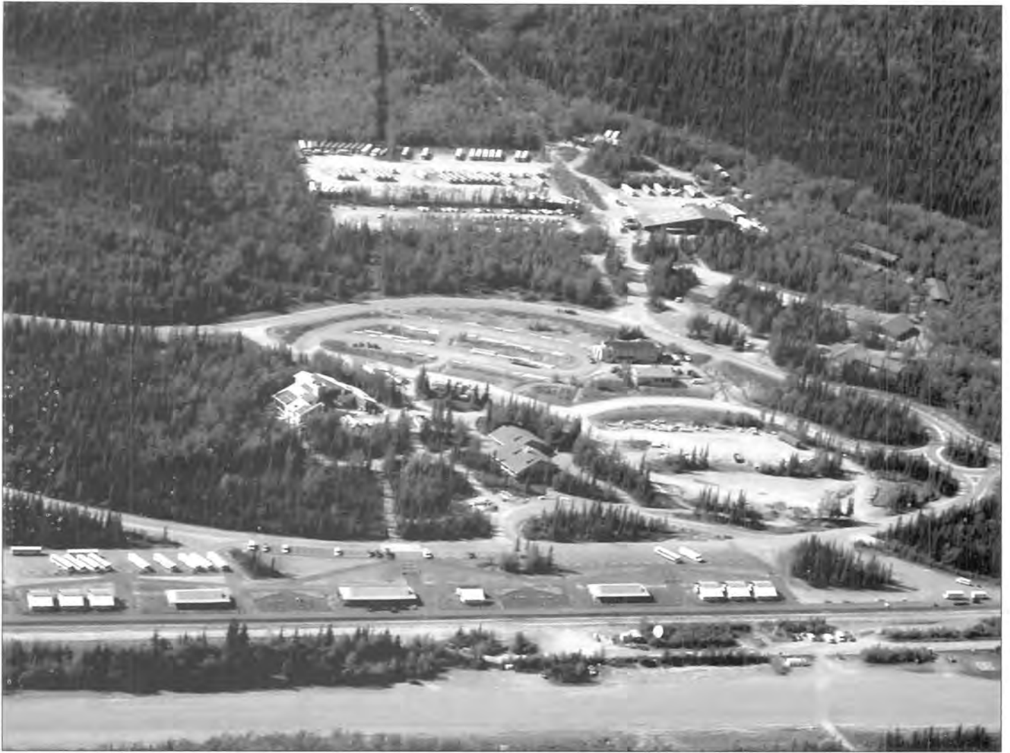
Shown center, in this fall 2004 photo, is the large new parking lot on the former McKinley Park Hotel site, with the hotel powerhouse and dormitory to the right. The Denali Visitor Center is left of center, still under construction. Note the rerouting of the park road from the roundabout on the far right and going to the north of the new parking lot. The old routing of the park road provides access to the depot and terminates there. Fire Management Collection, NPS, Denali National Park and Preserve
