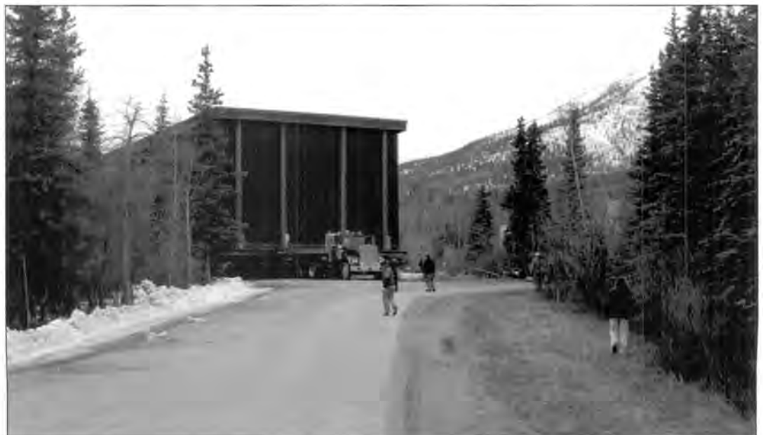
In 2002, the 5,000 square-foot auditorium was moved in one piece from its location behind the park hotel to a site just north of Healy. Clayton Flagg Collection
