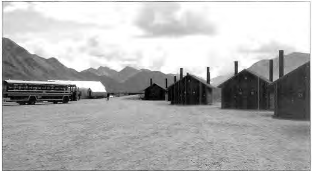
The new Toklat contact station and "SSTs" (Sweet Smelling Toilets) comprised the main rest area for bus passengers during the Eielson Visitor Center demolition and new construction of 2005-2007. NPS Photo
