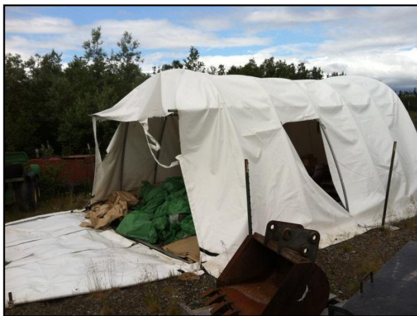
Figure 26. The weather port that stored plant material from past years is ripped apart.
