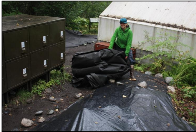
Figure 19. NPS biological technician Jamie Welfelt helps install the final layer of geotextile on the shade covers at Sheep Camp.
