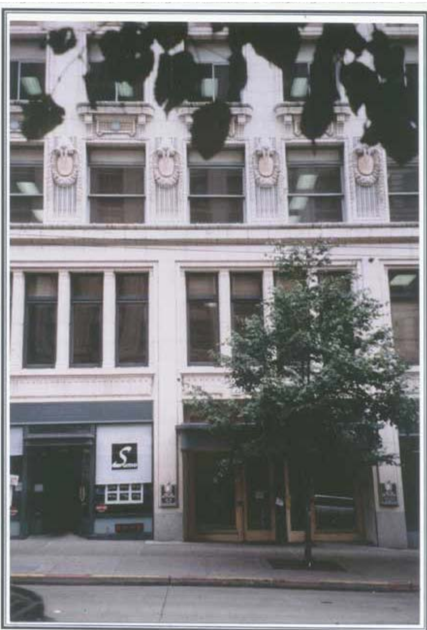
Twenty-seven walruses ring the third-floor exterior of the Arctic Building. (HRA photo)
