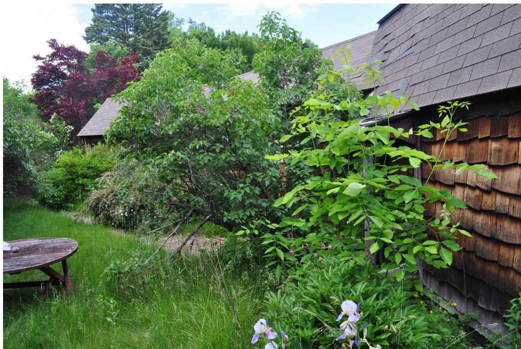
Figure 15. View northwest toward the front of the Beatteay House. The ornamental vegetation is growing unmaintained. (OCLP 2012)
