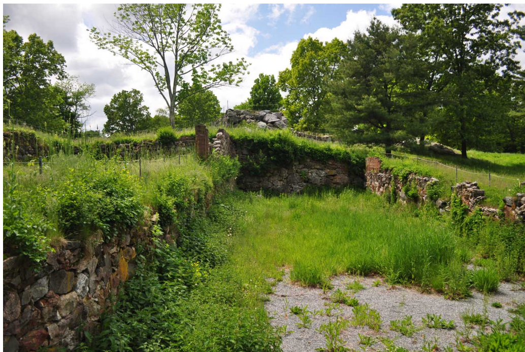
Figure 22. View west toward the large Charles Sawyer Barn Foundation. (OCLP 2012)
