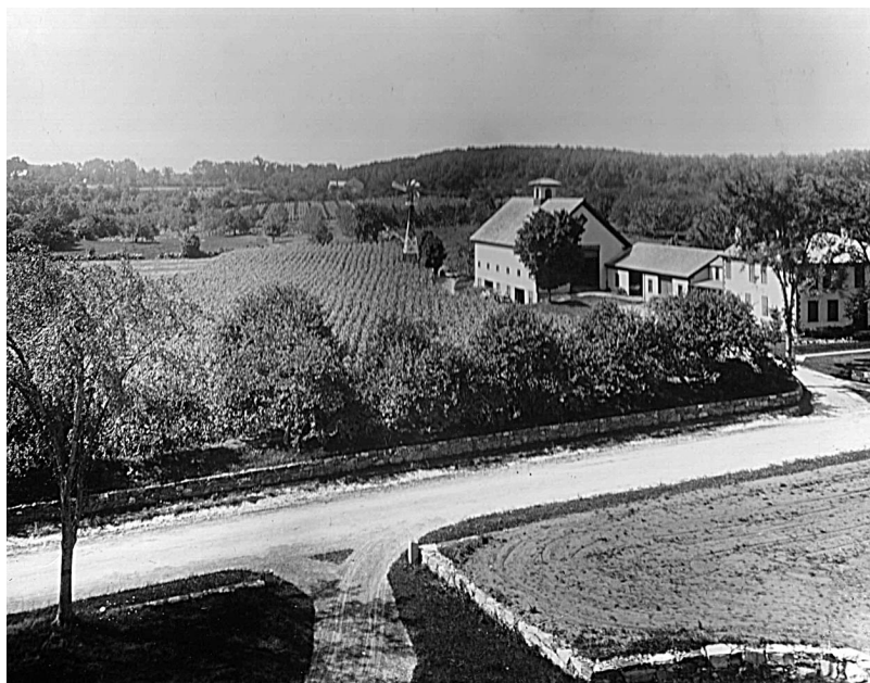
Figure 6. View south toward the Noah Brooks Tavern property, circa 1883-1907, when owned by Samuel Hartwell. (MIMA Library, copy of original photograph located at the Concord Free Public Library in the Alfred W. Hosmer Collection)
