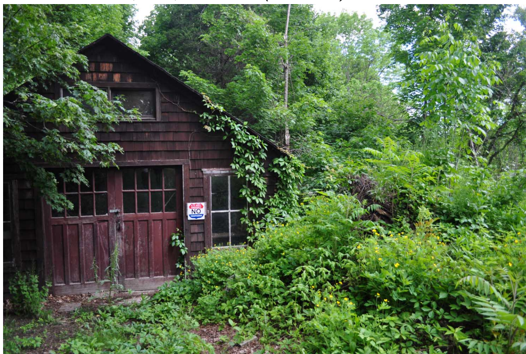
Figure 25. View north toward the Walter Beatteay garage obscured by vegetation. (OCLP 2012)
