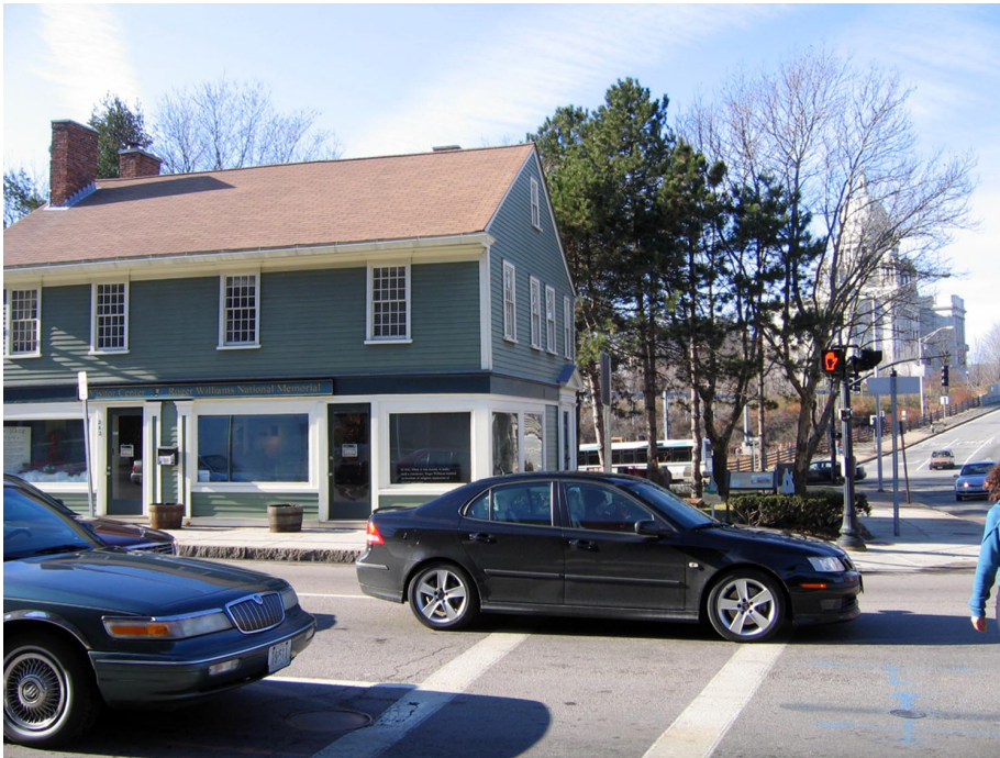
Figure 26. The Antram-Gray House, location of the visitor center and park offices, looking southwest across North Main Street with the state capitol in the background, 2008. (SUNY ESF)
