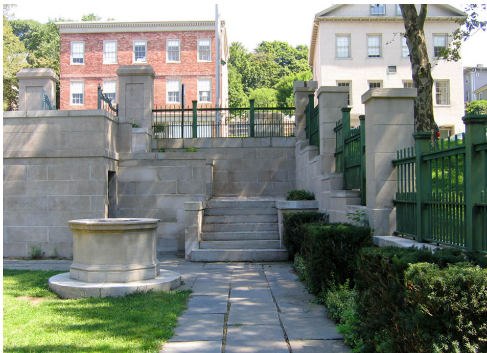
Figure 19. The steps of the main stairway looking east along the south side of the courtyard, 2008. This photograph also shows the bluestone walks, octagonal wellcurb, and the doorway into the utility room within the stairway structure. (SUNY ESF)
