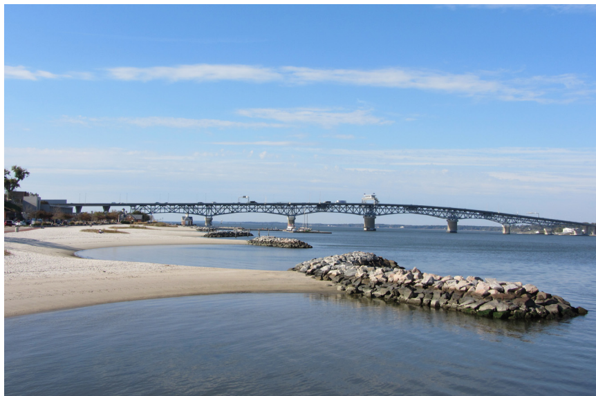
Figure 13. Rock breakwaters at Yorktown Beach along the York River (#116–118 Figure 12). Coleman Bridge in the background carries U.S. Highway 17. View is to the northwest.
