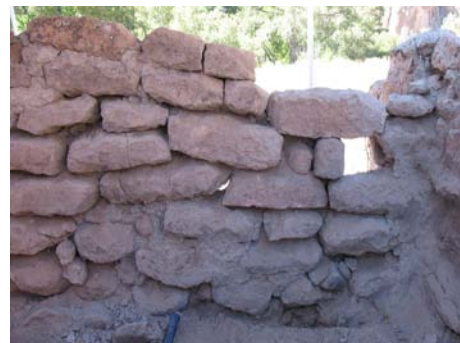
19 B NW I, after cleaning out joints and exposing the stones
