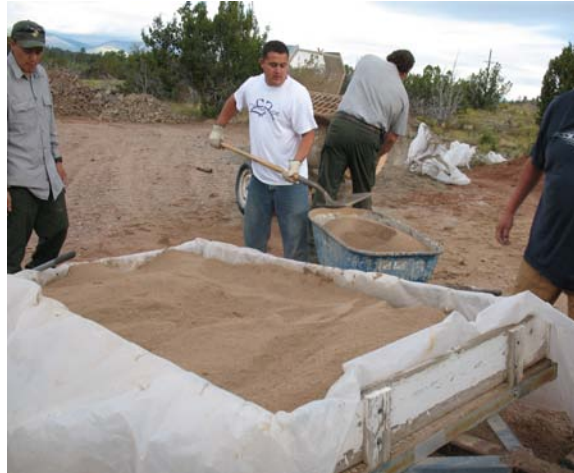
Figure 6: Loading up the trailer at the gravel yard
