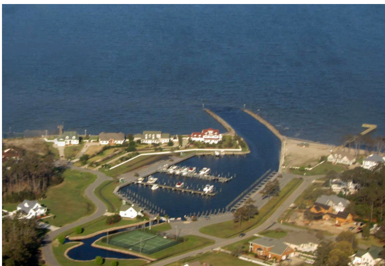
Figure 11. Heritage Point residential area and marina. View is to the northwest (image by Kate Dallas).
