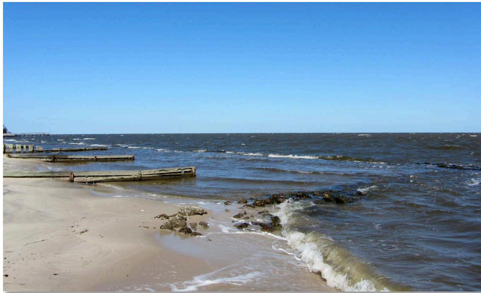
Figure 8. Wooden groins (#74–77 Figure 5) and submerged breakwater (#66 Figure 5) to the east of the theater. View is to the northwest (image by Kate Dallas).
