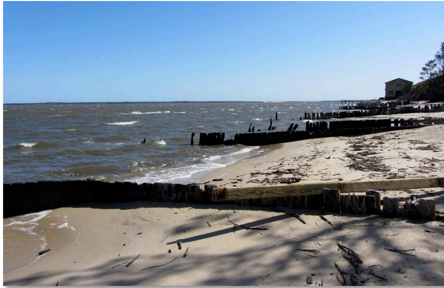
Figure 7. Wooden groins to the west of the Waterside Theater (#60–63 Figure 5). View is to the east (image by Kate Dallas).
