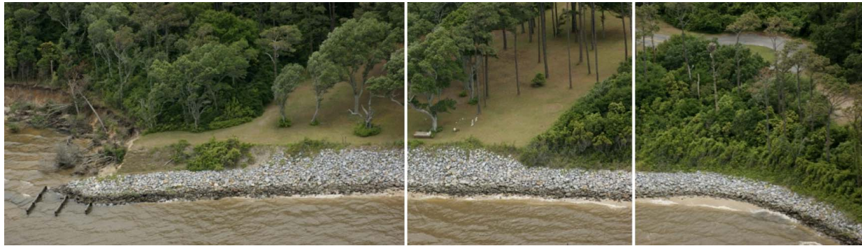
Figure 15. Rock revetment and groins in front of the Dough Cemetery (#42 Figure 5). View is to the south (images from Eshleman and York 2011).
