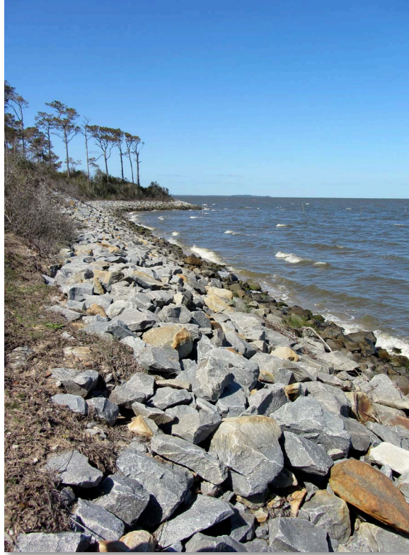
Figure 9. Revetment fronting the Dough Cemetery (#42 Figure 5). View is to the west (image by Kate Dallas).
