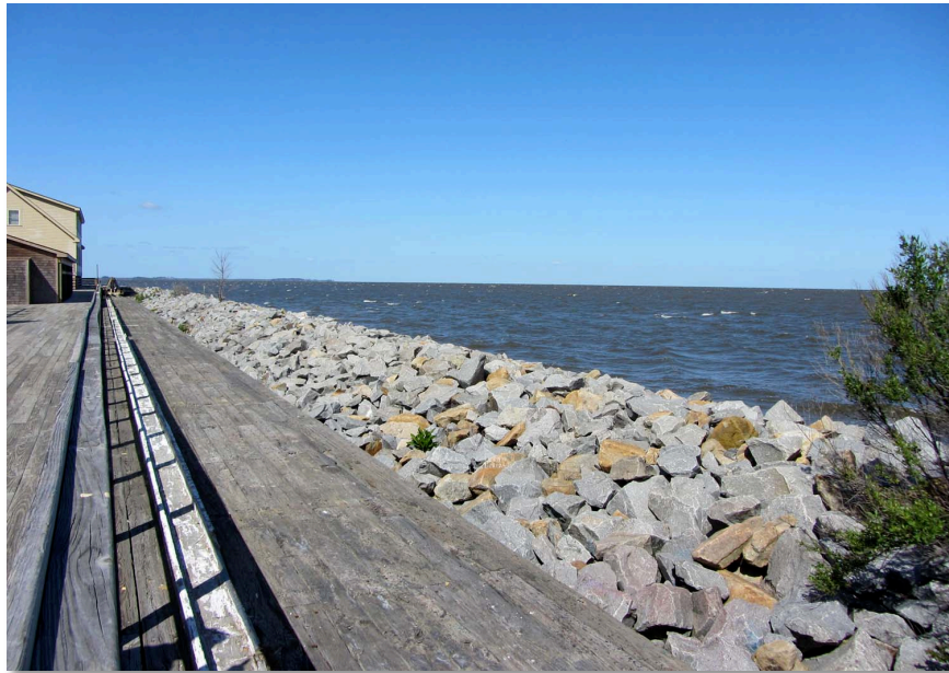
Figure 6. Revetment (#64 Figure 5) fronting the Waterside Theater. View is to the west (image by Kate Dallas).
