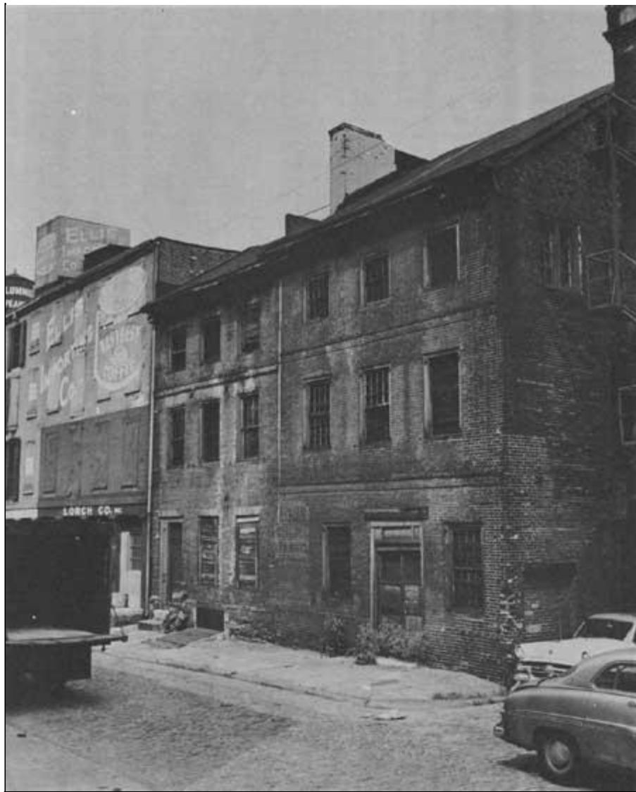
Illustration No. 3. "IRON RAIL FROM CHIMNEY TO CHIMNEY," on house at 115 North Water Street is shown in this photograph taken a few years before its demolition. Note such other characteristics of building's period as molded brick above second story windows. Independence National Historical Park photographic file.
