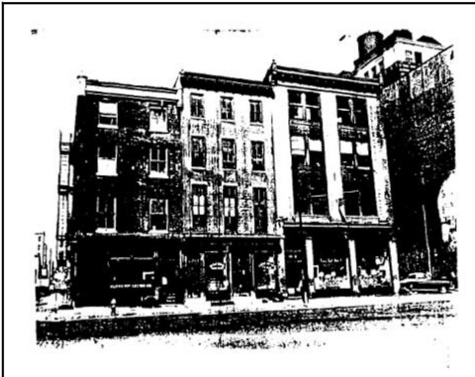
6. Fifth Street between Cherry Street and Quarry facing West. Photo By Kehoe July 1953 (INDE 1028) ( click on image for an enlargement in a new window )
