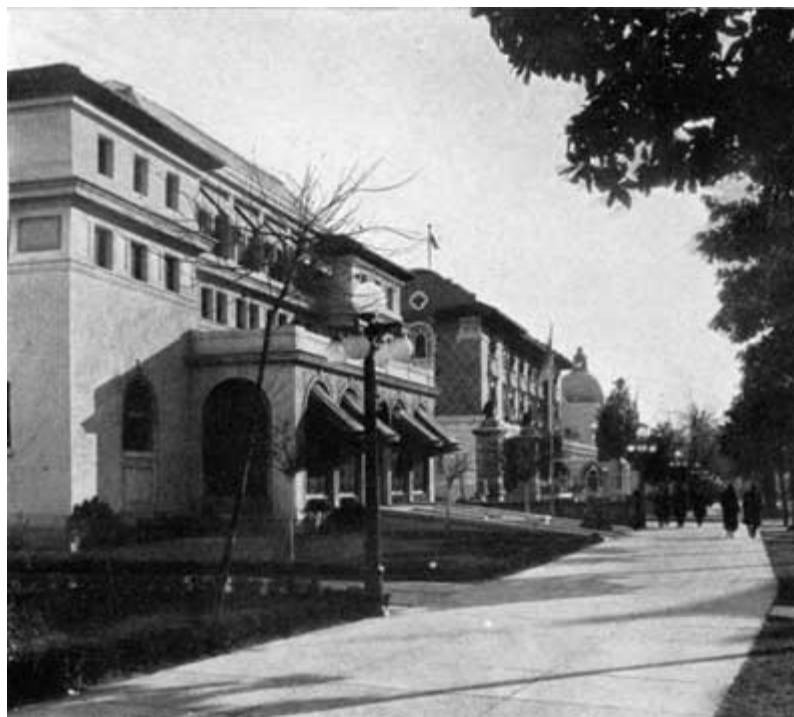
Bathhouse Row—Hot Springs National Park
