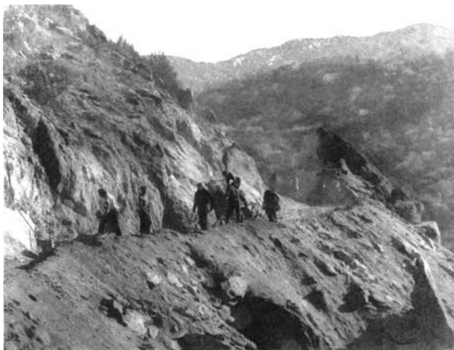
CCC men cutting a truck trail through granite ridge—Sequoia National Park
