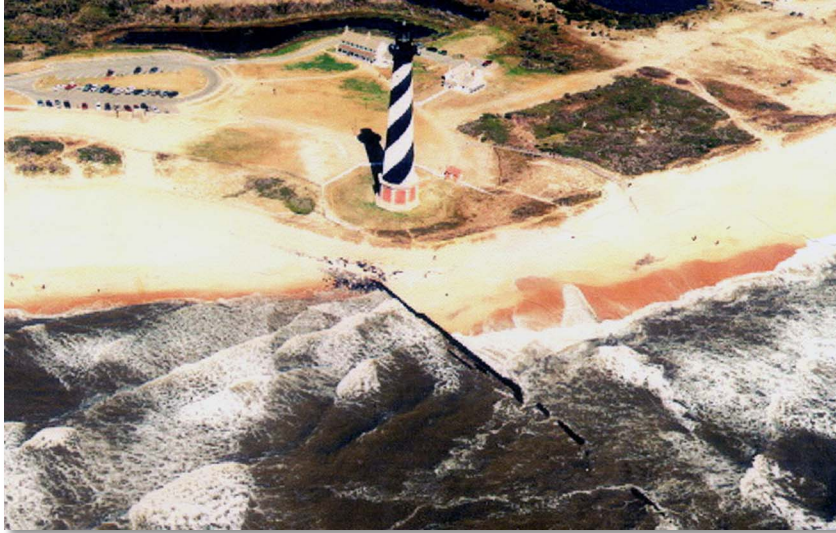
Figure 32. Photograph shows the proximity of the lighthouse to the ocean prior to relocation (circa 1990). Note the impoundment of sediment along the north (right) side of the groin. View is to the west (NPS photo).
