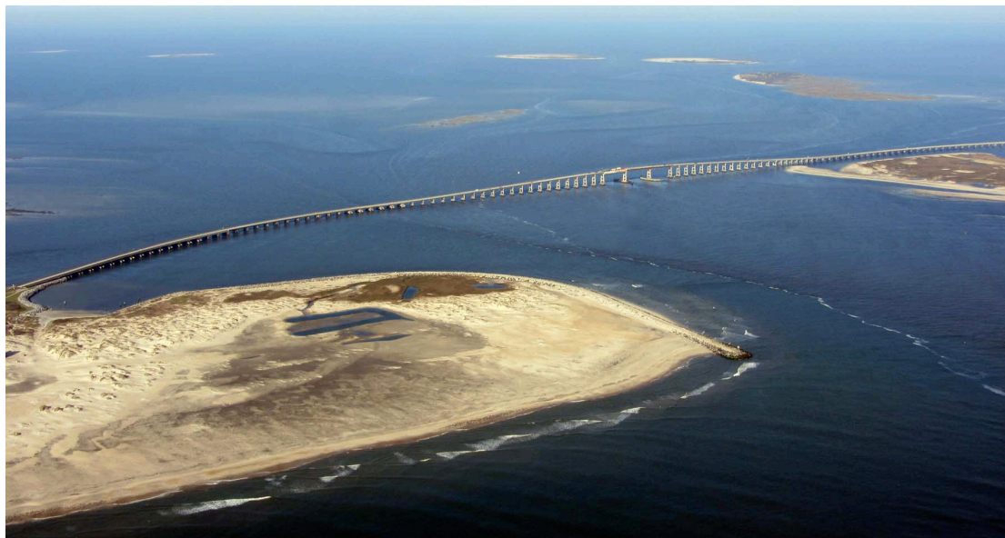
Figure 10. The Herbert Bonner Bridge across Oregon Inlet and the northern end of Pea Island. The terminal groin is visible in the middle of the image. View is to the northwest (image by Kate Dallas).
