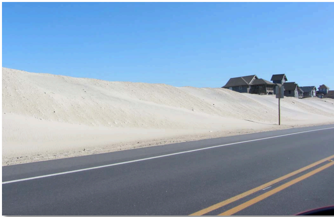
Figure 5. Constructed dunes (seen here north of Rodanthe in March 2012) parallel Highway 12 nearly the entire length of CAHA (image by Kate Dallas).
