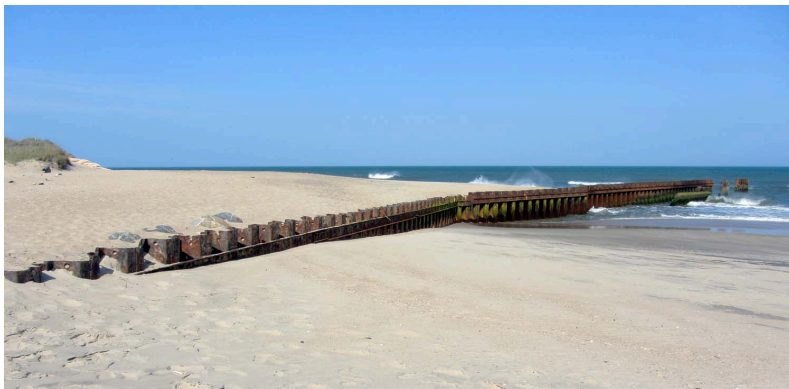
Figure 16. Steel sheet-pile groin (that was built in 1969 to protect a Navy facility) at the former location of the Cape Hatteras Lighthouse (#31 Figure 14). View is to the northeast (image by Kate Dallas).
