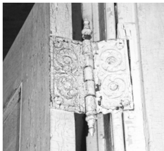
Figure 48 View of "fancy" hinges originally used at most primary doors. NPS SERO 2001.
