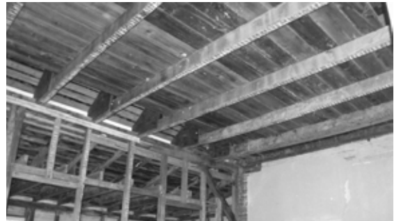
Figure 41 View of typical first floor ceiling framing. NPS SERO 2001.
