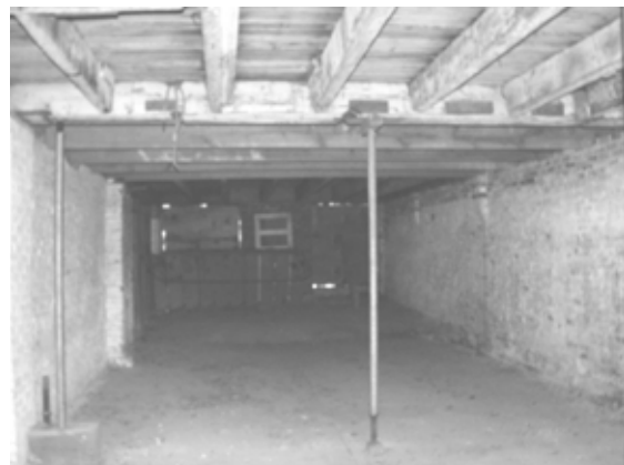
Figure 63 View east in Room 001. NPS SERO 2001.
