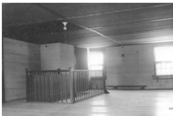
Figure 18 View north in Room 200, May 1965, showing fiber board ceiling installed by Major Holt in 1931. VICK Coll.
