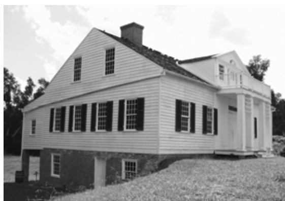
Figure 33 View of house from southwest. NPS SERO 2001
