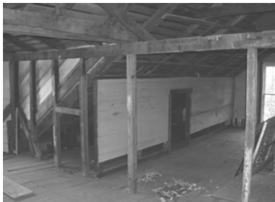
Figure 68 View southwest in Room 200. NPS SERO 2001.
