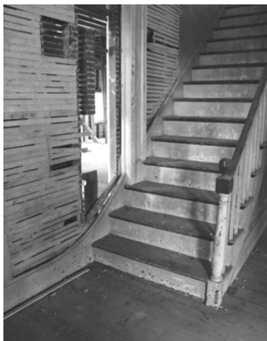
Figure 52 View of main staircase. NPS SERO 2001
