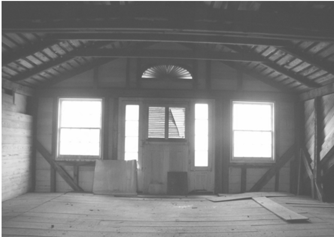
Figure 67 View south in Room 200. NPS SERO 2001.
