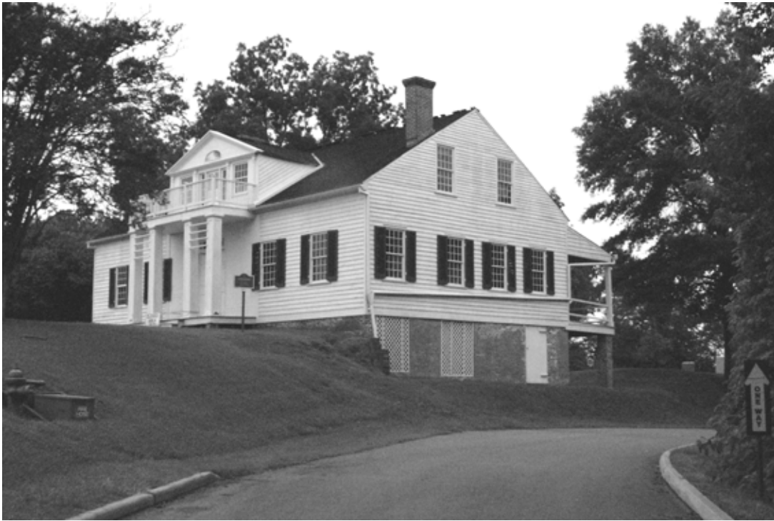
Figure 37 View northwest along Union Avenue. NPS SERO 2001.
