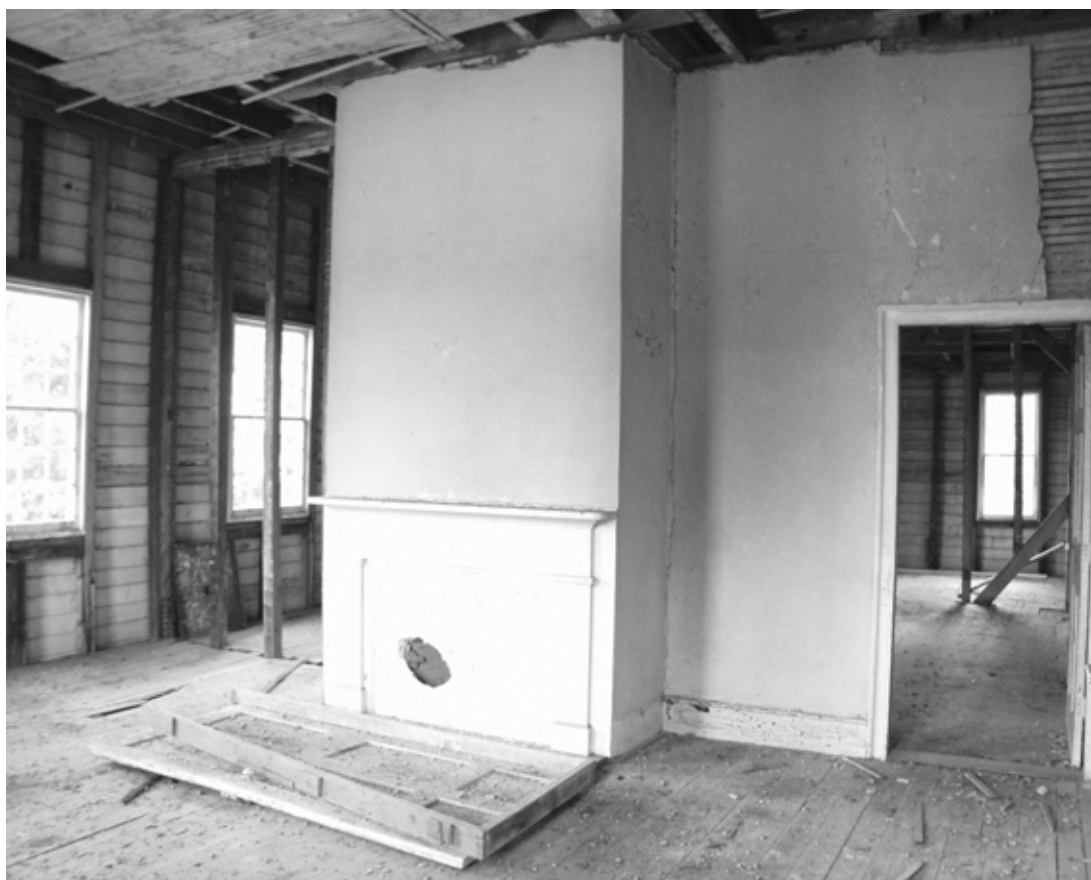
Figure 54 View to northwest in Room 101. NPS SERO 2001.
