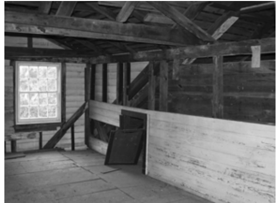
Figure 69 View to northeast in Room 200. NPS SERO 2001.
