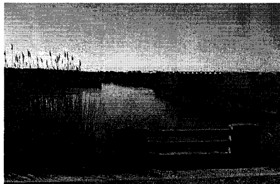
Figure 4 View from High Head Road looking toward Rte 6 culvert.
