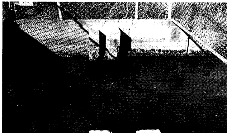
Figure 6 Weir gate guides located inside metal fence cage on Pilgrim Lake end of High Head Road culvert - flume system.
