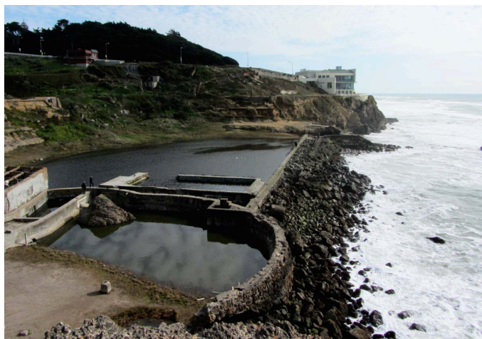
Figure 25. Sutro Baths' ruins with its concrete and rock seawall and revetment (#77–78 Figure 24). View is to the south (image by Kate Dallas).
