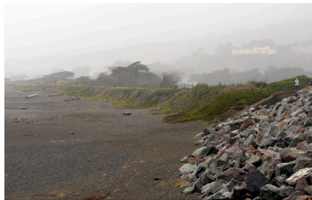
Figure 32. Levee and revetment at Mori Point/Sharp Park (#93–94 Figure 31). View is to the northeast (image by Kate Dallas).
