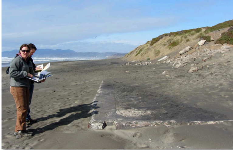
Figure 27. Jodi Eshleman and Mike Berry at the buried Taraval Seawall (#82 Figure 24). Concrete rubble is also visible on the dune face. View is to the north (image by Kate Dallas).
