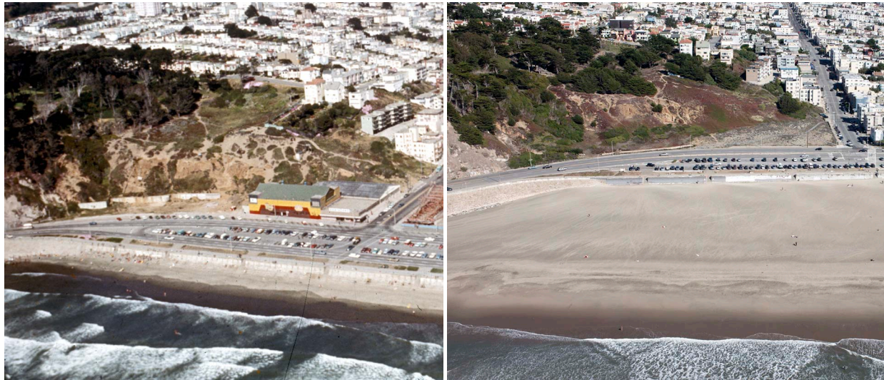
Figure 26. Oblique aerial imagery of northern Ocean Beach and the O'Shaughnessey Seawall (#79 Figure 24) in 1972 (left) and 2009 (right) illustrates the significant progradation that has occurred on the northern section of the beach (from Adelman and Adelman 2012).
