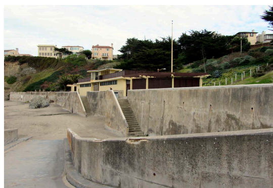
Figure 23. China Beach seawall (#76 Figure 24) (image by Kate Dallas).
