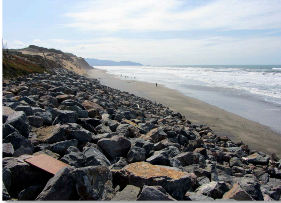
Figure 28. Revetment at southern Ocean Beach installed in 2010 (#86 Figure 24). View is to the south towards Fort Funston (image by Kate Dallas).
