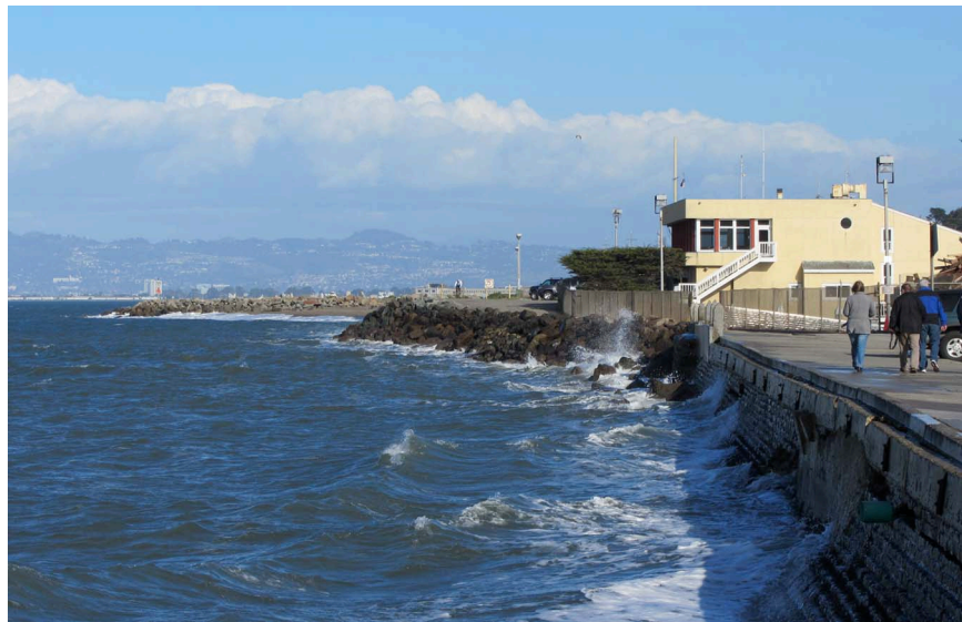
Figure 18. St. Francis Spit seawall and rubble breakwater (#53, 60 Figure 17). View is to the east (image by Kate Dallas).
