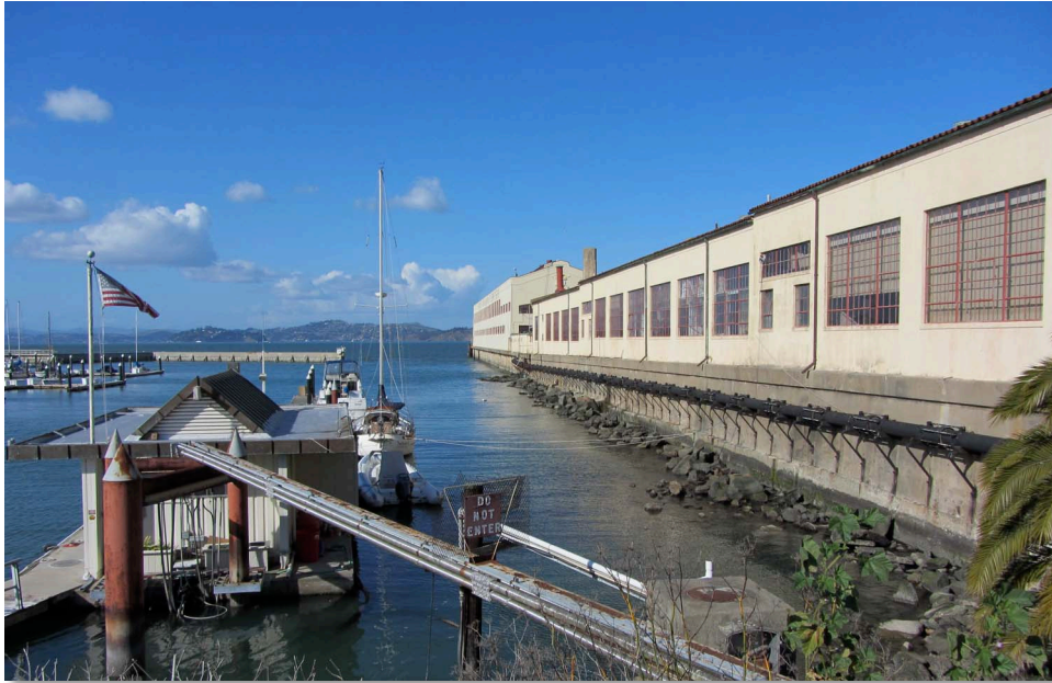
Figure 14. Fort Mason's Pier 1, seawall, and revetment (#29, 32, 33 Figure 13). Piers and a breakwater (middle left) in the San Francisco Marina's East Harbor are also visible (#35, 40, 41 Figure 13). View is to the north (image by Kate Dallas).
