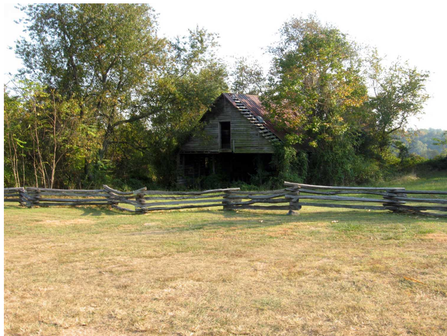
Figure 21. The abandoned c.1934 granary looking southeast across the visitor parking area, October 2007 (SUNY ESF).
