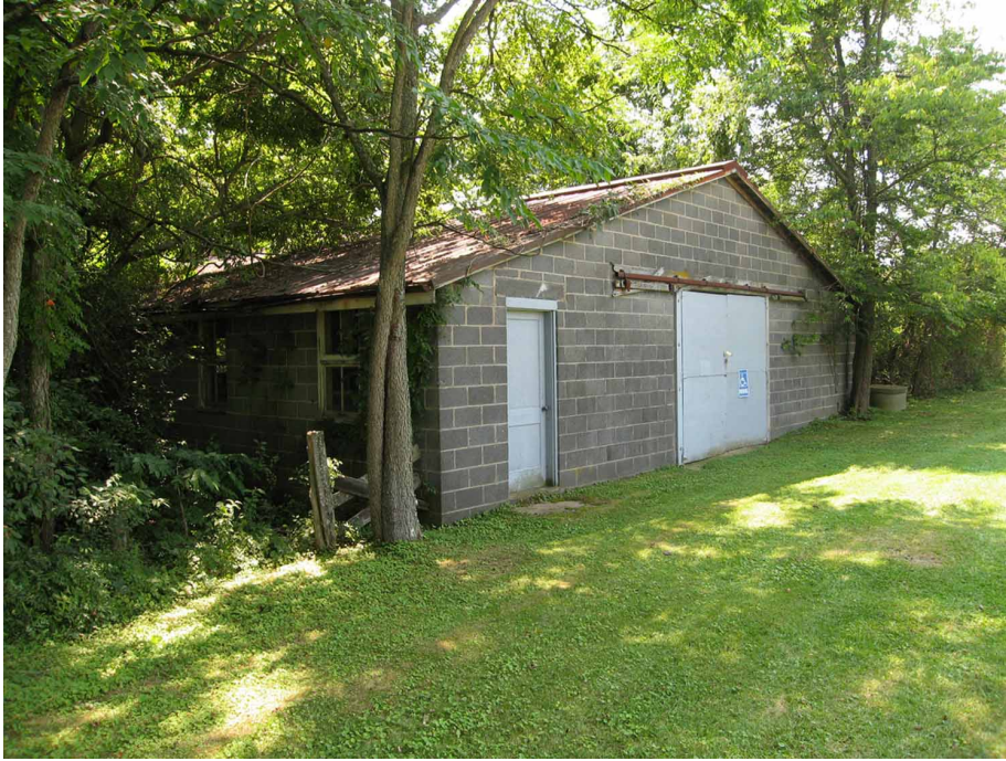
Figure 28. The c.1950 brooder house, presently used for storage, looking southwest, August 2007. Visible at the left of the building is a remnant of a plank fence that enclosed adjoining corrals. The vegetation has grown since the late 1960s (SUNY ESF).
