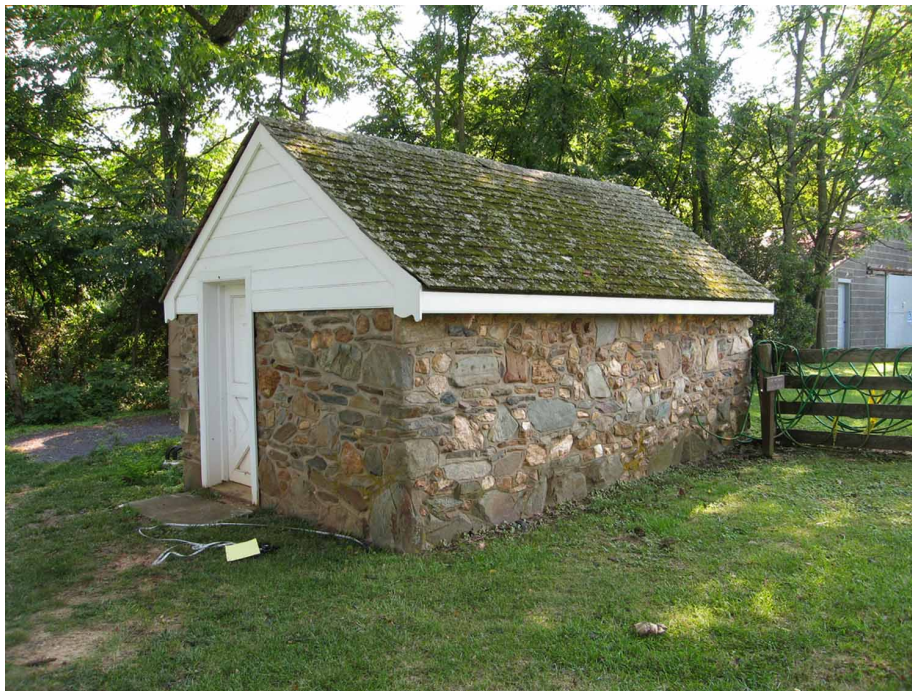
Figure 27. The 1934 farm office at the western edge of the house grounds looking southwest with the brooder house in the background, August 2007. The entrance is from the house grounds (SUNY ESF).
