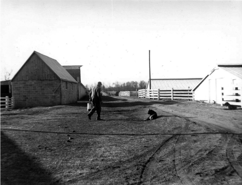
Figure 15. Looking west through the barnyard along the entrance road showing plank fences and buildings constructed after World War II, photographed c.1955 (Collection of Carolyn Elstner).
