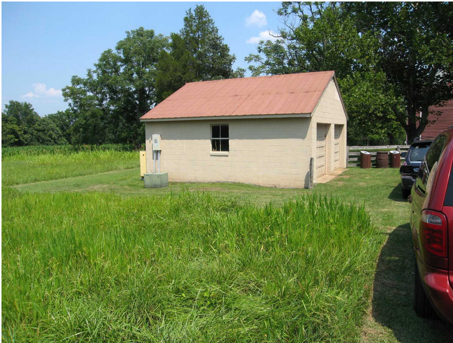
Figure 29. The c.1960 garage looking northeast from the entrance road, August 2007. This building serves as a maintenance facility (SUNY ESF).
