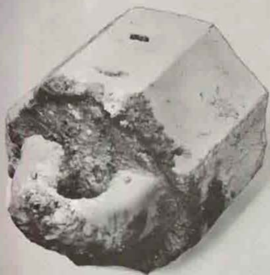
THIS 1,300-POUND IRON PILEDRIVER USED FOR DRIVING PILES IN THE BUILDING OF SMALL WHARVES WAS FOUND AT JAMESTOWN.
