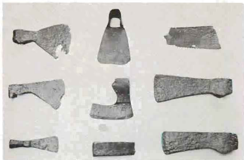
A FEW OF MANY TOOLS UNEARTHED AT JAMESTOWN WHICH WERE USED FOR TIMBERING: FELLING AXES, A HEWING AXE, ADZE, HATCHET, WEDGE, AND SAW FRAGMENT.
