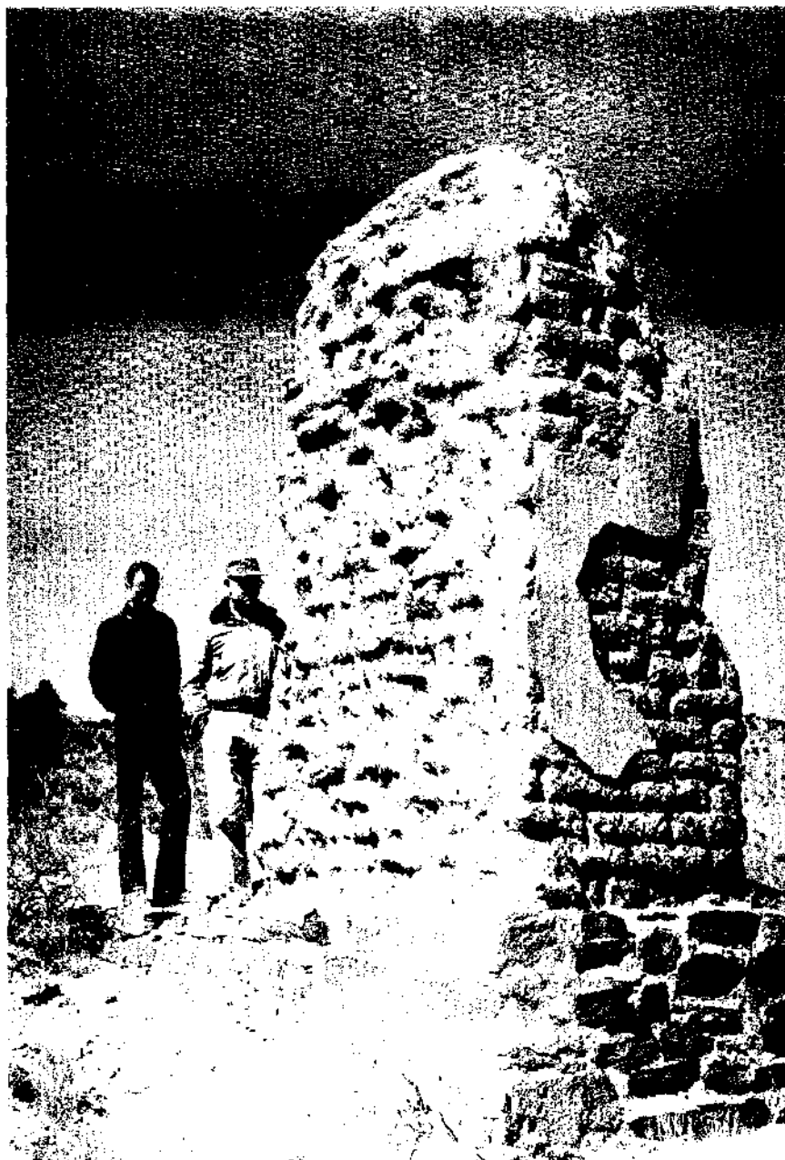
Photo No. 7 - Standing wall of the Hospital Stewards Quarters showing typical construction. Stone foundation, adobe walls and exterior plaster. McCollm and Benson in photo. Arnberger, 1957.
